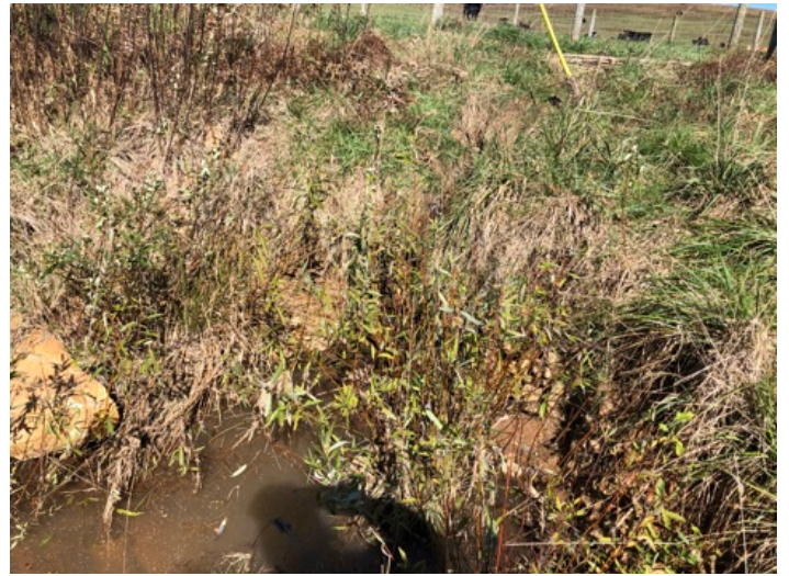
Photo 14 – UT2 BMP: Headcut at intake. 11-6-2020
