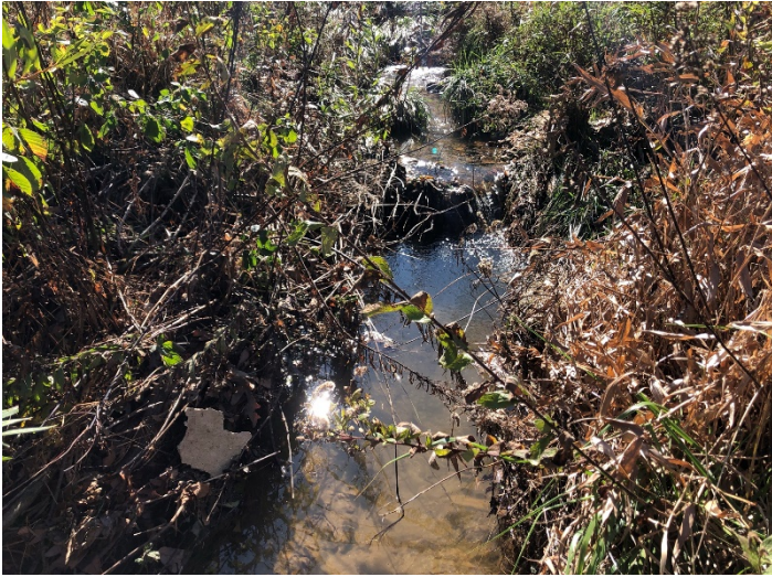
Photo 7 – UT1 R1: Station 205+10-205+50- Stream realignment. 11-6-2020
