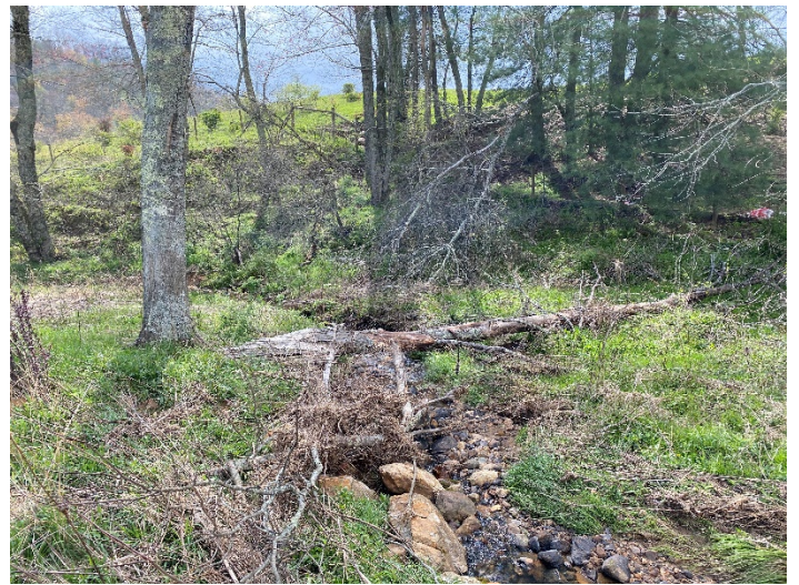
Photo Point 33 – view downstream UT2 (4/13/2020)
