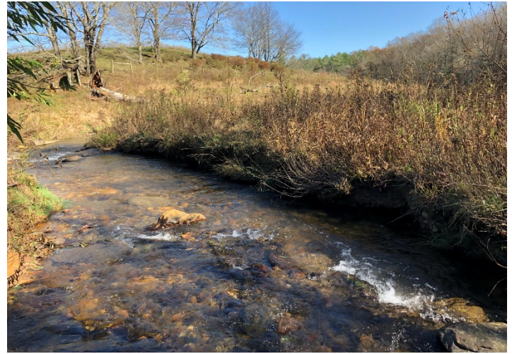
Photo 4 – Vile Creek R2: Station 120+70-121+00 – Bank scour. 11-6-2020
