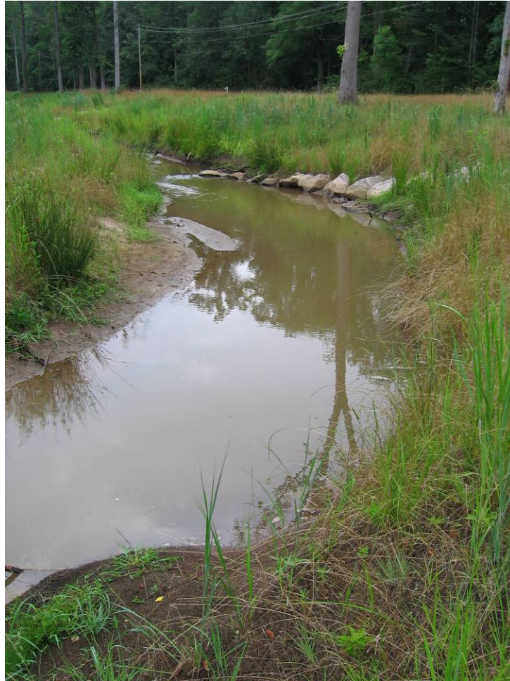
Photo 66: Problem Area X, 25+00 (0914 – Looking upstream) 06/22/05
