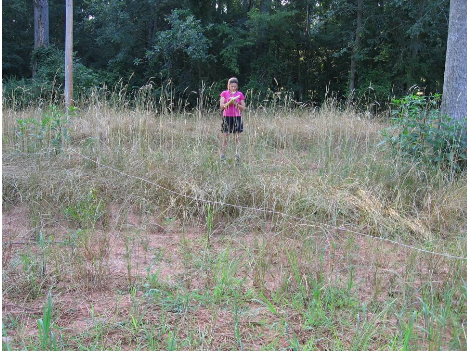
Photo 13: Vegetative Problem Area i, 22+50 – 23+80 (0819 – Left Bank) 06/22/05
