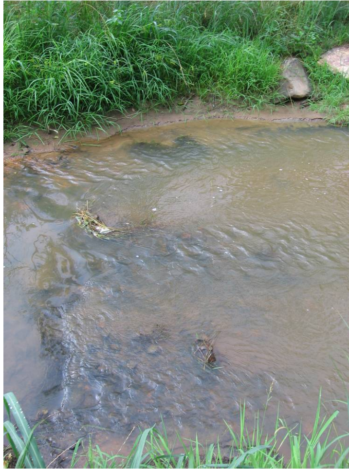
Photo 70: Problem Area XI, 26+70 (0921 – From Right Bank) 06/22/05
