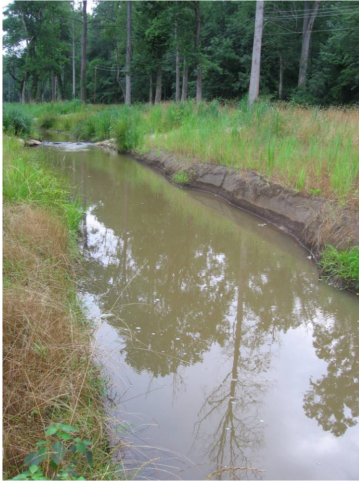
Photo 62: Problem Area IX, 23+10 (0904 – Looking upstream) 06/22/05
