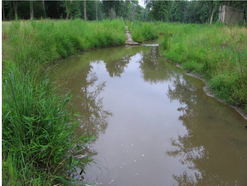
Photo 57: Problem Area V, 13+80 (0893 - Looking downstream) 06/22/05
