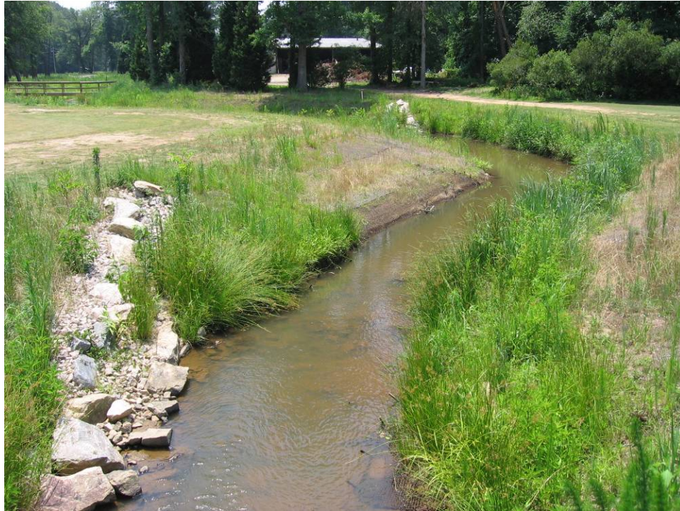
Photo 5: Vegetative Problem Area c, 4+00 – 4+50 (0788 – Left Bank) 06/22/05
