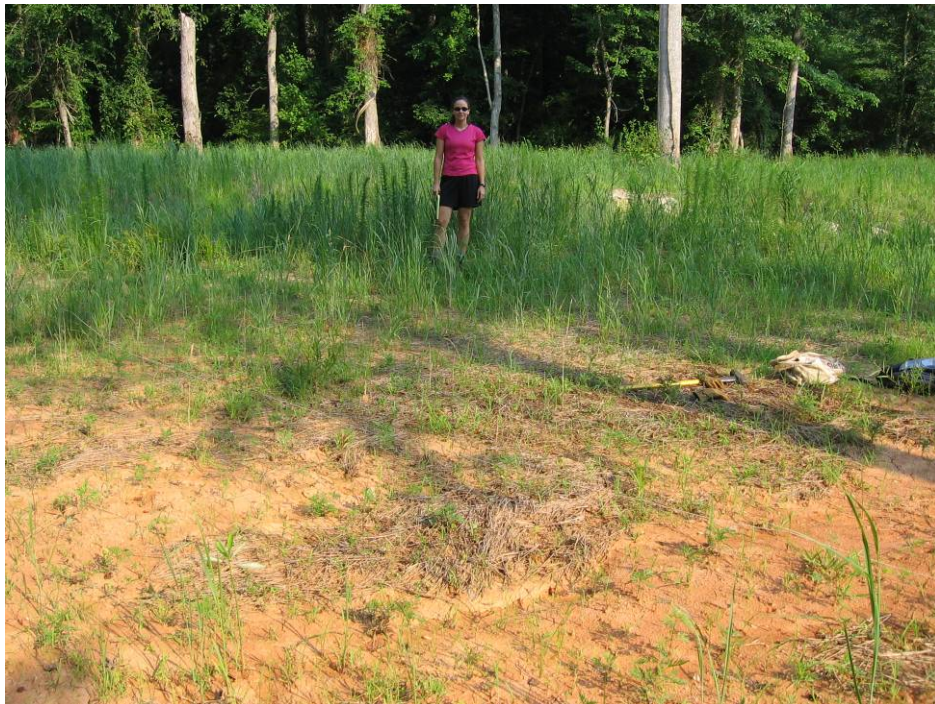
Photo 14: Vegetative Problem Area j, 25+50 – 26+50 (0822 – Left Bank) 06/22/05
