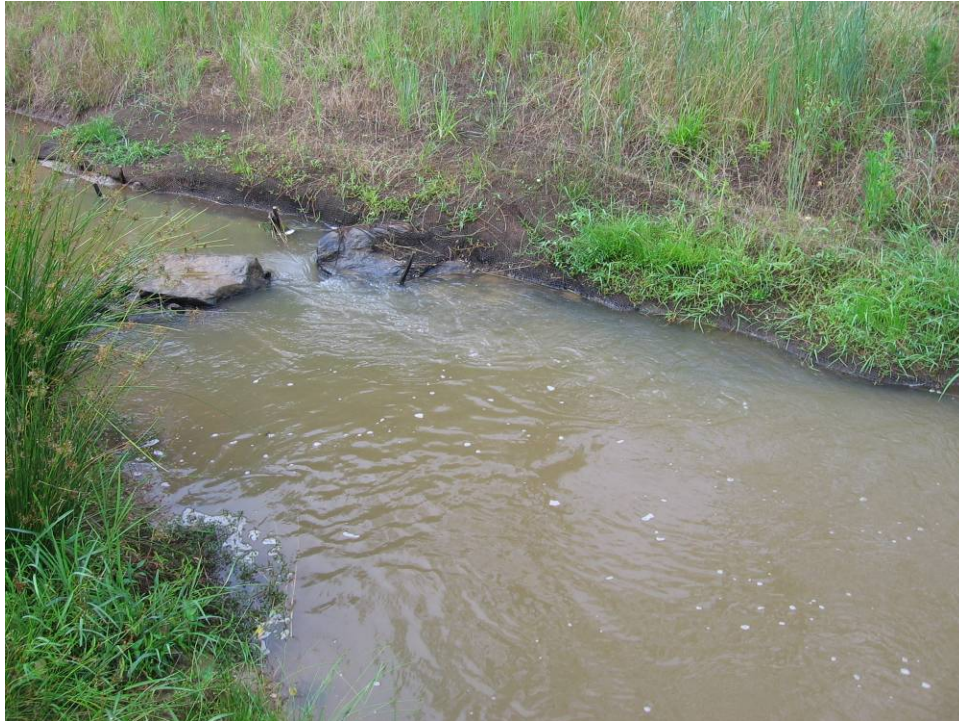
Photo 68: Problem Area X, 25+00 (0919 – Looking upstream) 06/22/05
