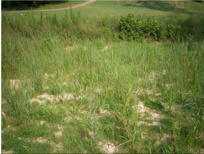
VPA 5: Vegetative Problem Area "c" 4+00 – 4+50
