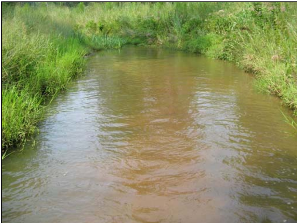
Photograph SPA-4: Channel Over-widening, 22+00, 8.01.06
