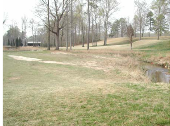
Photo 2. Representative bare floodplain problem area (approximately Station 13+00). Note the sandy deposits on the floodplain indicating a recent over-bankfull flow. Photo was taken on 3/28/2007.
