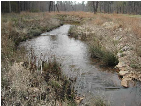
Photo 7: Representative over-widening of the channel (26+19 along mainstem).
