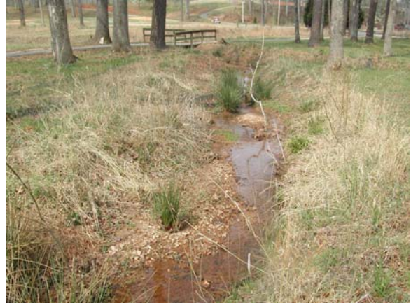
Photo 8: Representative aggradation problem area (14+17 along unnamed tributary).
