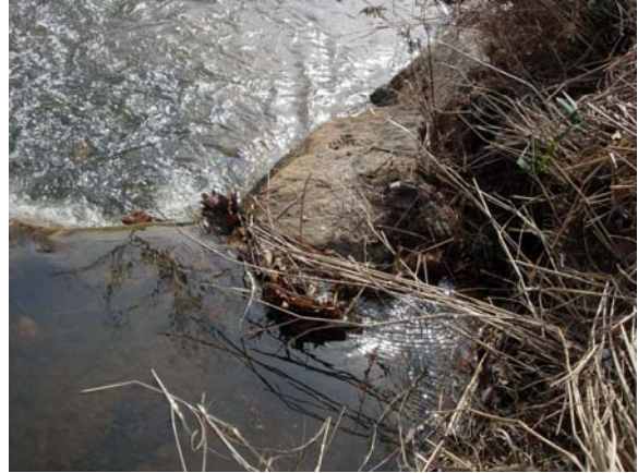
Photo 4: Representative cross-vane problem area, Horse Creek (Station 34+91 view downstream of piping on right arm; 2-15-2008).
