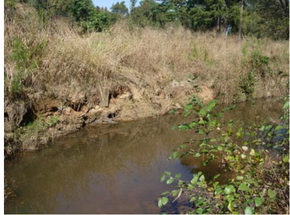
Photo 2: Representative severe bank erosion problem area (Station 29+65; view upstream of right bank along Horse Creek; 10-15-2008).
