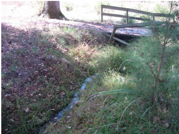
Photo-Point 12: View downstream. UT Horse Creek (10-16-2008).
