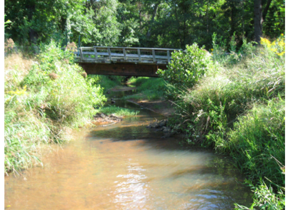
Cross-Section 1: View upstream. Horse Creek (8-19-2009).
