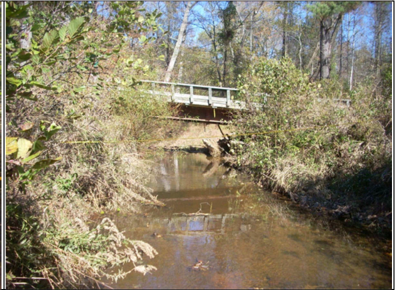
Cross-Section 1: View upstream. Horse Creek (11-10-2010)
