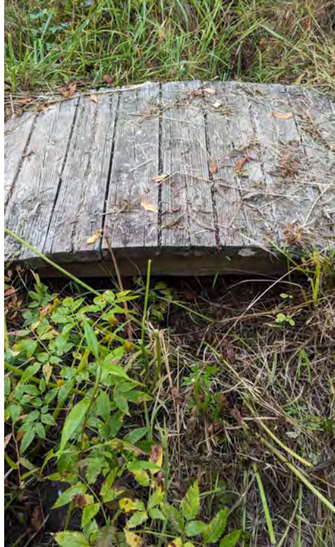
Permanent Photo Point 19: Footbridge crossing on UT 8 downstream end, facing upstream (Taken 9/27/23)
