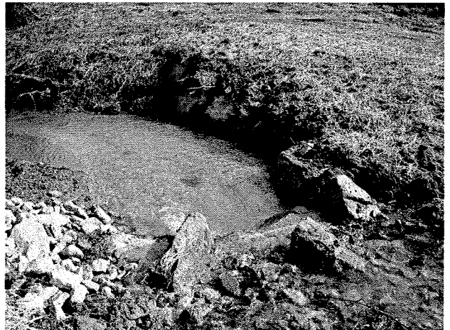
Photograph 52. Rock J vane installed at MC Station 21+63. (1/16/04)
