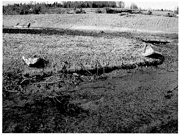
Photograph 56. Log toe protection installed on left bank between MC Stations 23+50 and 23+70. (1/16/04)
