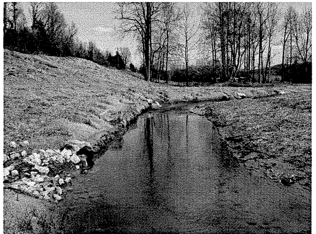
Photograph 24. Looking downstream at log toe protection and MS Station 53+96 rock vane. (4/7/04)
