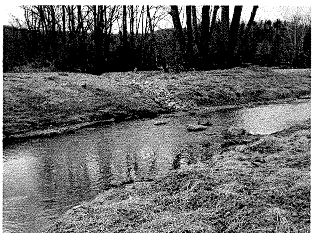
Photograph 120. Looking upstream at rock J vane installed at MS Station 4+72 (existing ditch in background). (4/7/04)
