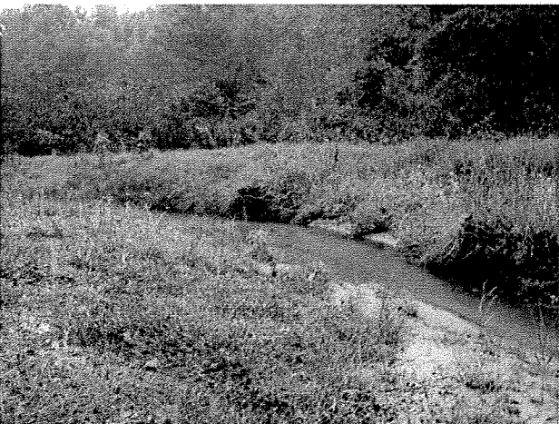
Photograph 23. Looking downstream at root wads installed between MC Stations 10+50 and 11+00. (9/27/04)
