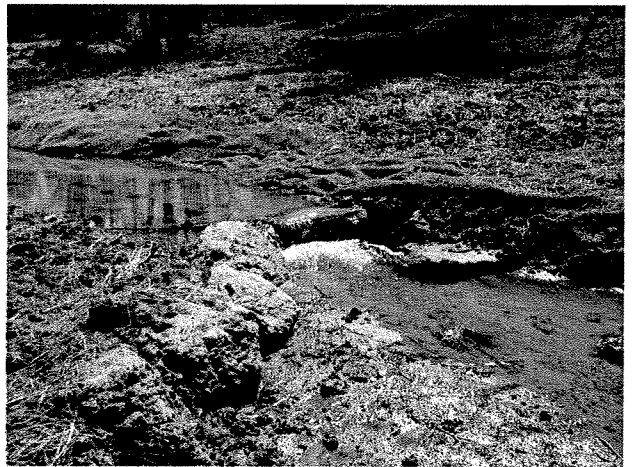
Photograph 22. Cross vane installed at LT Station 5+90. (4/7/04)
