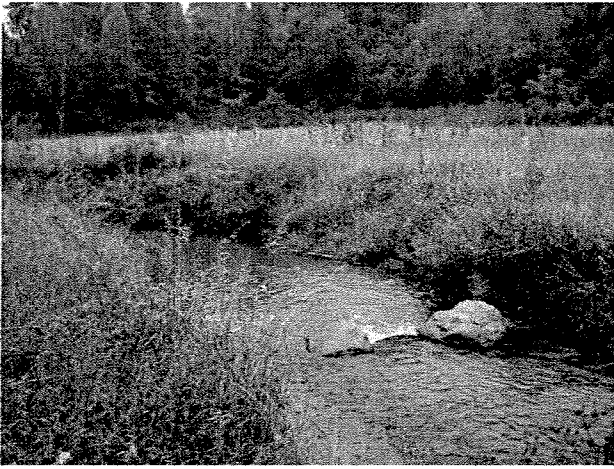
Photograph 67. Looking downstream at rock J vane installed at MS Station 29+10. (9/27/04)
