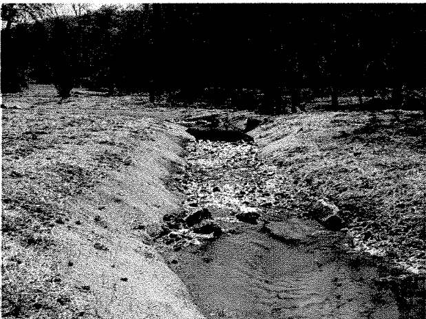
Photograph 17. Rock J vane installed at LT Station 4+33. (4/7/04)
