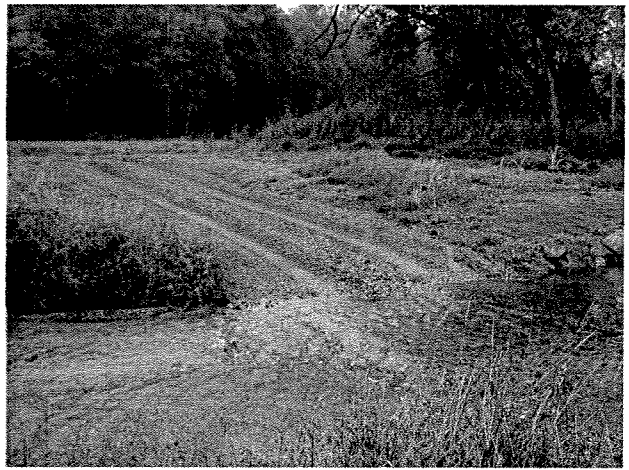
Photograph 86. Ford stream crossing installed at MS Station 18+75. (9/27/04)
