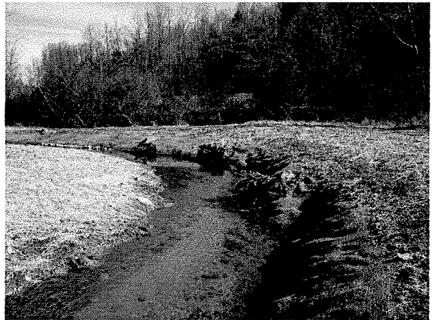
Photograph 22. Looking downstream at root wads installed between MC Stations 10+50 and 11+00. (1/16/04)
