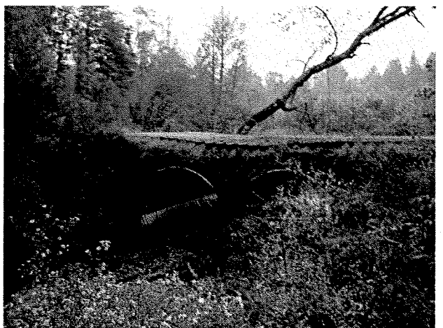
Photograph 6. Downstream face of culvert installed at upstream end of project area. (9/27/04)
