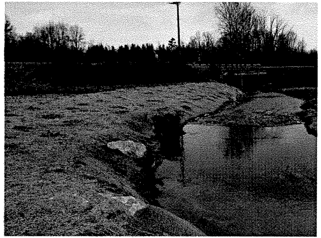
Photograph 128. Looking downstream at root wads installed between MS Stations 3+10 and 2+80. (4/7/04)
