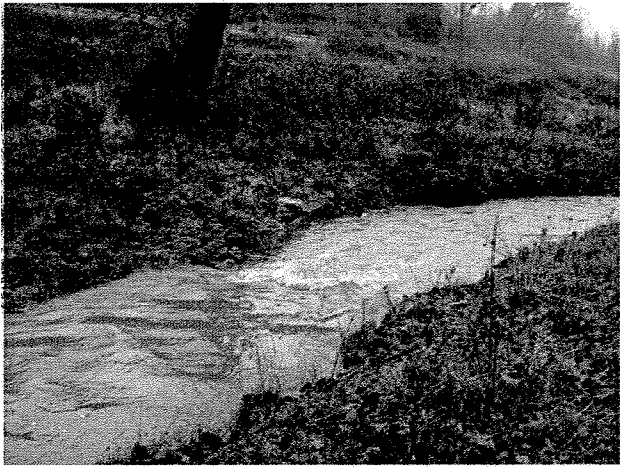
Photograph 21. Rock J vane installed at MS Station 56+19 during storm event. (11/12/04)
