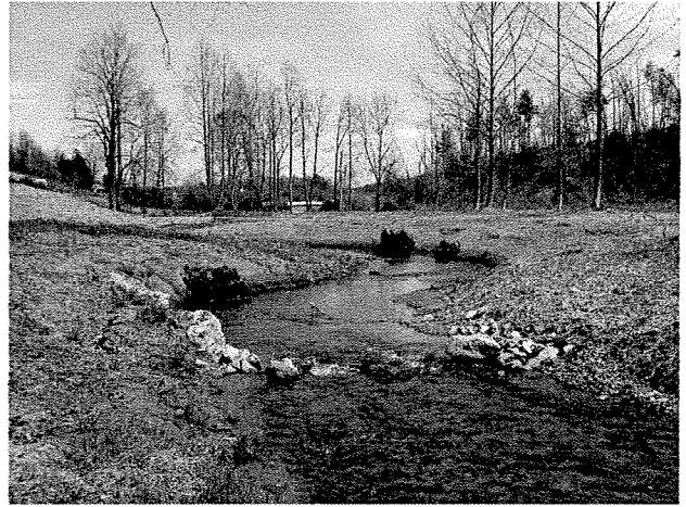
Photograph 20. Rock J vane installed at MS Station 56+19. (4/7/04)
