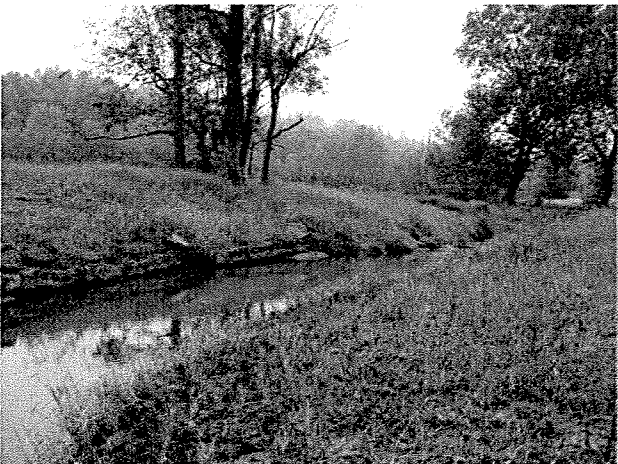
Photograph 113. Looking upstream at log toe protection installed between MS Stations 8+70 and 8+30. (9/27/04)
