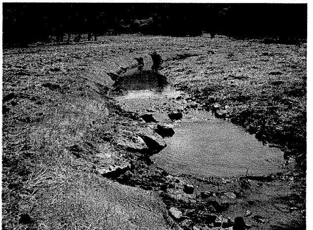
Photograph 30. Looking upstream at rock J vane installed at LT Station 8+38 (4/7/04)
