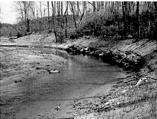
Photograph 47. Looking downstream from MS Station 38+00 at rock toe protection/root wad and rock vane installed at MS Station 37+17. (4/7/04)
