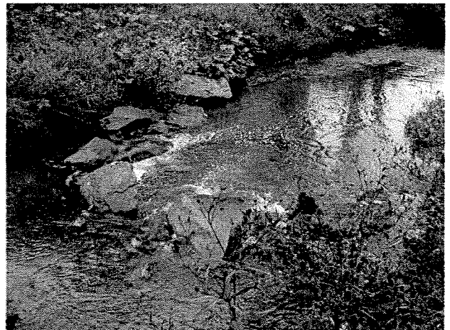
Photograph 18. Rock J vane installed at MS Station 57+66. (9/27/04)
