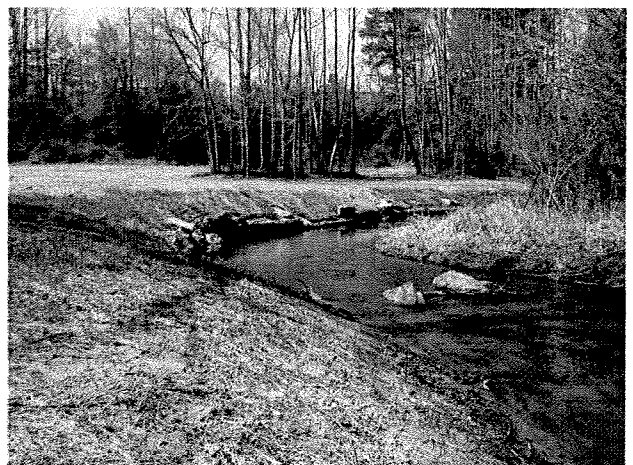
Photograph 10. Looking downstream from MS Station 65+50 at rock J vane, log toe protection, and root wad. (4/7/04)
