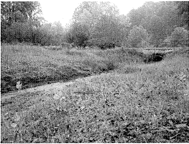
Photograph 31. Downstream face of culvert installed at MC Station 13+29. (9/27/04)
