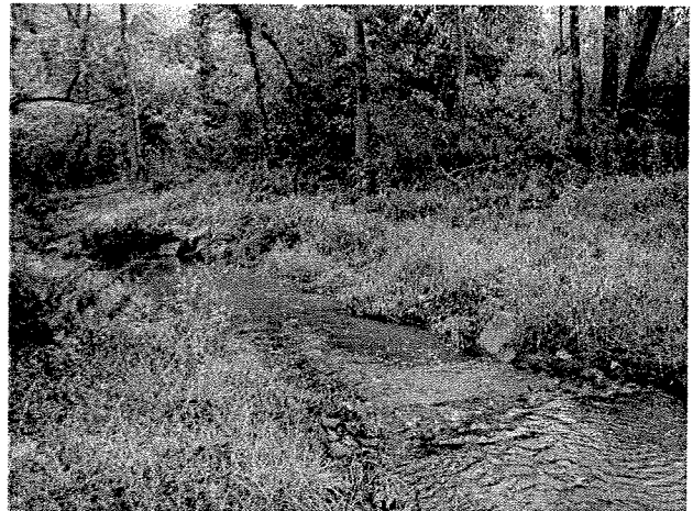
Photograph 46. Looking downstream at rock cross vane installed at MS Station 38+20. (9/27/04)
