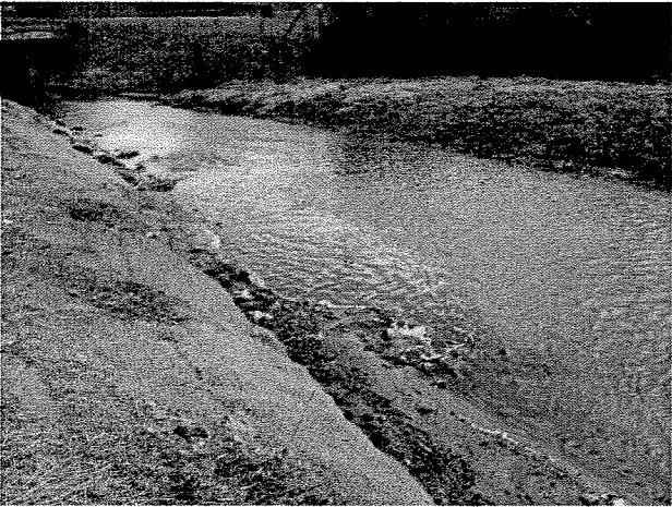
Photograph 129. Looking downstream from rock cross vane installed at MS Station 1+50 area. (4/7/04)
