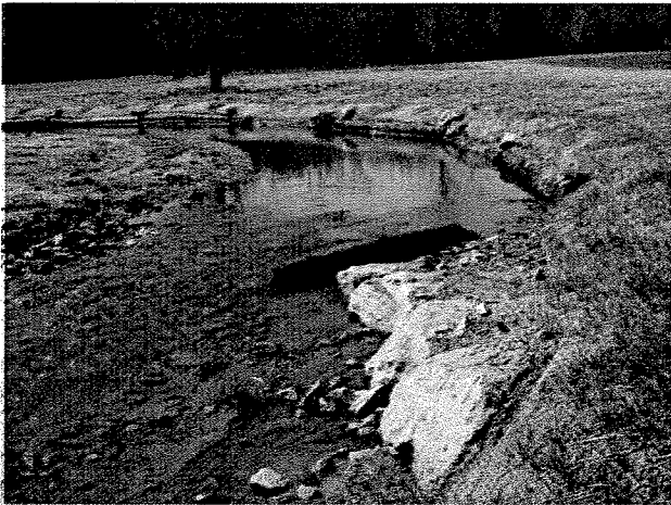
Photograph 105. Looking upstream at rock vane installed at MS Station 11+10. (4/7/04)
