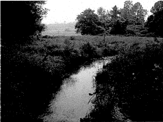
Photograph 9. Looking downstream from LT Station 2+25. (9/27/04)
