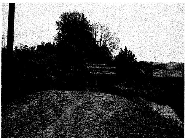
Photograph 132. Gravel path installed at downstream end of main stem for cattle access to NC 18 culvert. (9/27/04)
