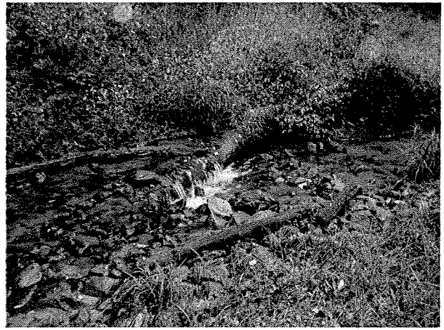
Photograph 8. Log vane installed at LT Station 1+80. (9/27/04)
