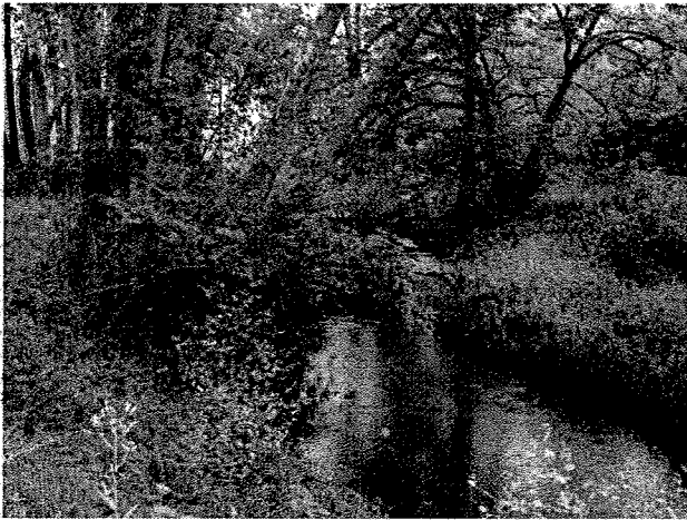
Photograph 7. Looking downstream from rock J vane installed in existing MS channel. (9/27/04)
