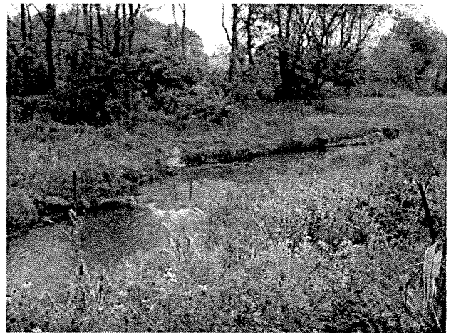
Photograph 116. Rock cross vane installed at MS Station 6+58. (9/27/04)
