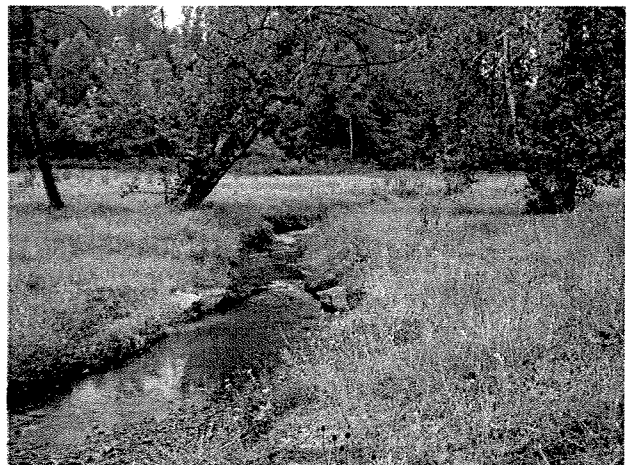
Photograph 70. Looking upstream at rock cross vane installed at MS Station 27+33. (9/27/04)
