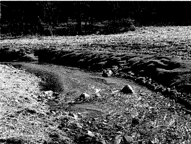
Photograph 21. Looking downstream at rock J vane installed at MC Station 10+14. (1/16/04)
