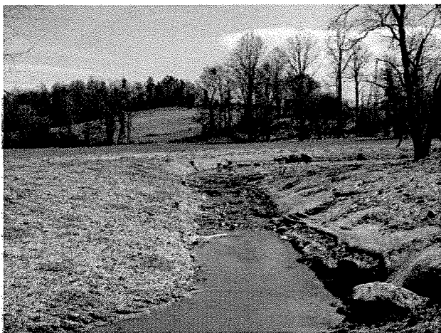
Photograph 45. Looking upstream at rock cross vane installed at LT Station 12+44. (4/7/04)
