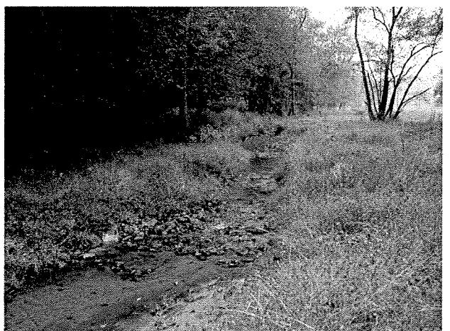
Photograph 6. Looking downstream at rock vane installed at LT Station 0+94. (9/27/04)
