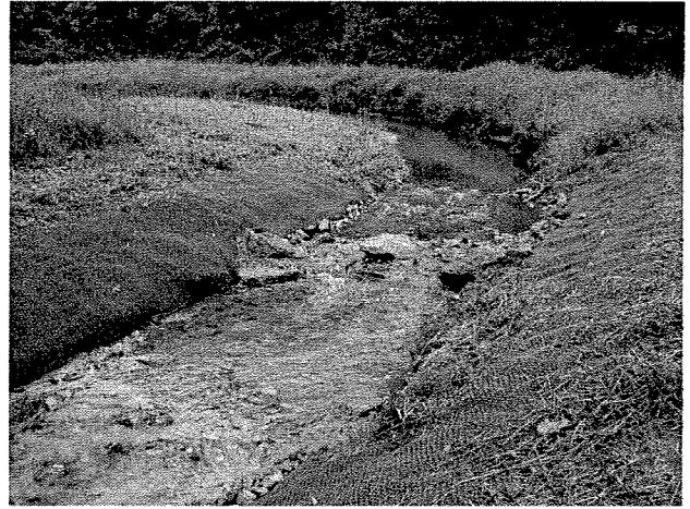
Photograph 20. Looking upstream at rock J vane installed at MC Station 9+72. (9/27/04)
