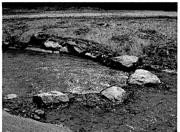
Photograph 66. Rock J vane installed at MS Station 29+10. (4/7/04)
