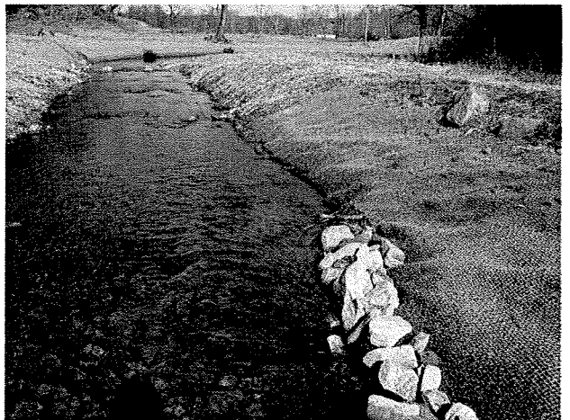
Photograph 24. Log vane installed at MC Station 11+26. (1/16/04)
