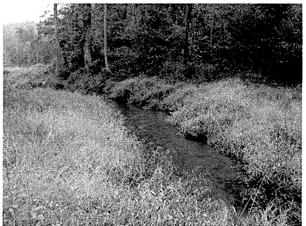
Photograph 52. Looking downstream from MS Station 35+00 at installed rock toe protection and root wads. (9/27/04)
