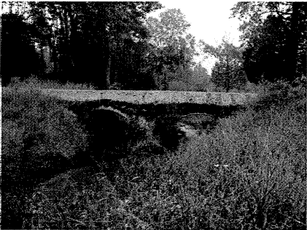
Photograph 57. Downstream face of culvert installed at MS Station 33+00. (9/27/04)
