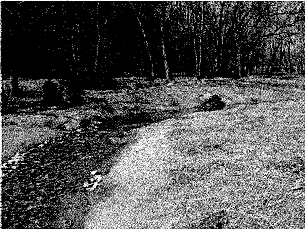
Photograph 15. Looking downstream at rock cross vane and root wad installed between LT Stations 3+58 and 3+90. (4/7/04)
