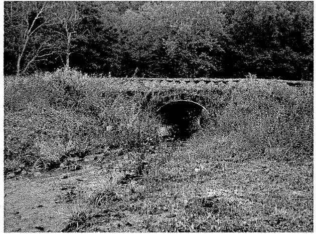
Photograph 40. Downstream face of culvert installed at LT Station 10+38. (9/27/04)
