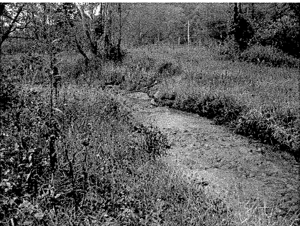
Photograph 53. Looking downstream at rock J vane installed at MC Station 21+63. (9/27/04)
