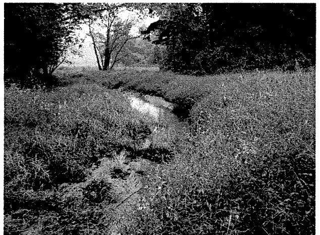
Photograph 4. Looking downstream at log toe protection and root wads installed between LT Stations 0+25 and 0+95. (9/27/04)
