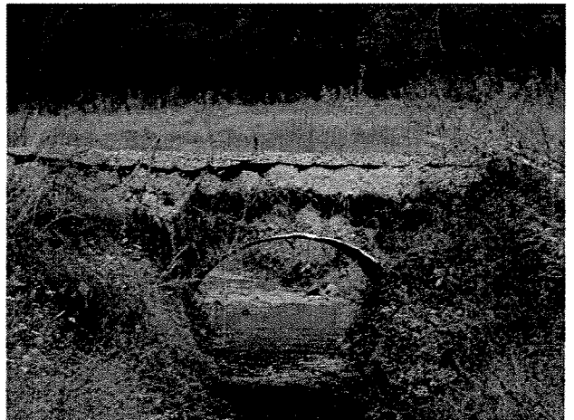
Photograph 30. Upstream face of culvert installed at MC Station 13+29. (9/27/04)
