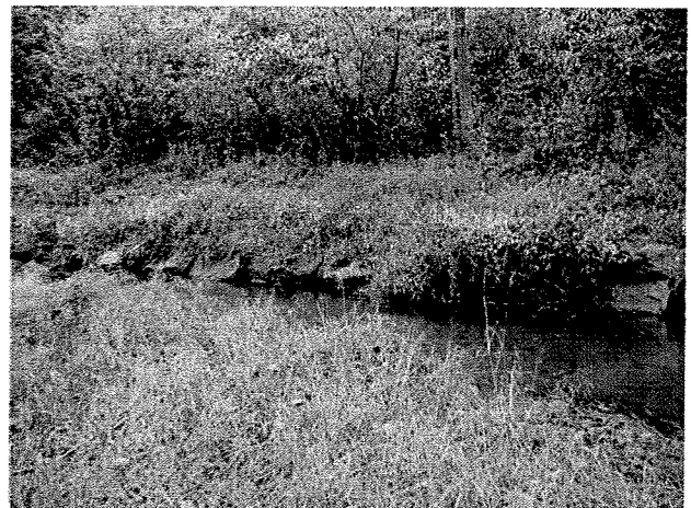
Photograph 48. Looking downstream at rock toe protection installed between MS Station 37+80 and 37+25. (9/27/04)
