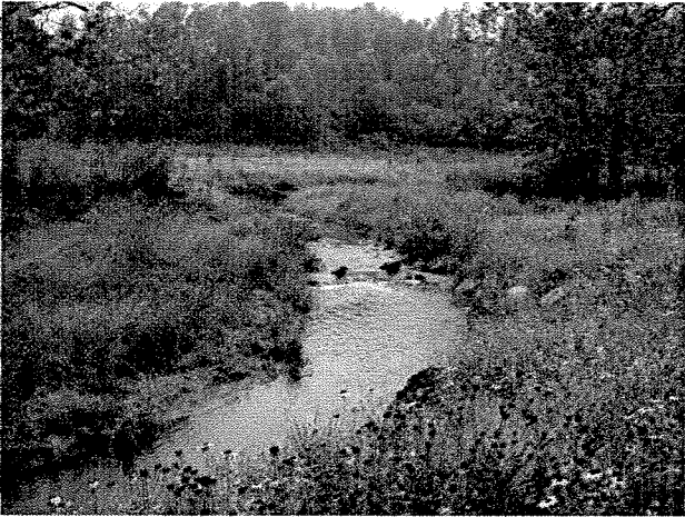
Photograph 75. Looking upstream at rock J vane installed at MS Station 24+03. (9/27/04)
