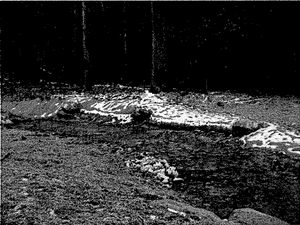
Photograph 3. Looking downstream at log toe protection installed between LT Stations 1+50 and 1+90 to protect large trees. (12/18/03)
