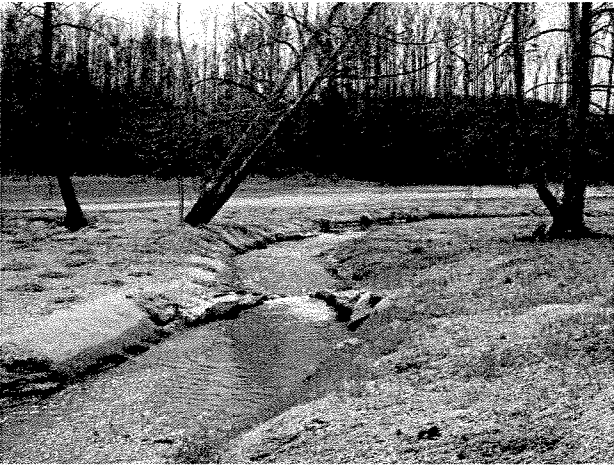
Photograph 69. Looking upstream at rock cross vane installed at MS Station 27+33. (4/7/04)
