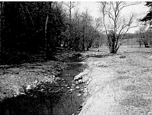
Photograph 5. Looking downstream at rock vane installed at LT Station 0+94. (4/7/04)
