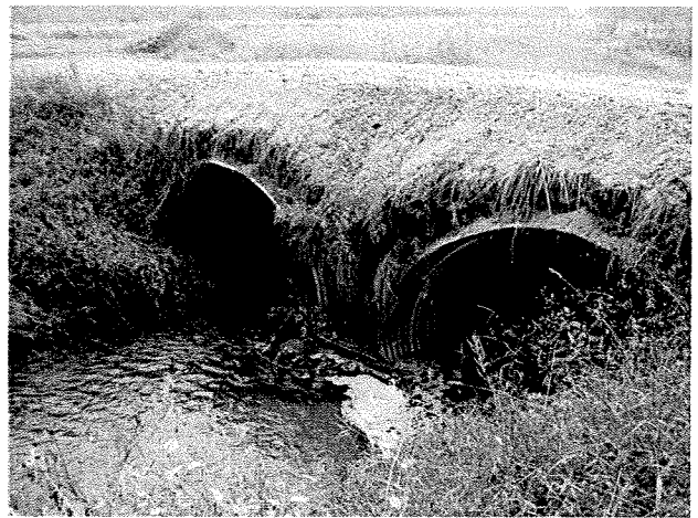
Photograph 56. Upstream face of culvert installed at MS Station 33+00. (9/27/04)
