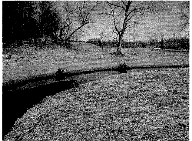
Photograph 28. Looking downstream at root wads installed between MC Stations 12+45 and 12+65. (1/16/04)
