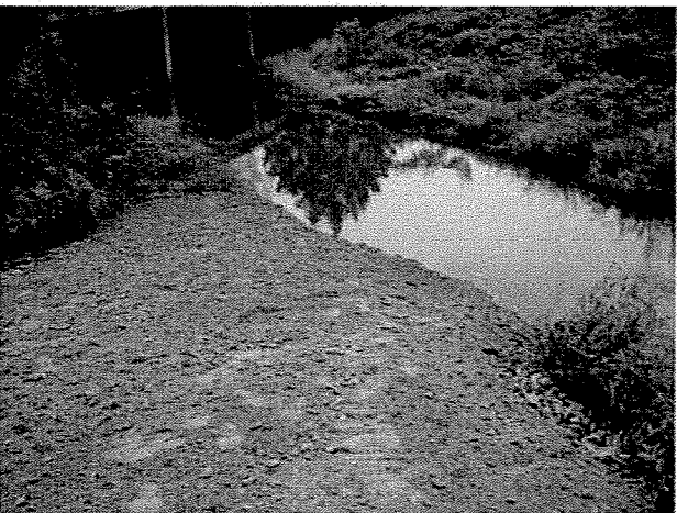
Photograph 131. Gravel path installed at downstream end of main stem for cattle access to NC 18 culvert. (9/27/04)
