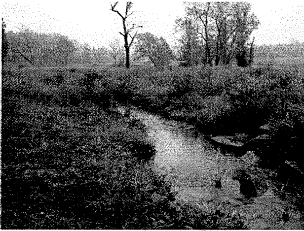
Photograph 31. Looking downstream from rock J vane installed at LT Station 8+38. (9/27/04)
