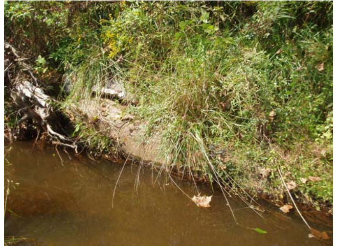
BWPA2 facing left bank
