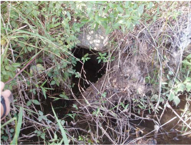
BWPA15 facing left bank
