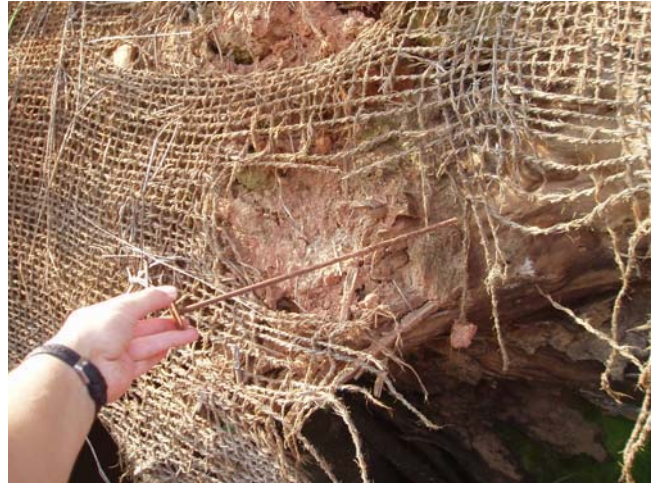
BWPA8 facing left bank
