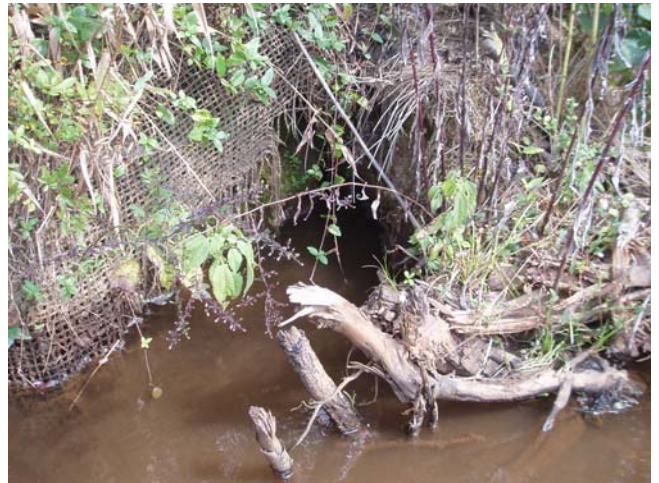
BWPA4 facing left bank
