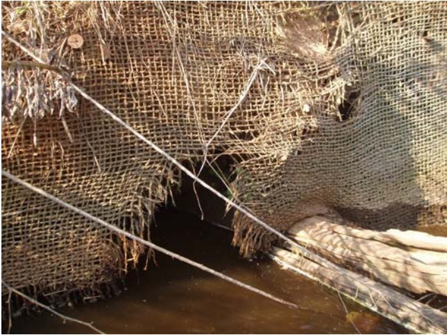
BWPA7 facing left bank
