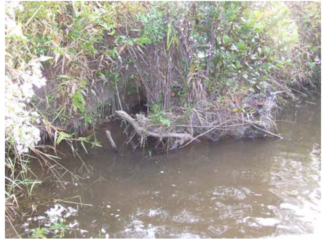
BWPA4 facing left bank
