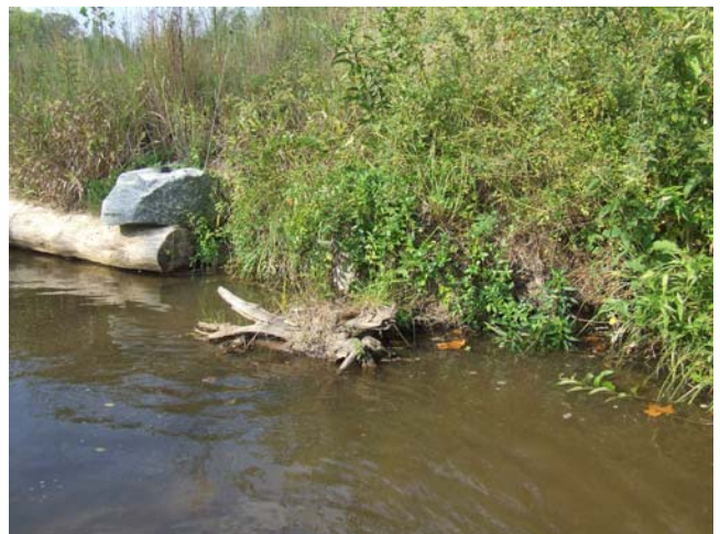
BWPA24 facing downstream
