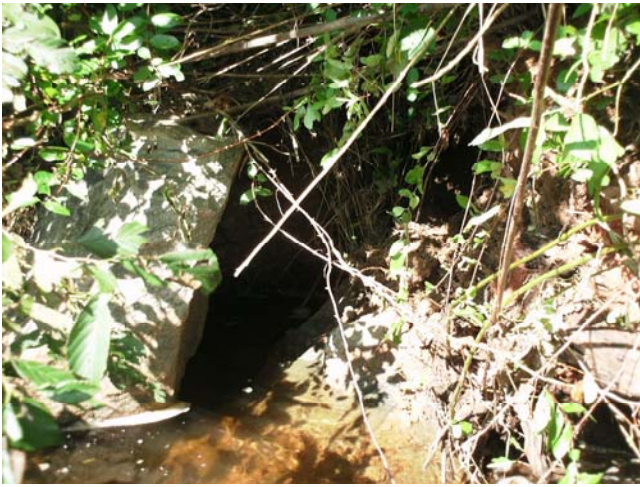
BWPA2 facing right bank
