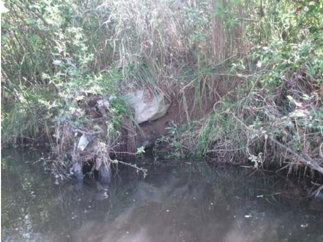
BWPA22 facing right bank
