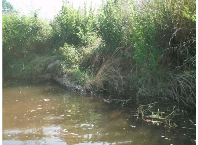
BWPA23 facing upstream
