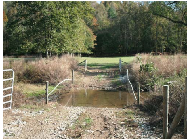
PS16 facing right bank
