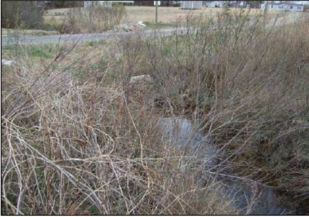
Facing north (downstream) at culvert under Norma Drive
