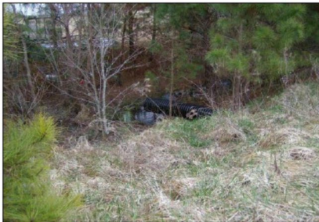
Drain pipe entering perimeter ditch along northeast property boundary
