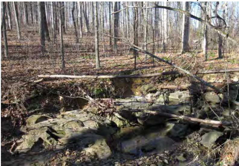
PP #16 – UT1 Preservation Reach (01/03/10)
