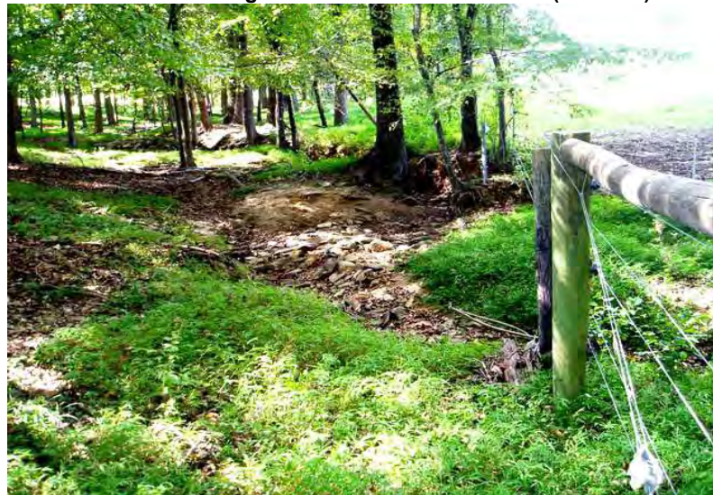
PP #8 – Looking up UT3 from lower end (10/02/13)
