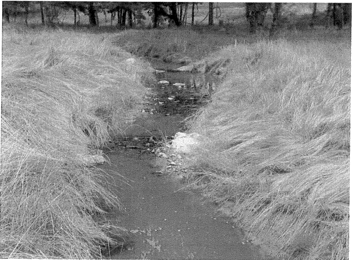
Reach #2. Photograph Point #6. Looking upstream. 06/15/04 7
