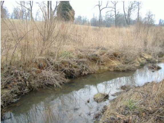
Photo 3: Representative problem root wad and bank erosion (10+82.28 along plan view). Root wads located in bank along left side of picture.
