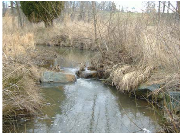
Photo 4: Representative problem cross vane (12+75.47 along plan view).
