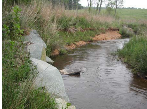
Photo 2: Representative problem j-hook and bank erosion (Station 15+03 along plan view).
