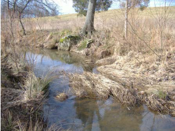
Photo 1: Representative grass aggradation problem area (19+06.73 along plan view).
