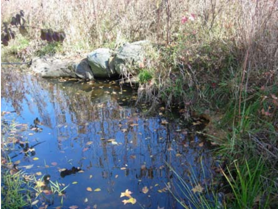
Photo 1: Representative jhook and bank erosion problem area (Station No. 16+42; bank erosion is in the right corner of picture; view downstream; 11-6-2008).
