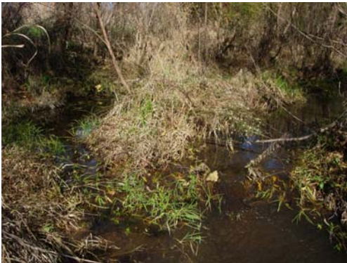
Photo 3: Representative midbar problem area (Station No. 18+02; view downstream; 11-6-2008).
