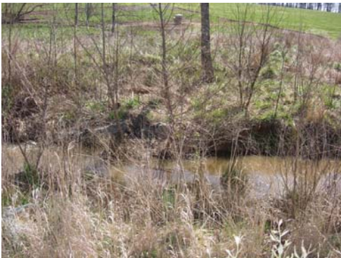
Photo 5: Representative bank erosion problem area (Station No. 10+83; view across stream toward left bank on 3-20-2008).
