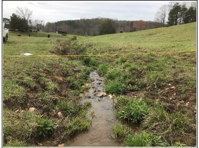
Upper UT5 at XS-1, downstream (4/9/18)
