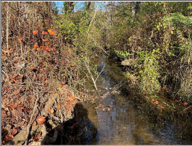
PP-33: Reach UT4B, upstream, Station 13+75
