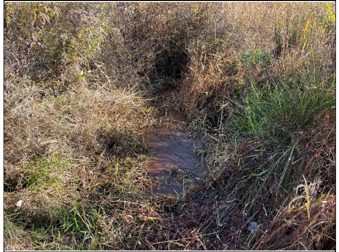
PP-38: Reach UT5, upstream, Station 17+75
