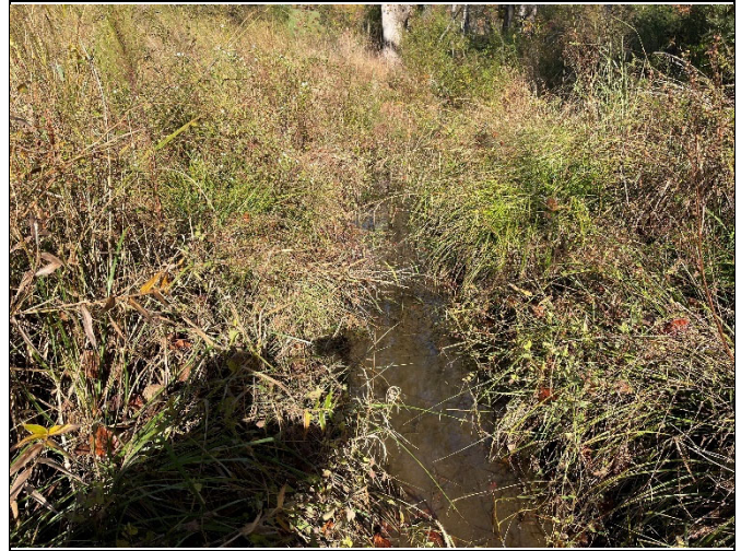
PP-32: Reach UT4B, upstream, Station 15+50
