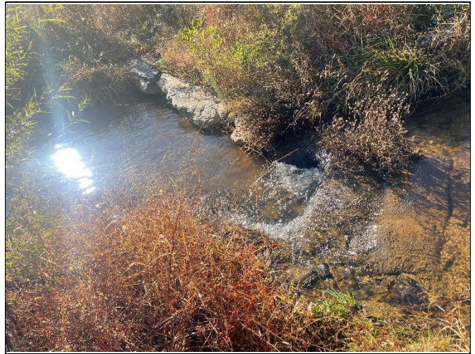
PP-20: Reach 7, downstream, Station 23+25
