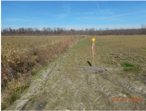
(13) PS7 (looking north along Reach B3)
