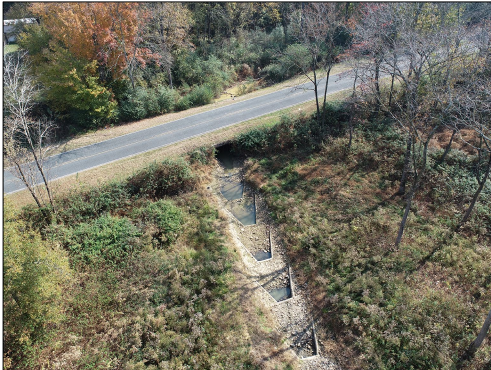
Site Outfall and Drop Structure, taken November 8, 2023
