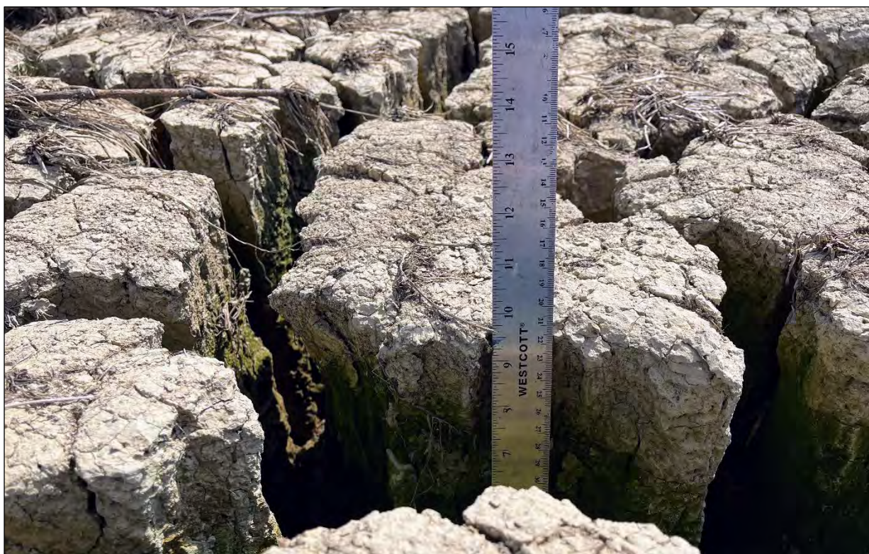
Photo 4: Depth to un-cracked sub-grade/soil
