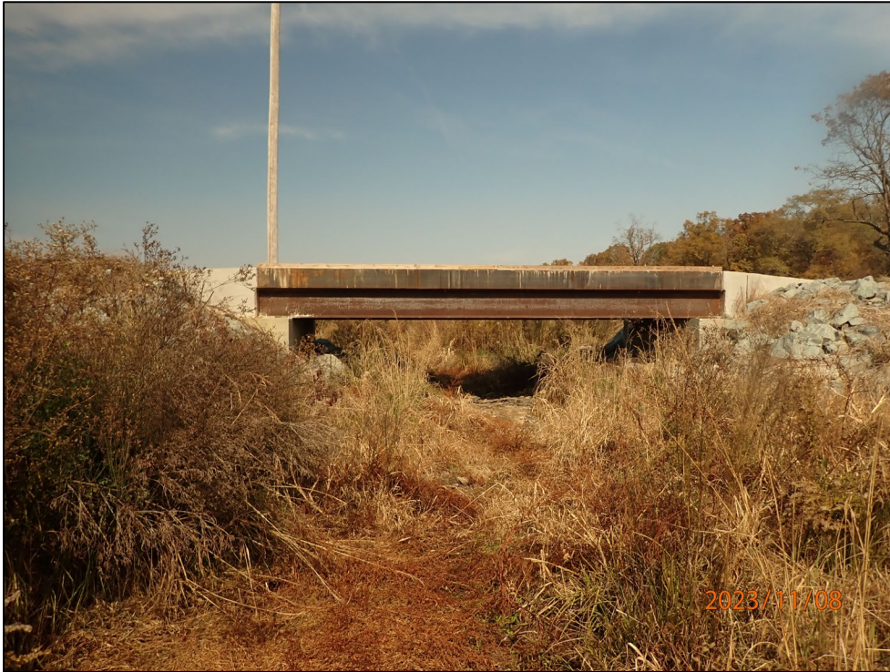
Bridge Crossing on Waxhaw Branch, taken November 8, 2023
