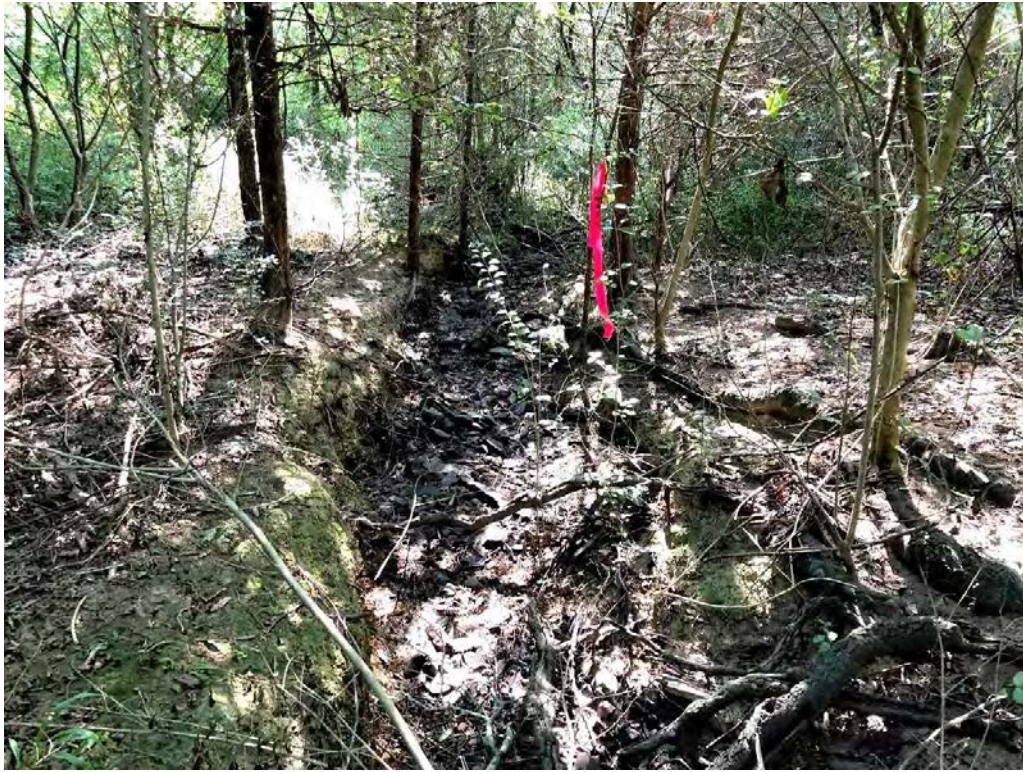
Photo 13: UT-1 Data Point facing downstream – July 15, 2020
