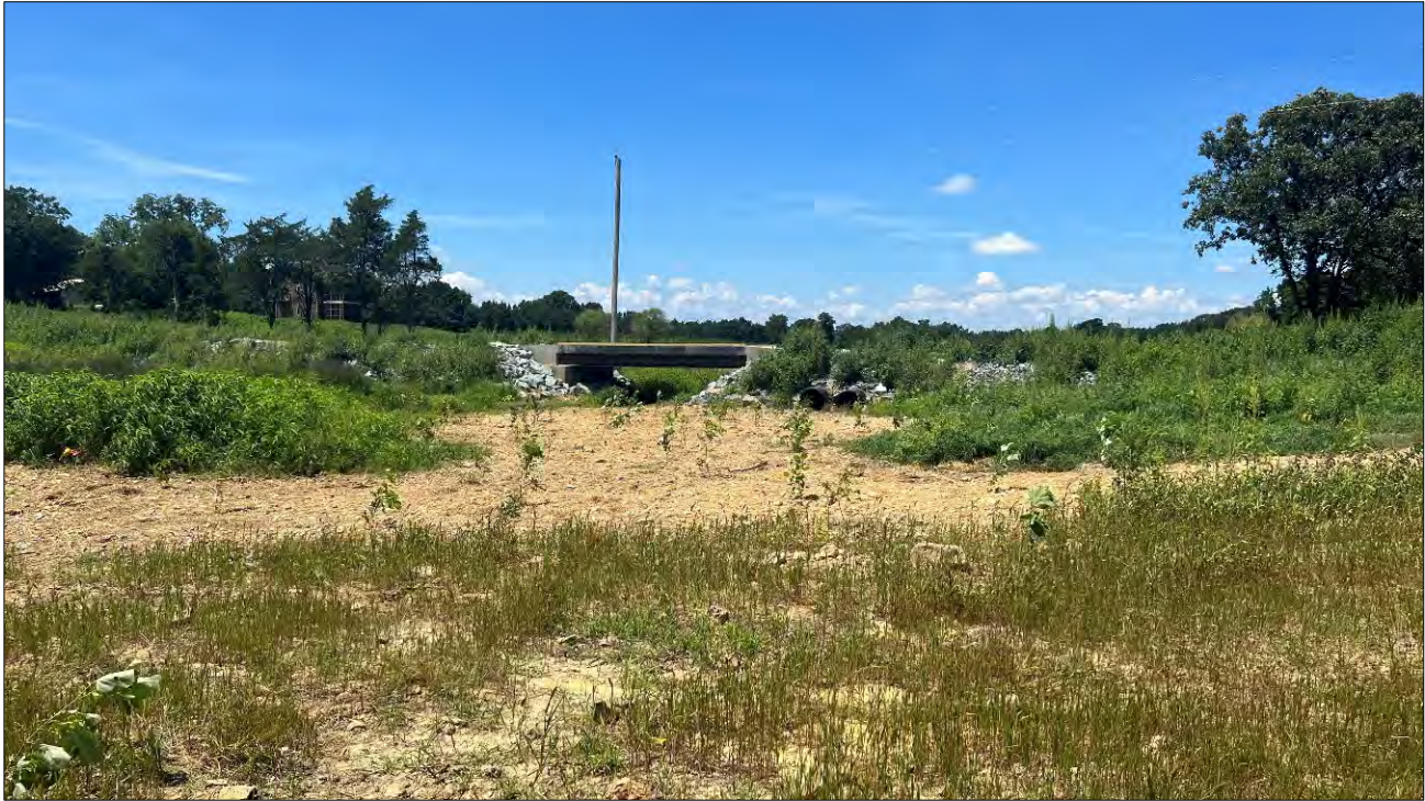
1-gallon containerized planting, Waxhaw Branch, old access road/bridge construction area, 07/28/2022
