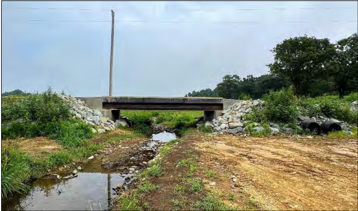
Bridge Crossing on Waxhaw Branch, taken July 15, 2022
