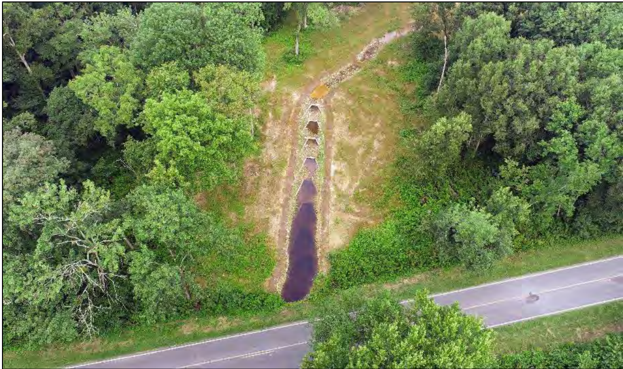
Site Outfall and Drop Structure, taken July 15, 2022
