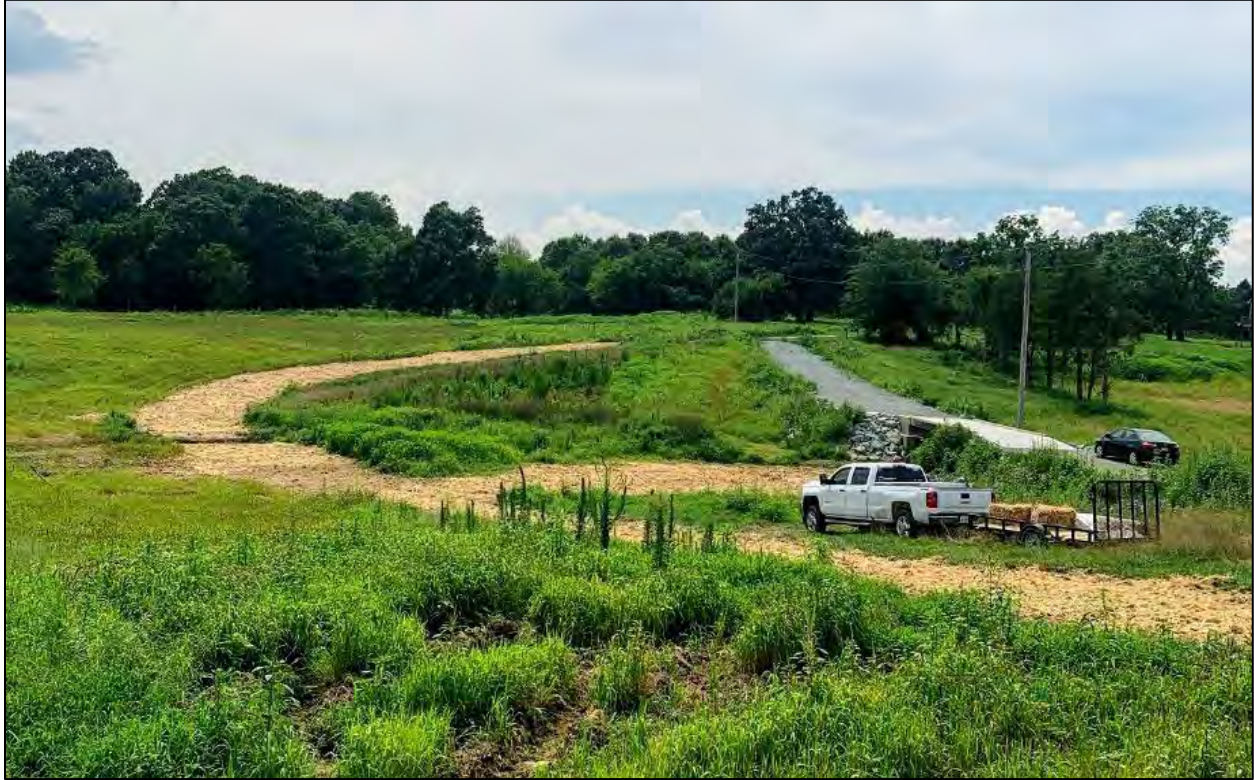
Old Road Removed, New Road Build, taken July 22, 2022
