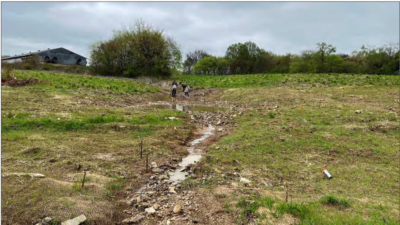
Live stake planting, UT2 Marsh Treatment Area, 04/07/2022
