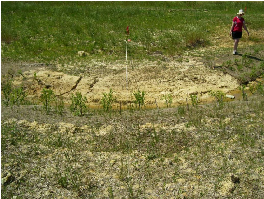
R2 PXS1: Looking at Left Bank (May 29, 2008)
