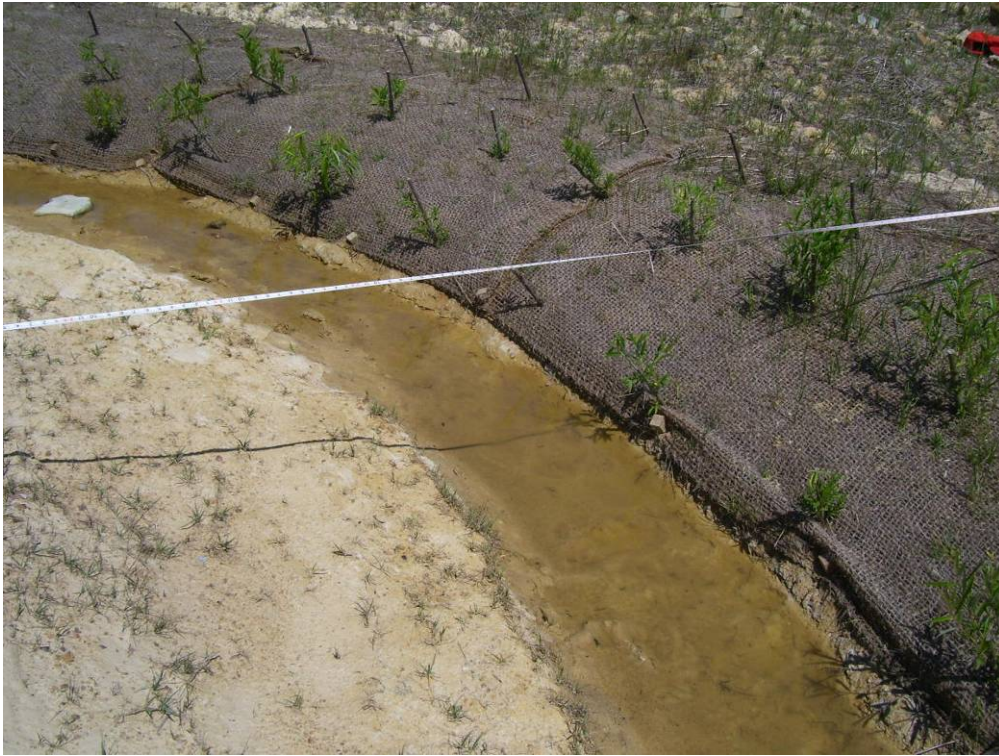
R2 PXS1: Looking Upstream (May 29, 2008)
