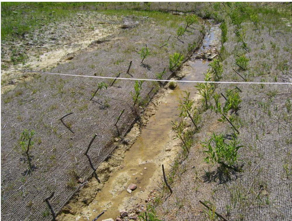
R2 RXS2: Looking Downstream (May 29, 2008)
