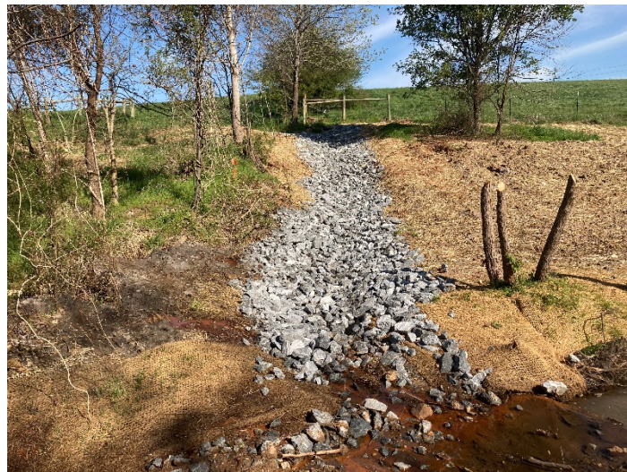
UT2 R1 – Photo Point 21 looking northwest (4/12/2022)
