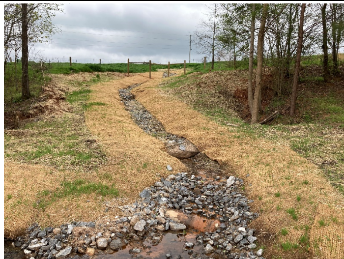
UT2 R1 – Step-Pool Stormwater Conveyance looking southeast (4/12/2022)
