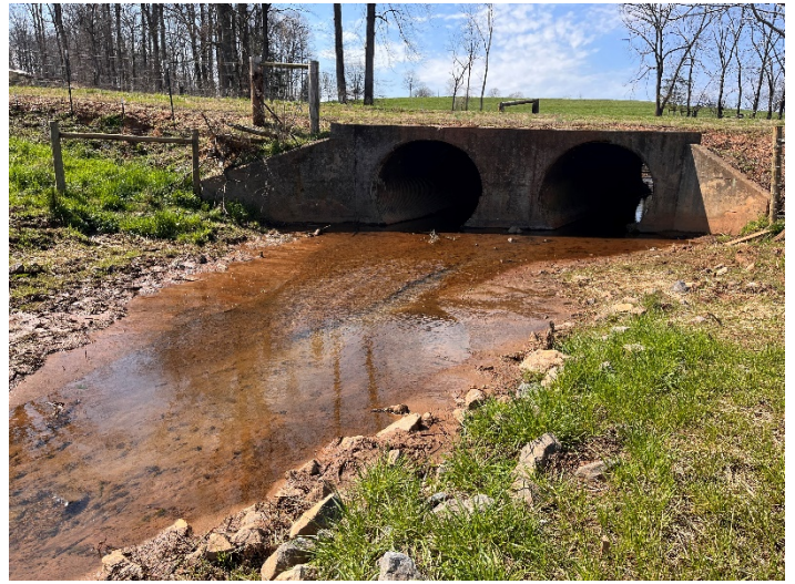
Wyant R2 Crossing – Looking upstream outlet (3/8/2022)
