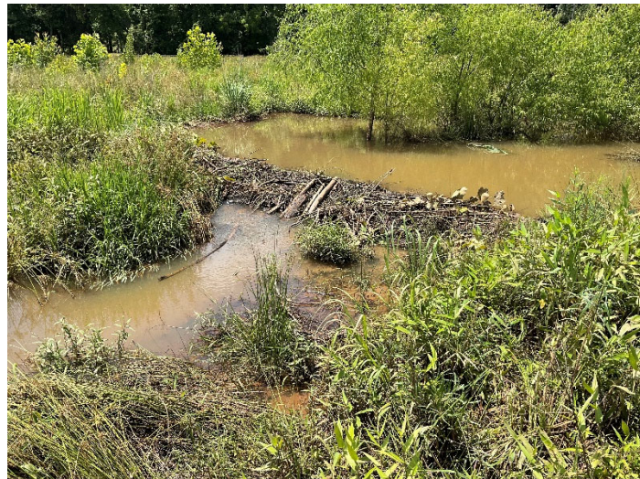
Wyant Creek R4 – STA:139+50 Beaver Dam Pre-Removal (6/23/2023)
