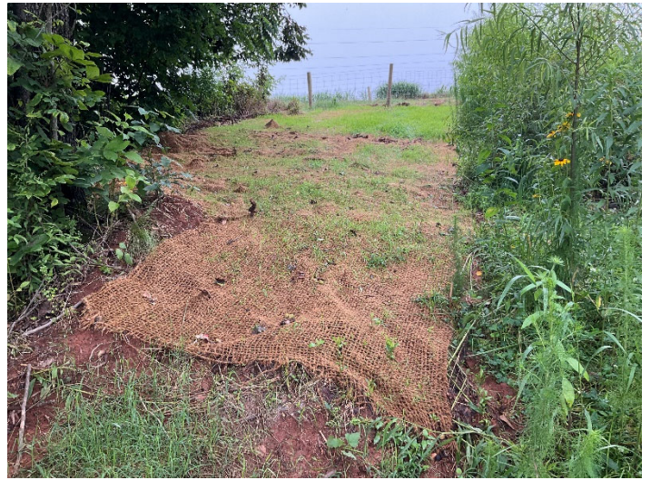
UT2 R1 – Repaired Gully looking upslope (6/23/2023)
