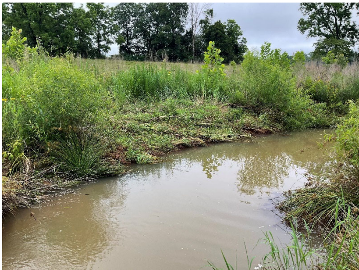
Wyant Creek R4 – STA:128+75 (XS15) Bank Repair (6/23/2023)
