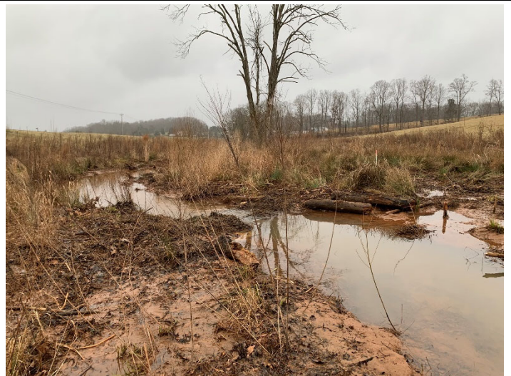
Wyant Creek R1 – STA:102+50 Beaver Dam Removed (2/6/2023)
