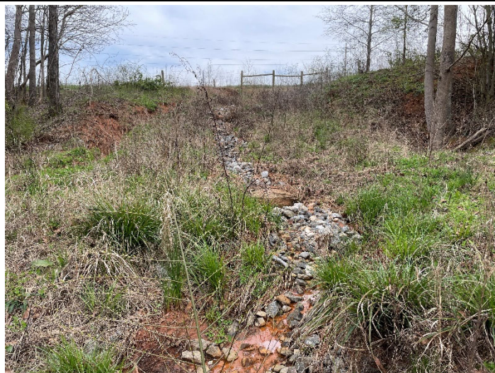
BMP 3 - looking up from bottom (3/22/2023)
