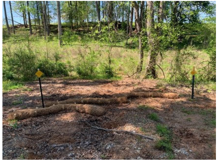
UT2 R3 – Off-Site Sediment Repair (5/2/2023)
