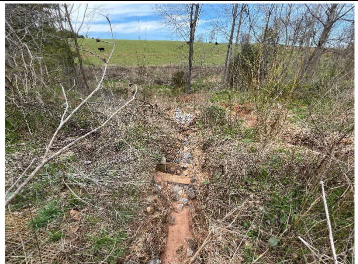
BMP 3 - looking down from outside easement (3/22/2023)
