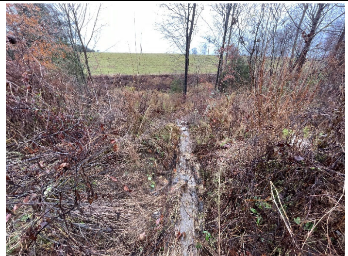
BMP 3 - looking down from top outside fence (11/30/2022)
