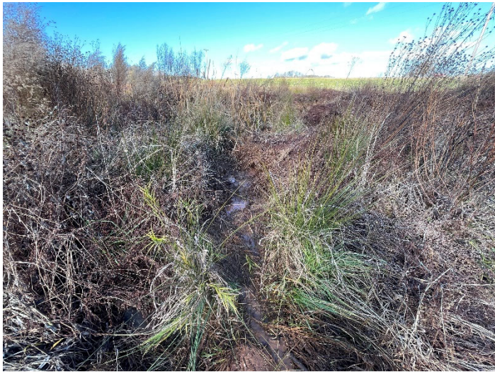
BMP 1 - looking up from bottom (11/30/2022)
