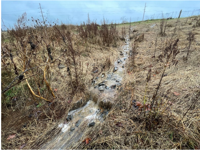
BMP 3 - looking up from outside fence (11/30/2022)
