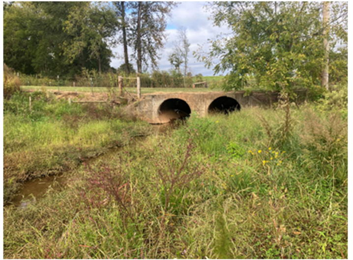
Wyant Road Culvert – Improved Erosion Mitigation (10/3/2022)
