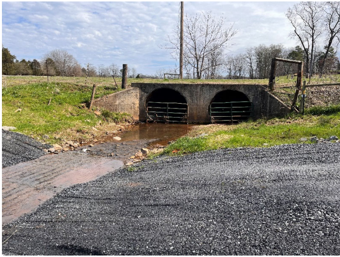
Wyant R2 – Photo Point 6A downstream inlet (3/8/2022)
