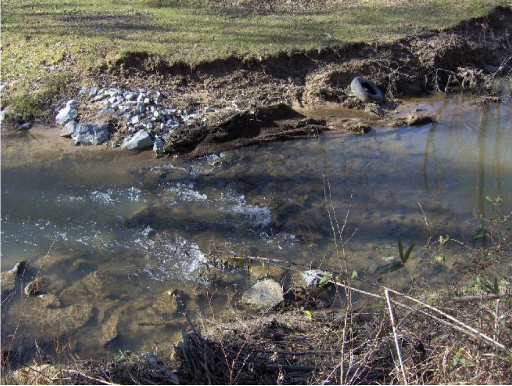
STRUCTURE # 38 – BANK REINFORCEMENT / ROCK-VAIN
