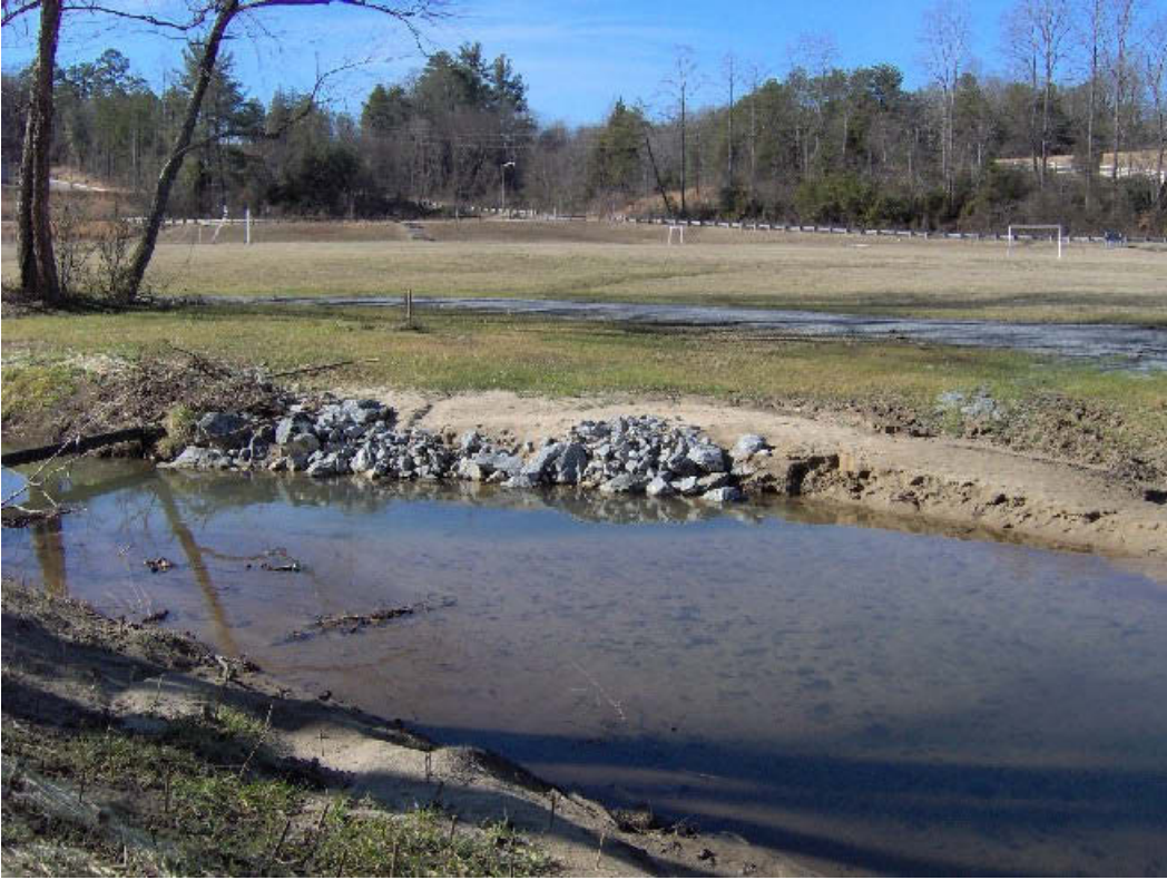
STRUCTURE # 28 - BANK REINFORCEMENT
