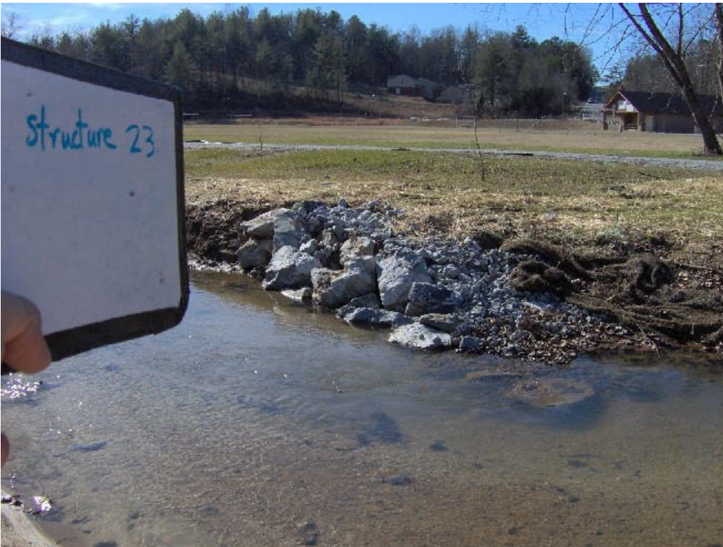
STRUCTURE # 23 – BANK REINFORCEMENT
