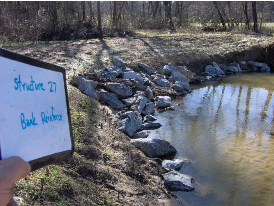
STRUCTURE # 27 – BANK REINFORCEMENT
