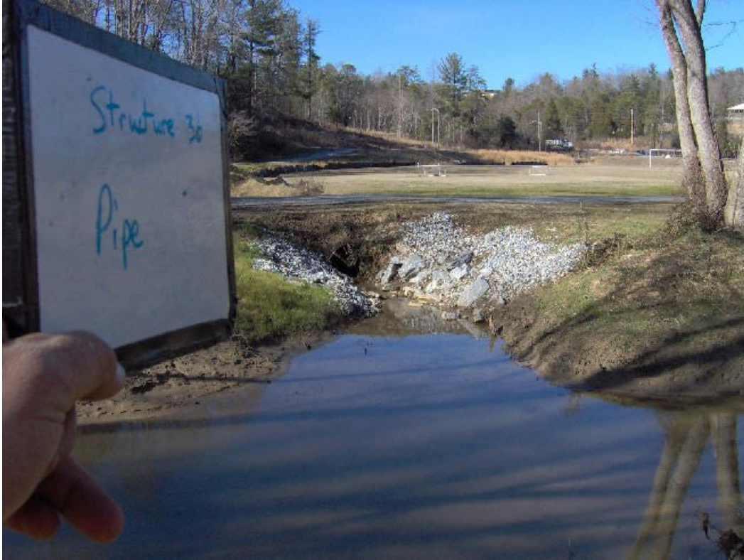
STRUCTURE # 36 – EXISTING PIPE
