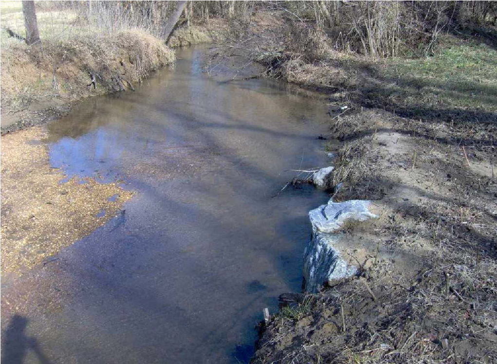
STRUCTURE #1 – CROSS-VAIN (BEGINNING OF PROJECT)
