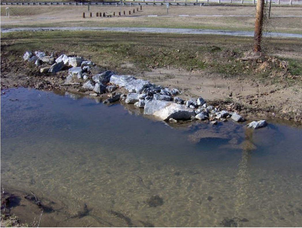
STRUCTURE # 21 – BANK REINFORCEMENT
