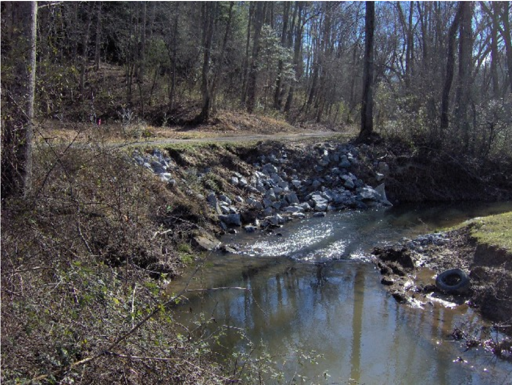
STRUCTURE # 38 – BANK REINFORCEMENT / ROCK-VAIN
