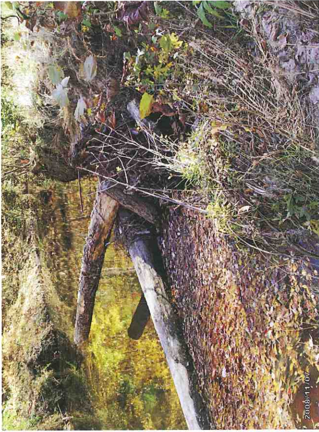
Problem Area 9 - log vane displaced
