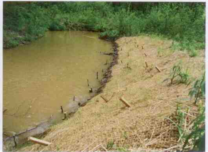
STATION 27+25 – RIGHT BANK REPAIR
