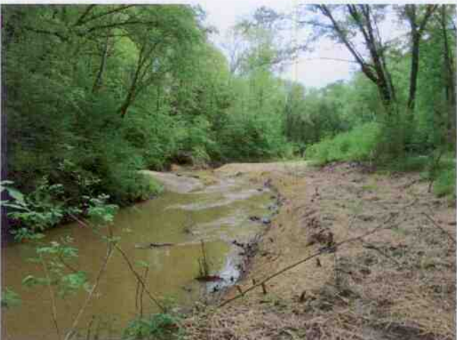
STATION 44+00 – RIGHT BANK REPAIR
