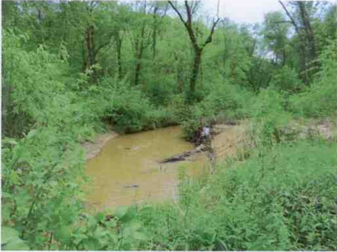
STATION 36+75 – RIGHT BANK REPAIR
