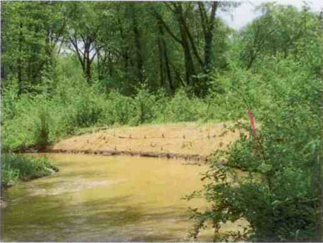
STATION 27+25 – RIGHT BANK REPAIR
