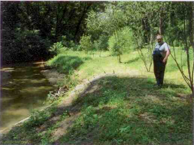
STATION 41+00 – RIGHT BANK REPAIR
