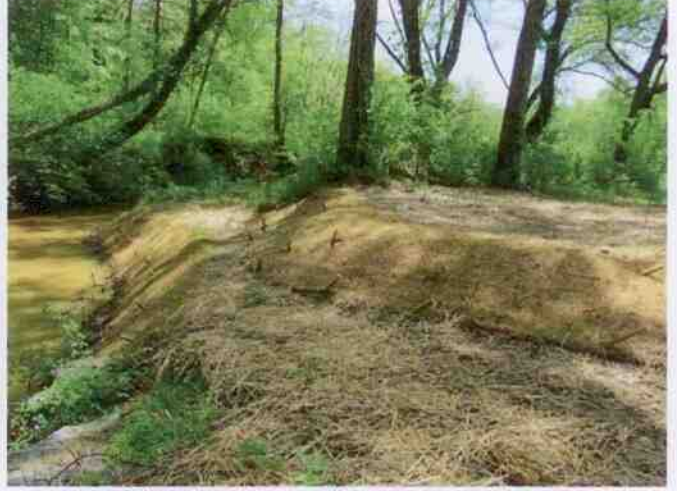
STATION 31+50 – RIGHT BANK REPAIR
