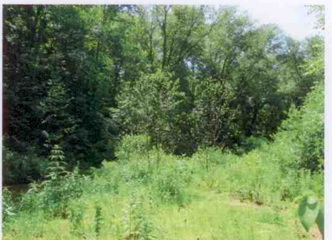
STATION 46+50 – RIGHT BANK REPAIR
