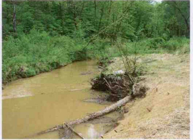
STATION 35+00 – RIGHT BANK REPAIR
