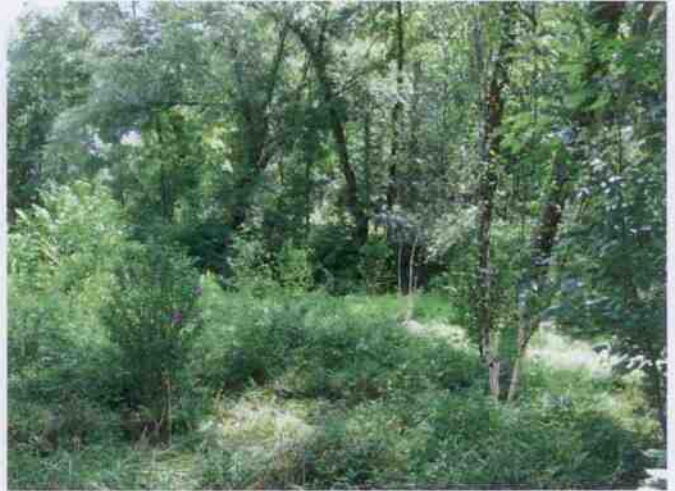
STATION 31+50 – RIGHT BANK REPAIR
