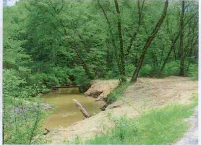
STATION 38+25 – RIGHT BANK REPAIR
