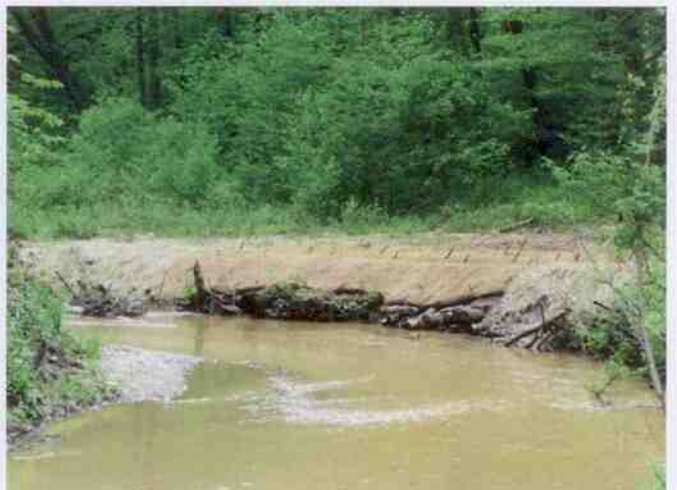
STATION 46+50 – RIGHT BANK REPAIR
