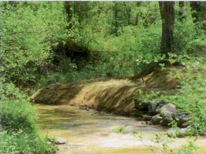
STATION 31+50 – RIGHT BANK REPAIR
