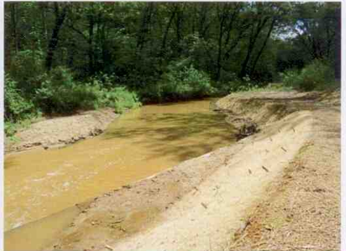
STATION 41+00 – RIGHT BANK REPAIR
