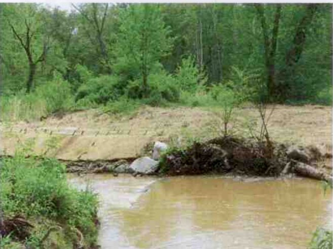
STATION 35+00 – RIGHT BANK REPAIR
