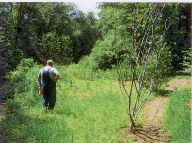
STATION 46+50 – RIGHT BANK REPAIR
