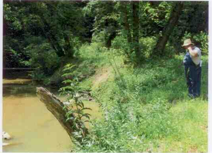
STATION 38+25 – RIGHT BANK REPAIR
