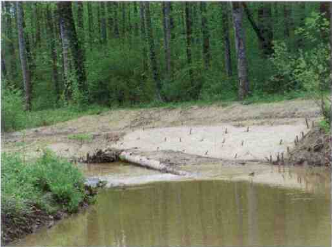
STATION 41+00 – RIGHT BANK REPAIR
