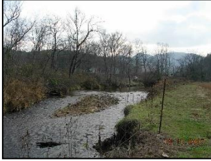
Unstable stream channel on Savannah Creek
