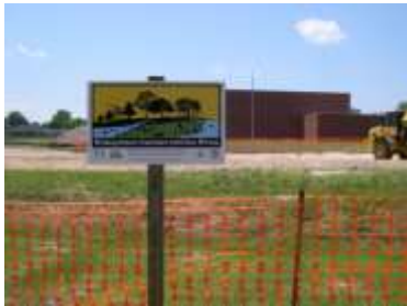
East Tarboro Canal stream restoration site during construction.
