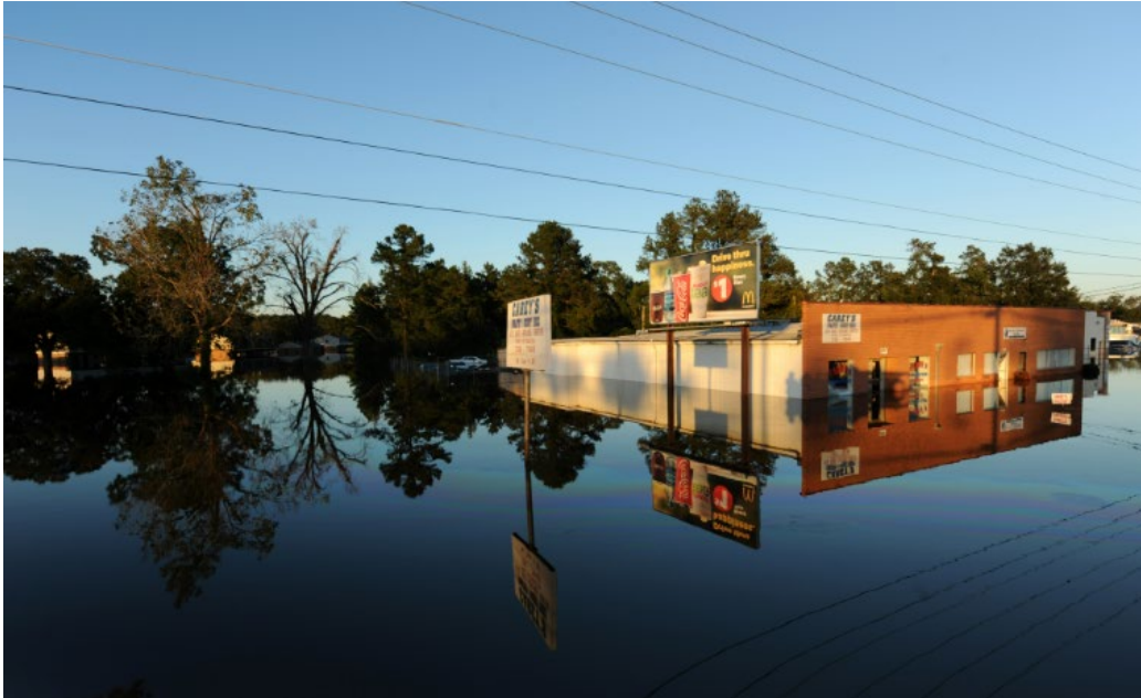
Figure 1.2: NC Flooding Damage
