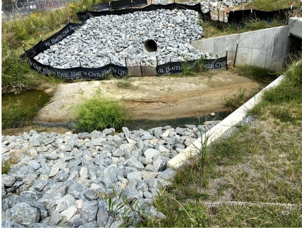
Photo- Culvert completed, surrounding areas stabilized (9/30/21)
