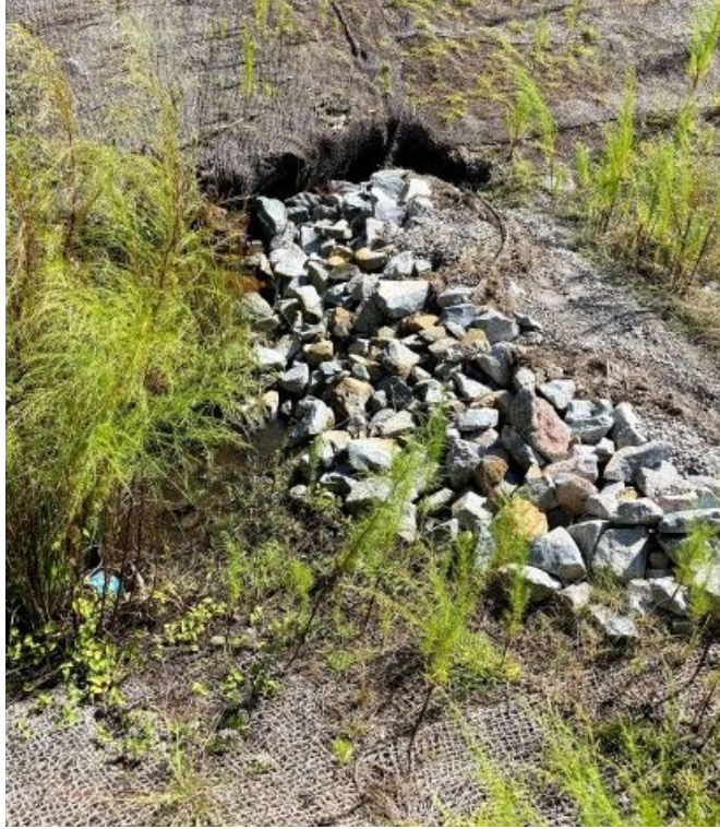
Photo - End cutting around Temporary Rock Silt Check-Type A. (9/23/21)
