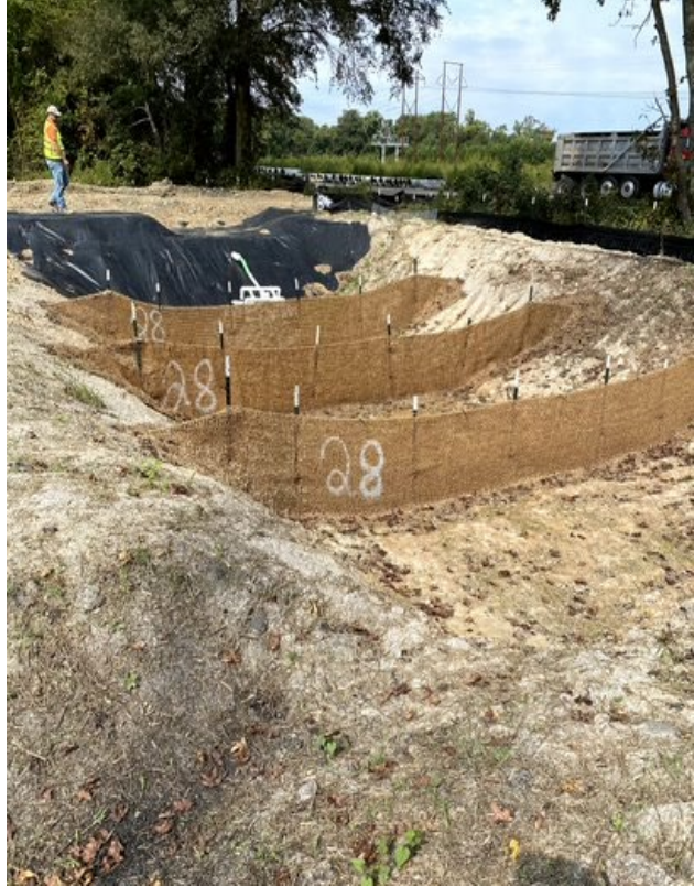
Photo- Skimmer Basins installed in laydown area (9/30/21)
