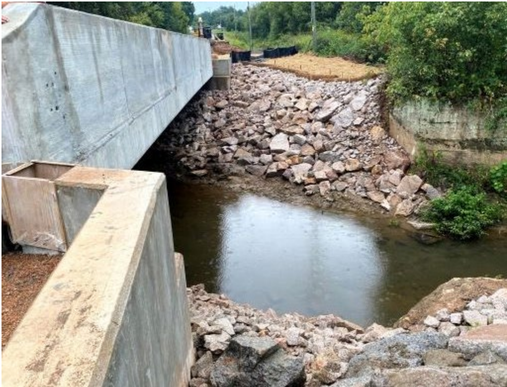
Photo- Bridge #255 over Grant's Creek – Area around Bridge being stabilized (9/16/2021)
