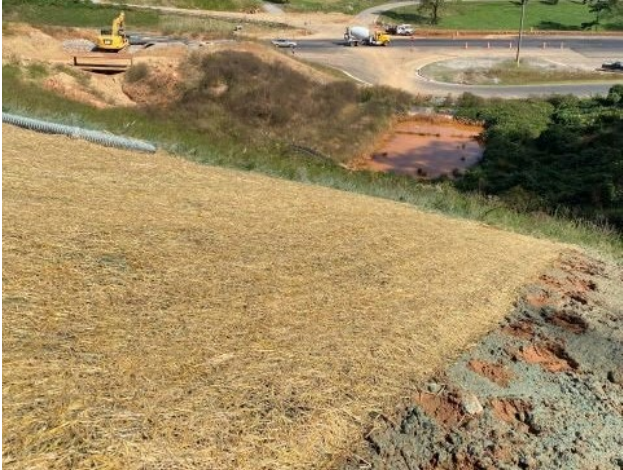
Photo- Waste Area Skimmer Basin and Entrance (10/13/21)
