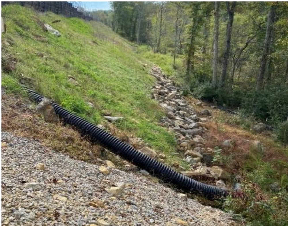
Photo- Slopes Stabilized (10/12/21)
