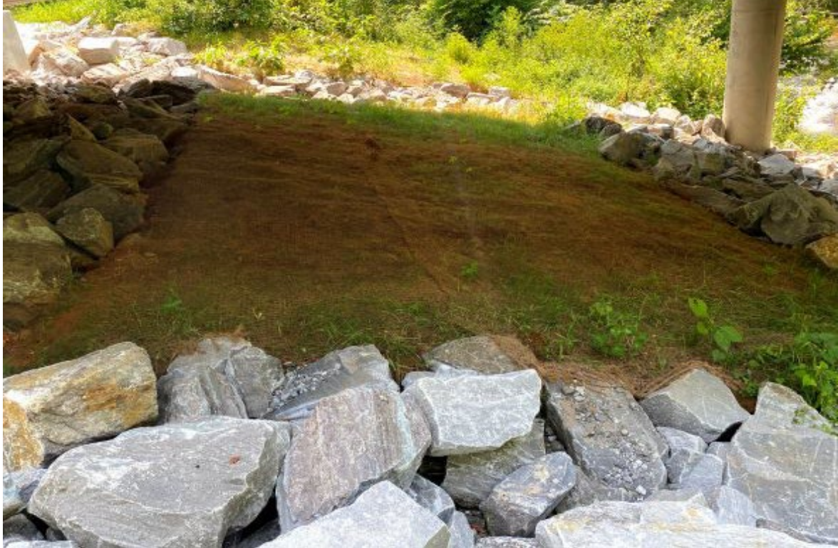
Photo- BR-0124 : Riprap and matted stabilization below bridge (8/25/2021)
