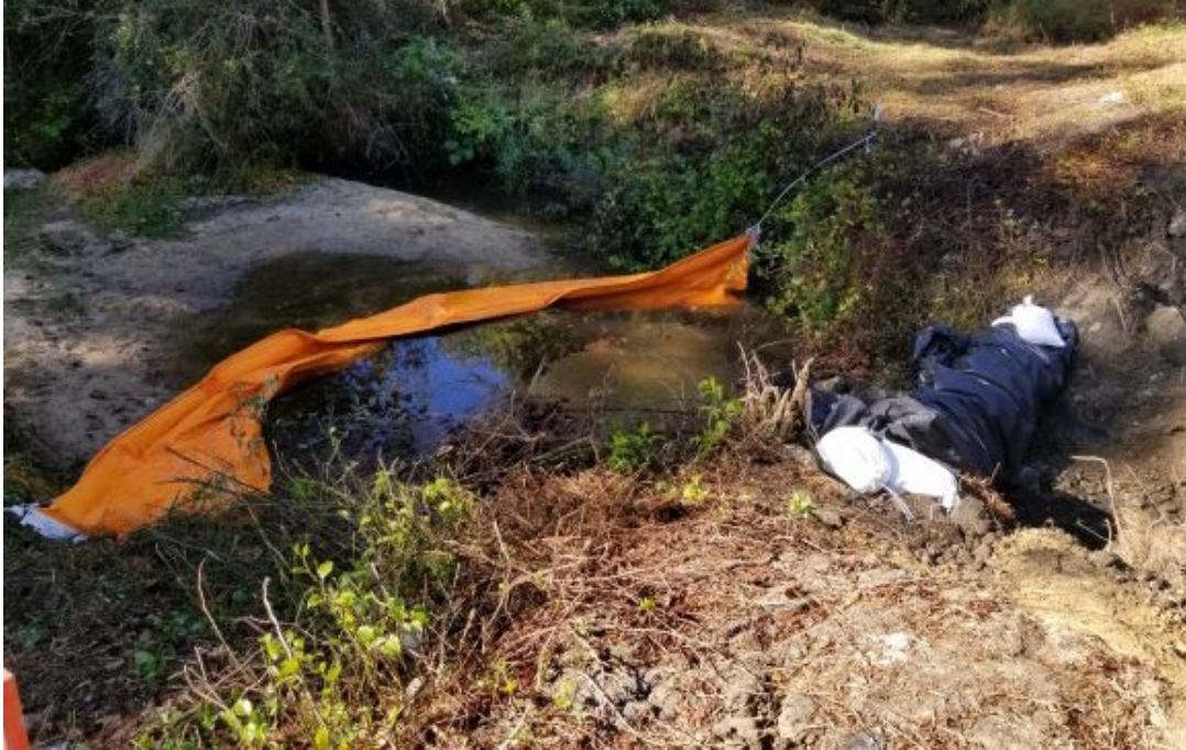
Photo- Impervious Dike and Turbidity Curtain installed downstream (10/19/2021)
