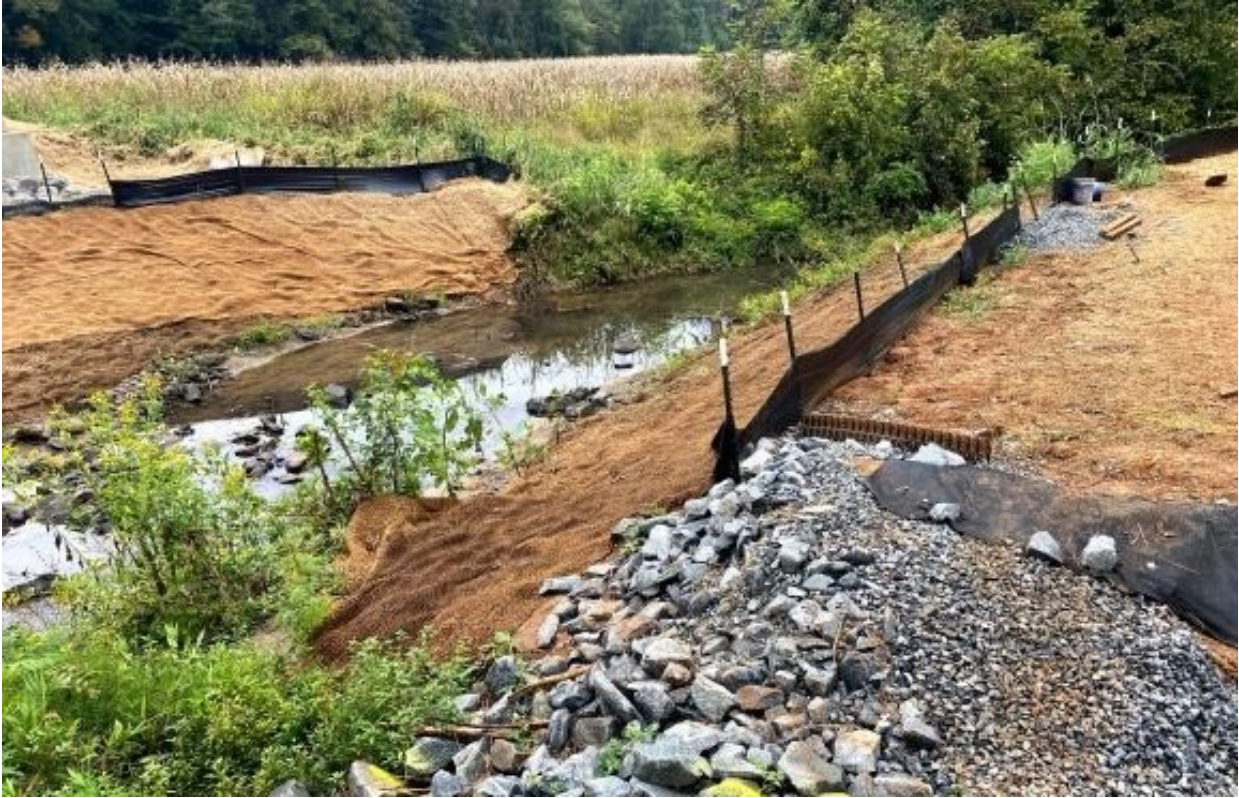
Photo- Bridge #64 over Beaverdam Creek- Additional Silt Fence (9/16/2021)
