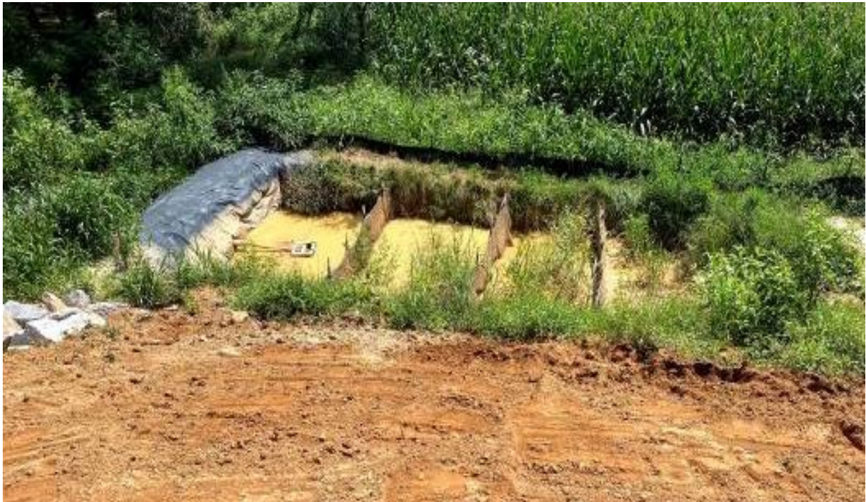
Photo- BR-0125: Basin in the SE corner of the bridge (8/25/2021)
