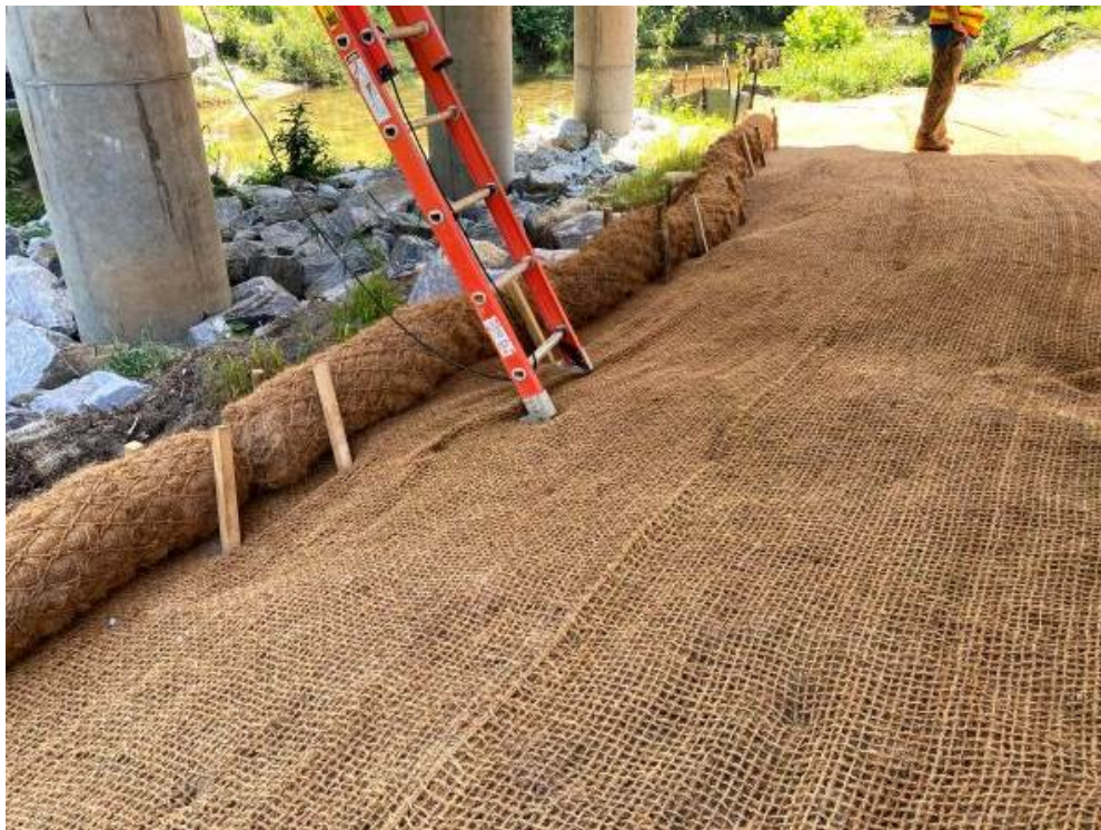
Photo- BR-0125 : Coir Fiber laid as matting and Wattles installed (8/25/2021)
