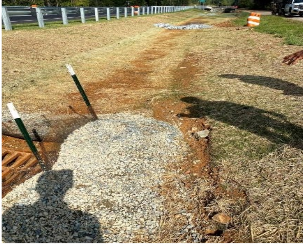
Photo- Ditch line measures installed (10/5/21)
