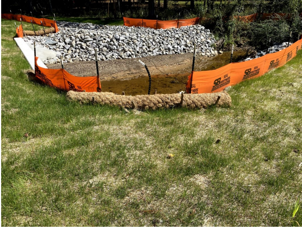
Photo- Riprap armor and silt fence maintained (9/28/2021)
