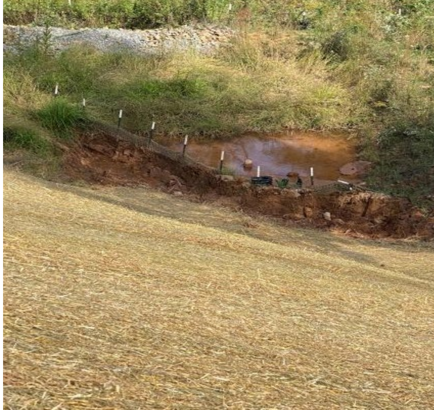
Photo- TRSD-B partially removed for slope grading (10/13/21)
