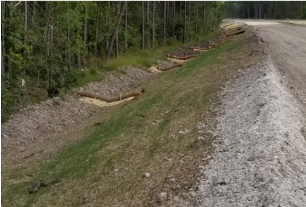
Photo- Grass establishing in ditch with Wattles and polyacrylamide (PAM). (10/4/21)
