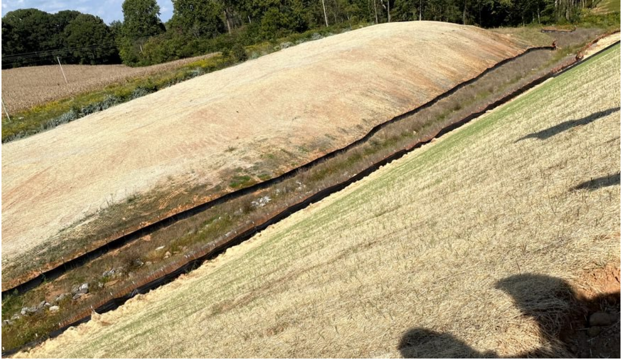
Photo- Channel change and slopes stabilized (9/29/21)
