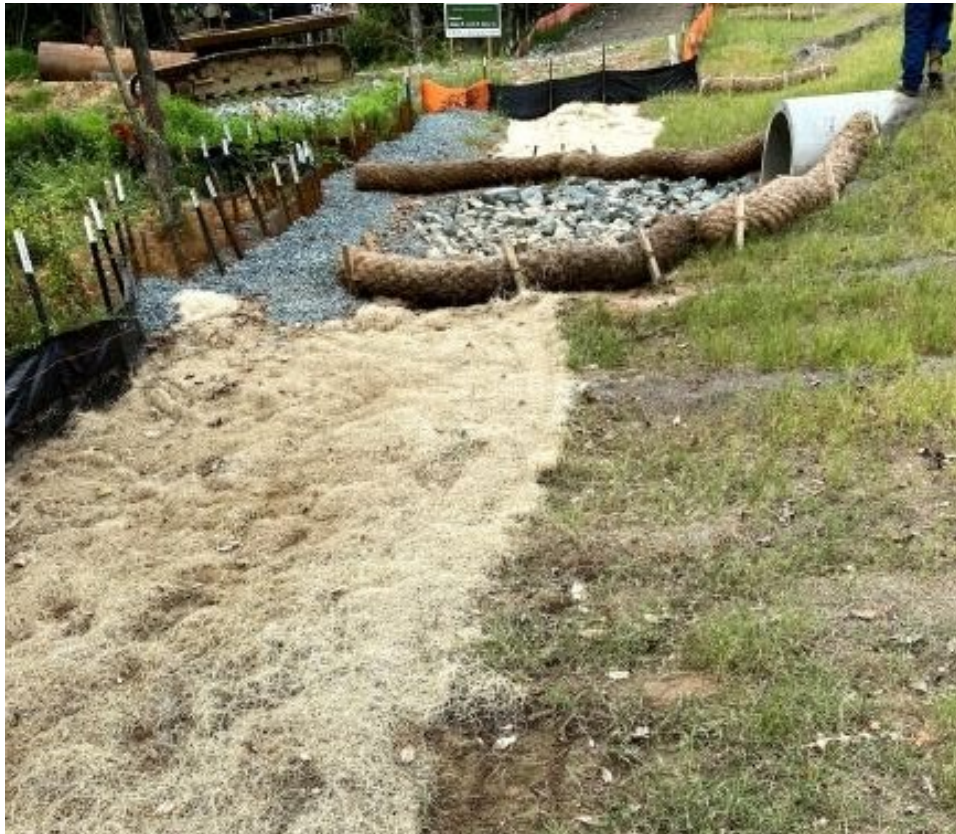
Photo- Storm Drain Outlet (9/17/21)
