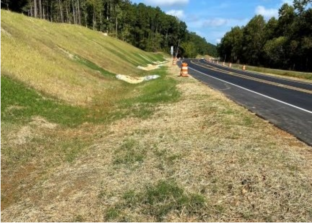
Photo- Vegetation establishing and TRSC-A with PAM installed (10/5/21)
