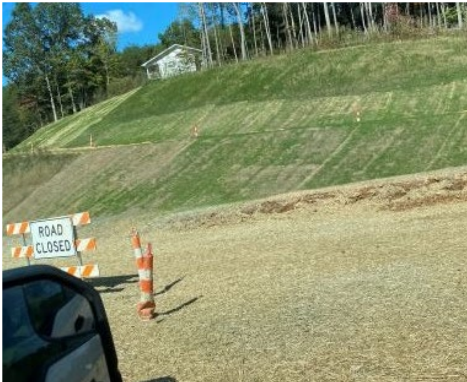
Photo- Completed Slopes stabilized (10/13/21)
