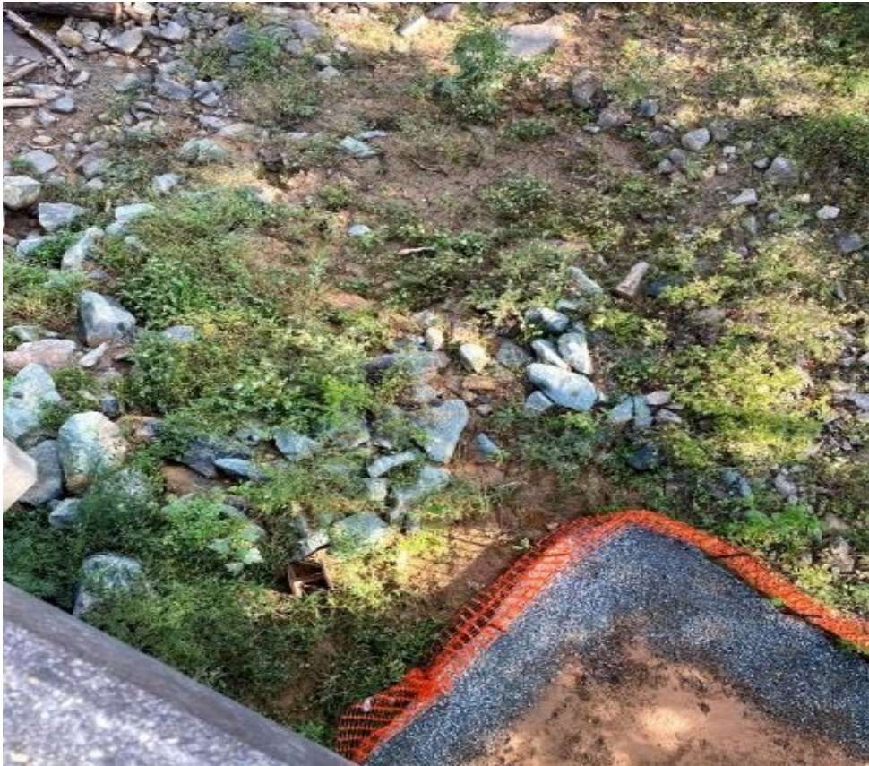
Photo- Evidence of Previous Sediment loss at SSCF (10/5/21)
