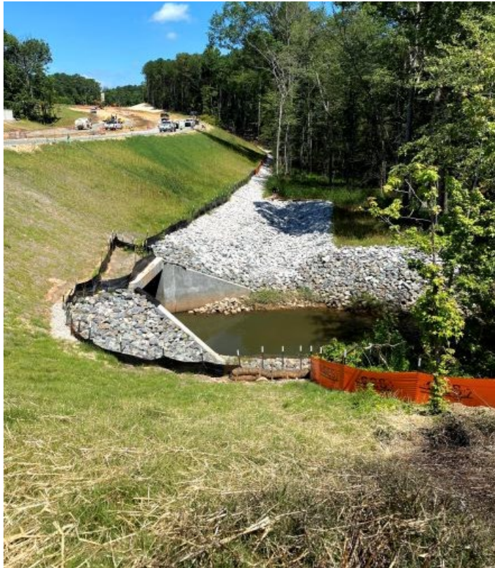
Photo- Culvert installed and area stabilized. (7/14/2021)
