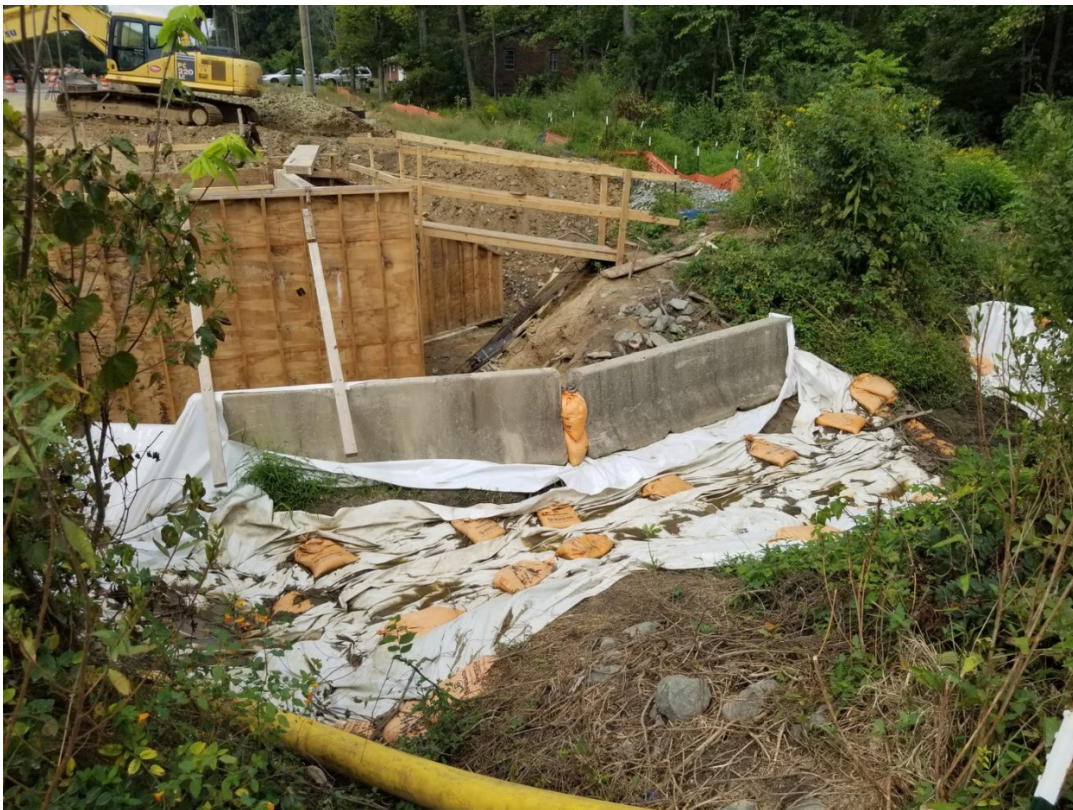
Photo- Lined Stream Diversion and Impervious Dike around Culvert installation (9/17/21)
