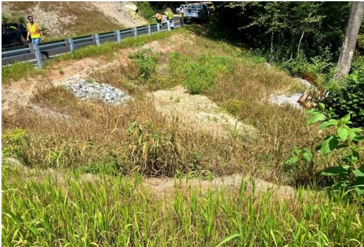
Photo- BR-0124 : Areas being stabilized (8/25/2021) TIP BR-0125 :
