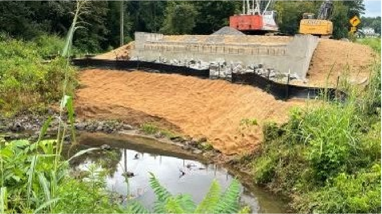
Photo- Bridge #64 over Beaverdam Creek- Finished End Bent stabilized (9/16/2021)
