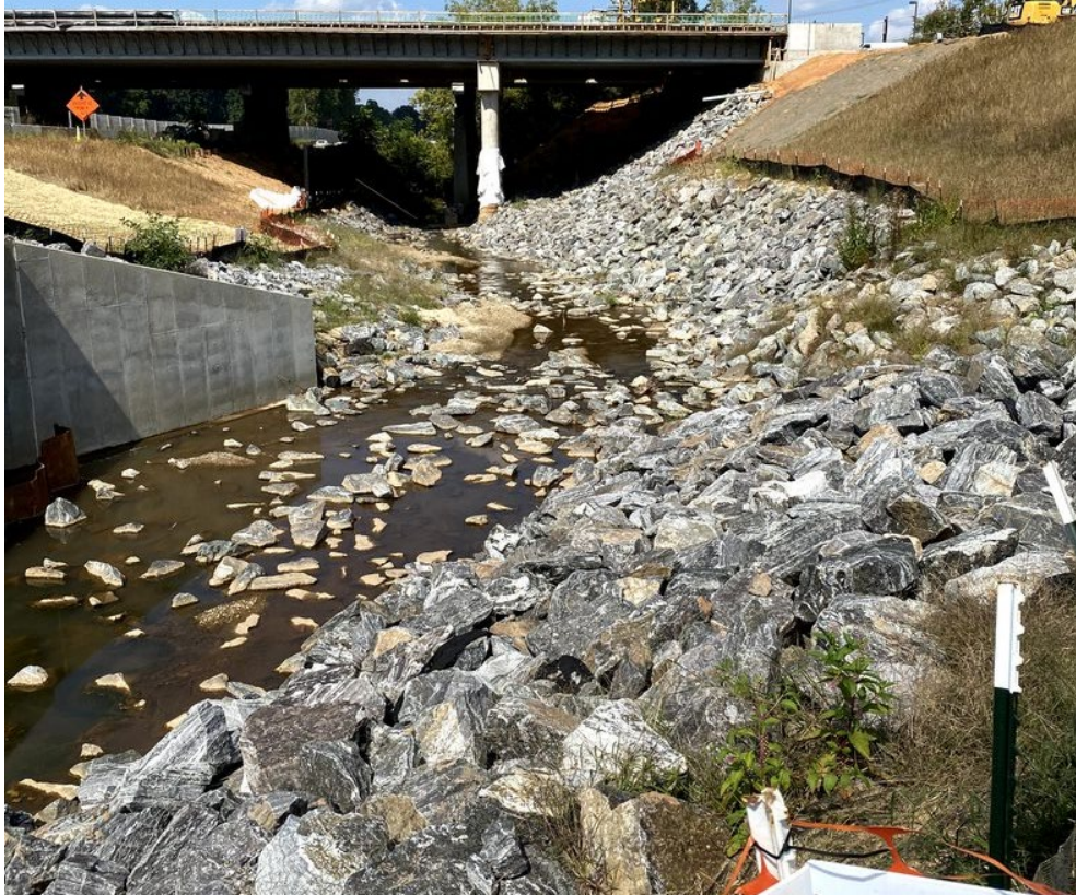
Photo- Culvert extension and Channel Stabilization (9/29/21)
