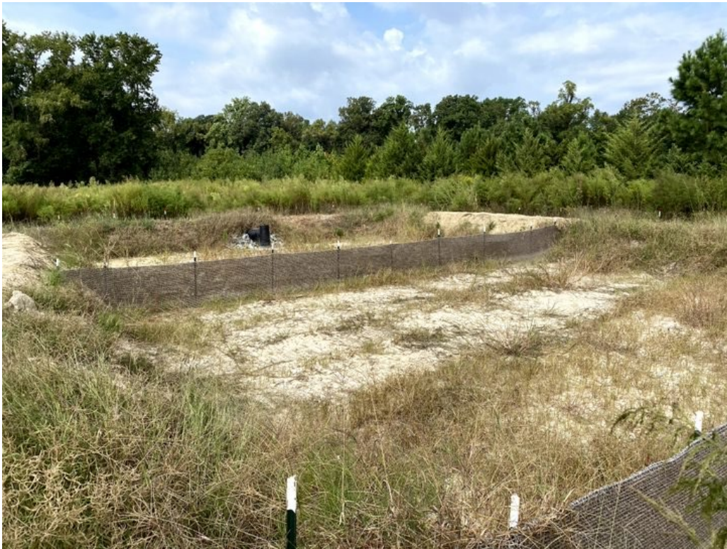
Photo- Stilling basin for Borrow Pit dewatering (9/30/21)
