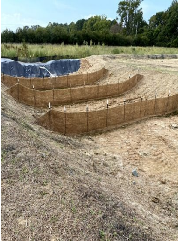
Photo- Skimmer Basins installed in laydown area (9/30/21)
