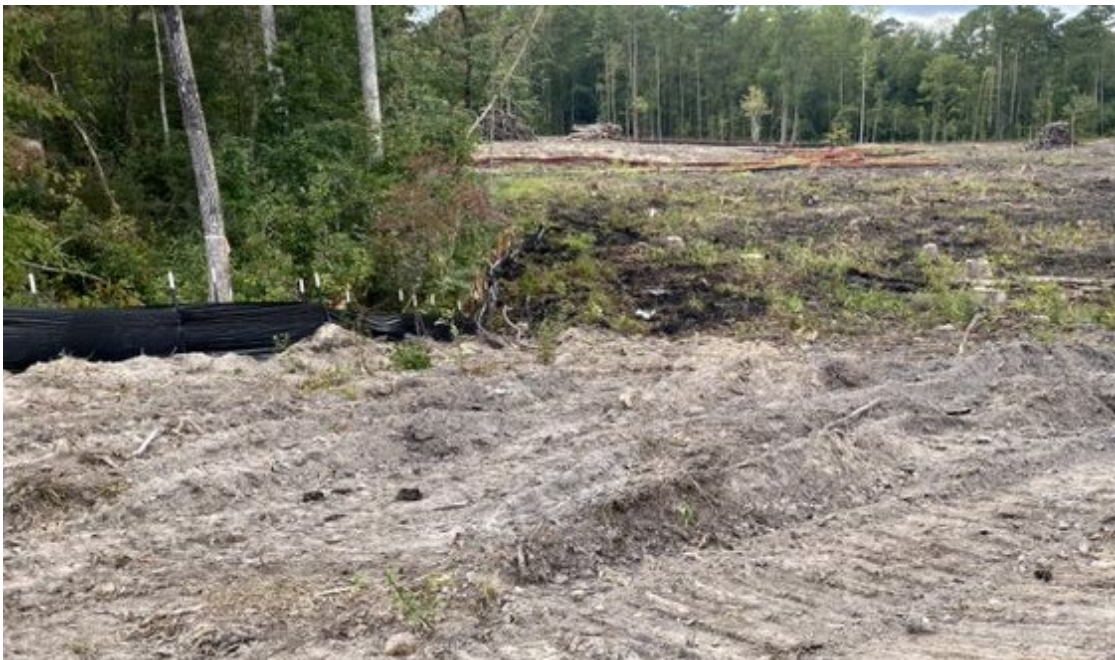
Photo- Active Clearing, ESAs delineated, and Silt fence installed. (10/4/21)
