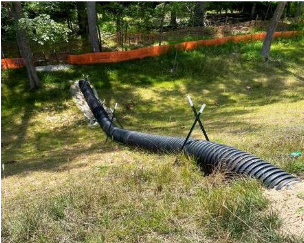
Photo – Well maintained Temporary Slope Drain. (7/14/2021)
