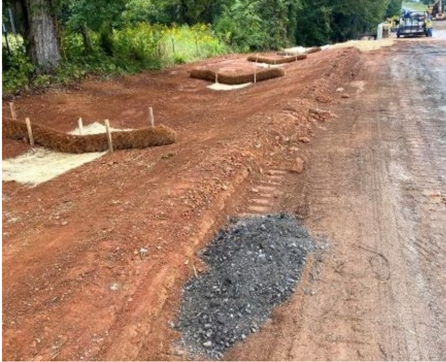
Photo- Bridge #255 over Grant's Creek – Coir Fiber Wattles with PAM (9/16/2021)
