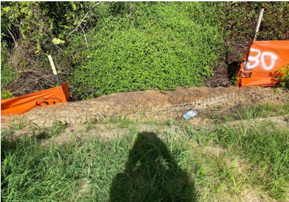
Photo- Silt fence and wattle breaks installed and maintained (8/31/21)
