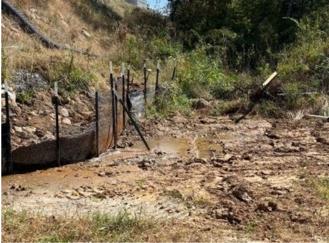
Photo- Sediment deposited beyond SSCF (10/14/21)
