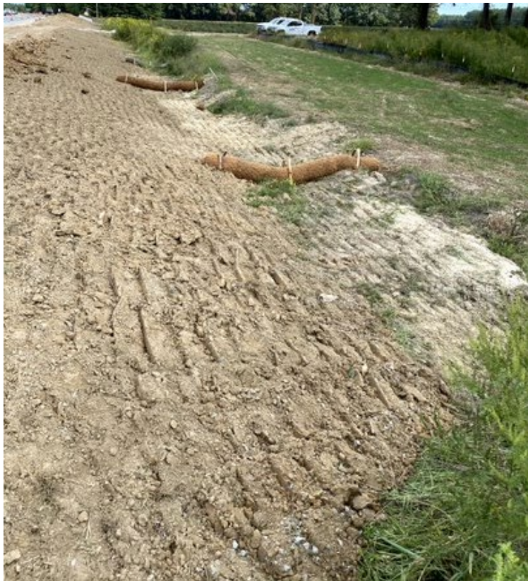
Photo- Recently graded ditch with Wattles (9/30/21)
