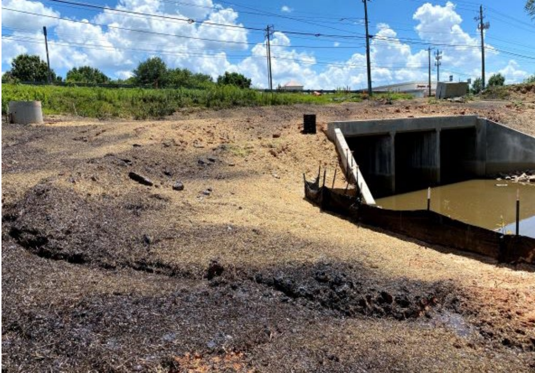
Photo- Culvert installed (7/14/2021)
