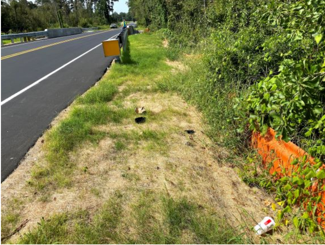
Photo – Final vegetation being established (8/31/21)
