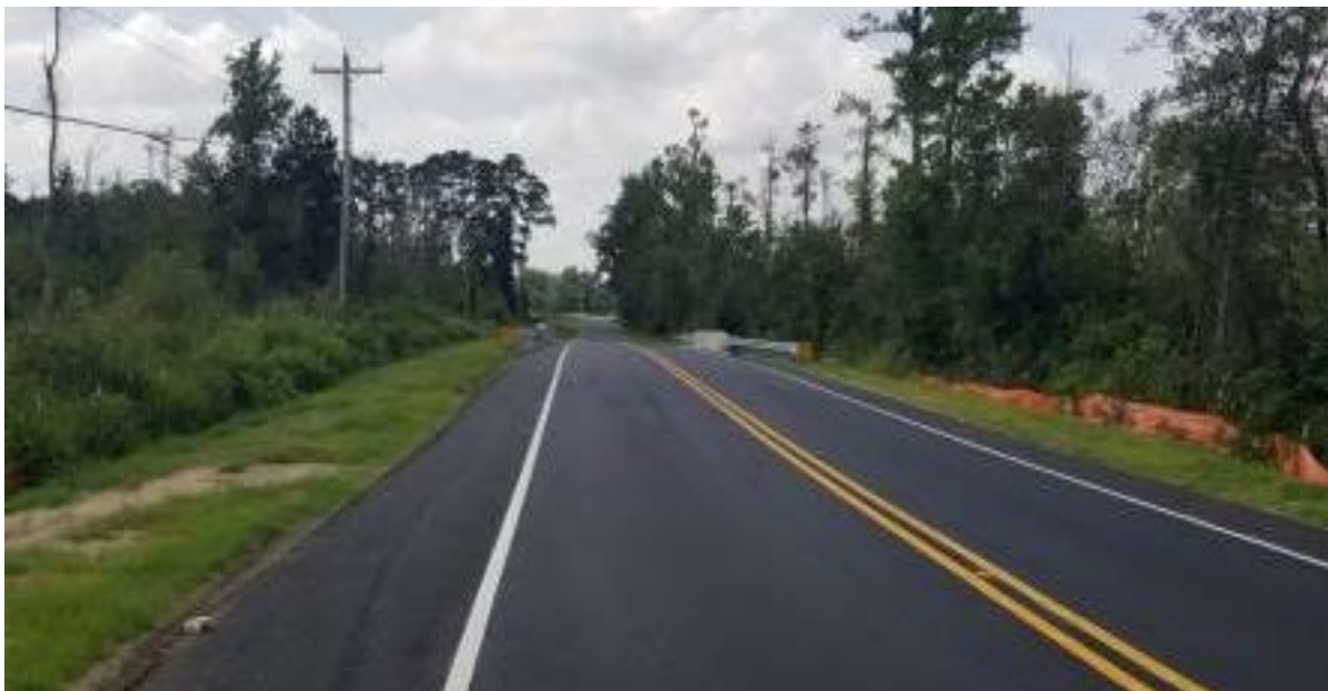
Photo -Bridge construction completed (8/31/21)
