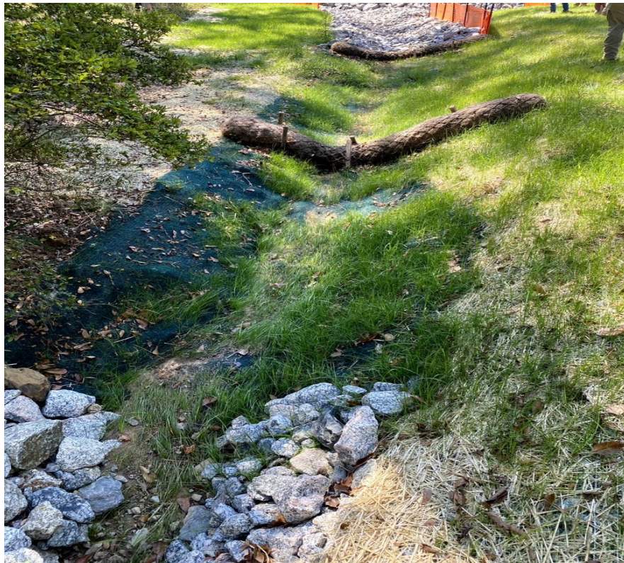
Photo- Wattles and vegetation establishing (9/28/2021)
