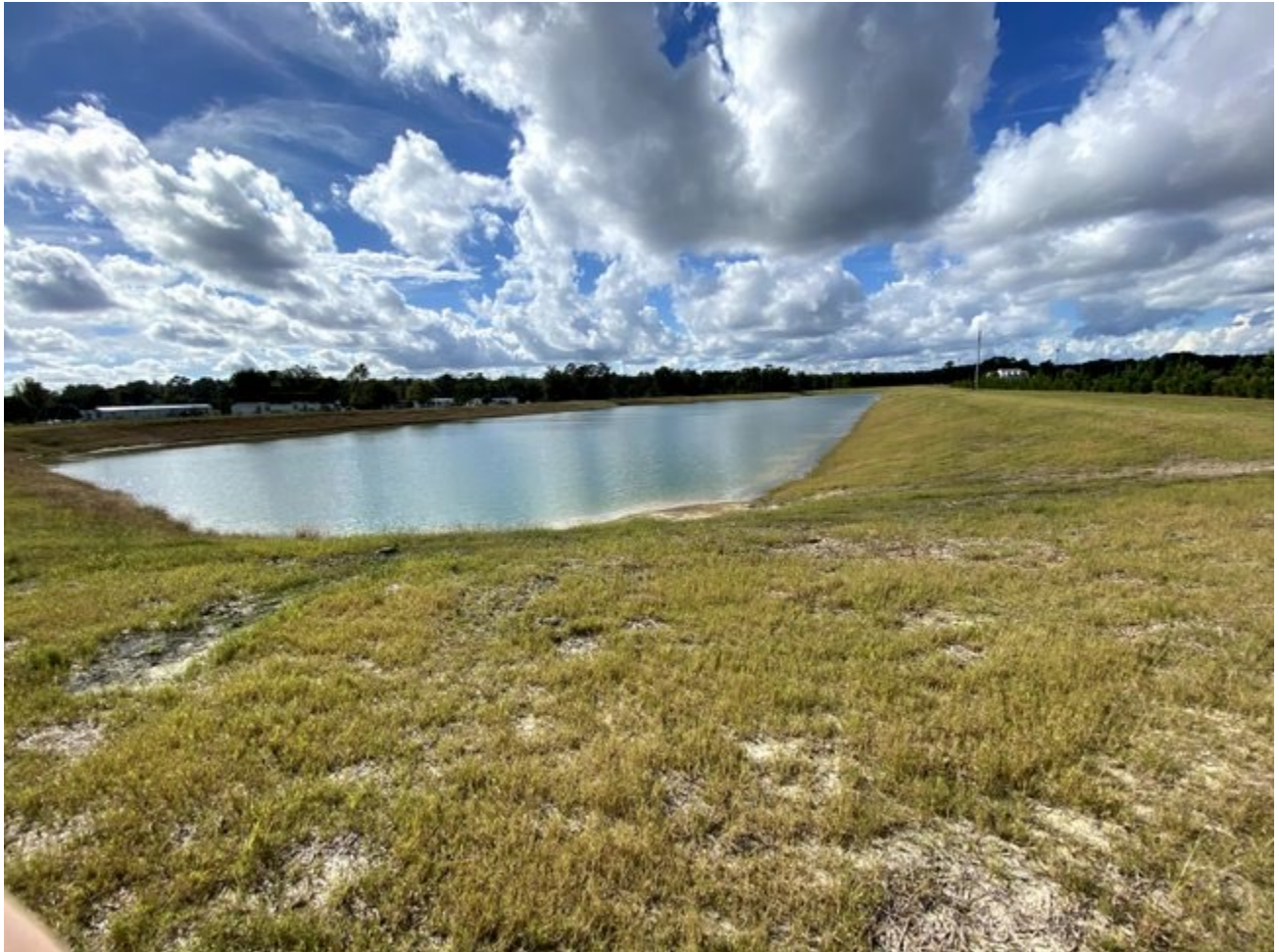
Photo- Completed Borrow Pit (10/4/21)
