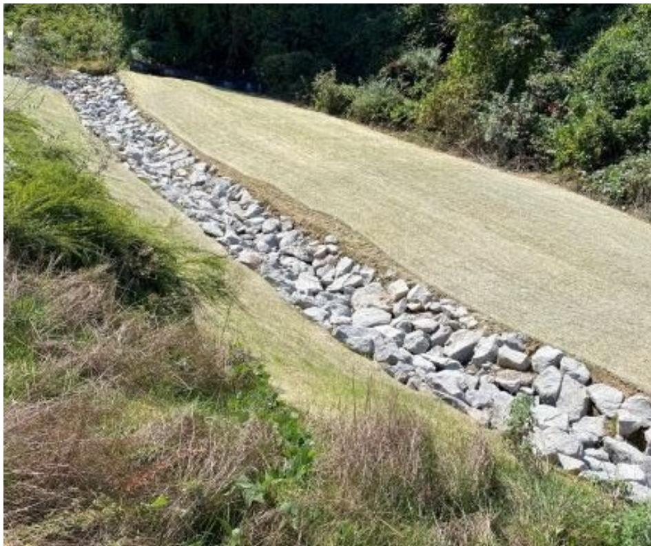
Photo- Basin removed and Permanent Ditch recently completed (10/13/21)
