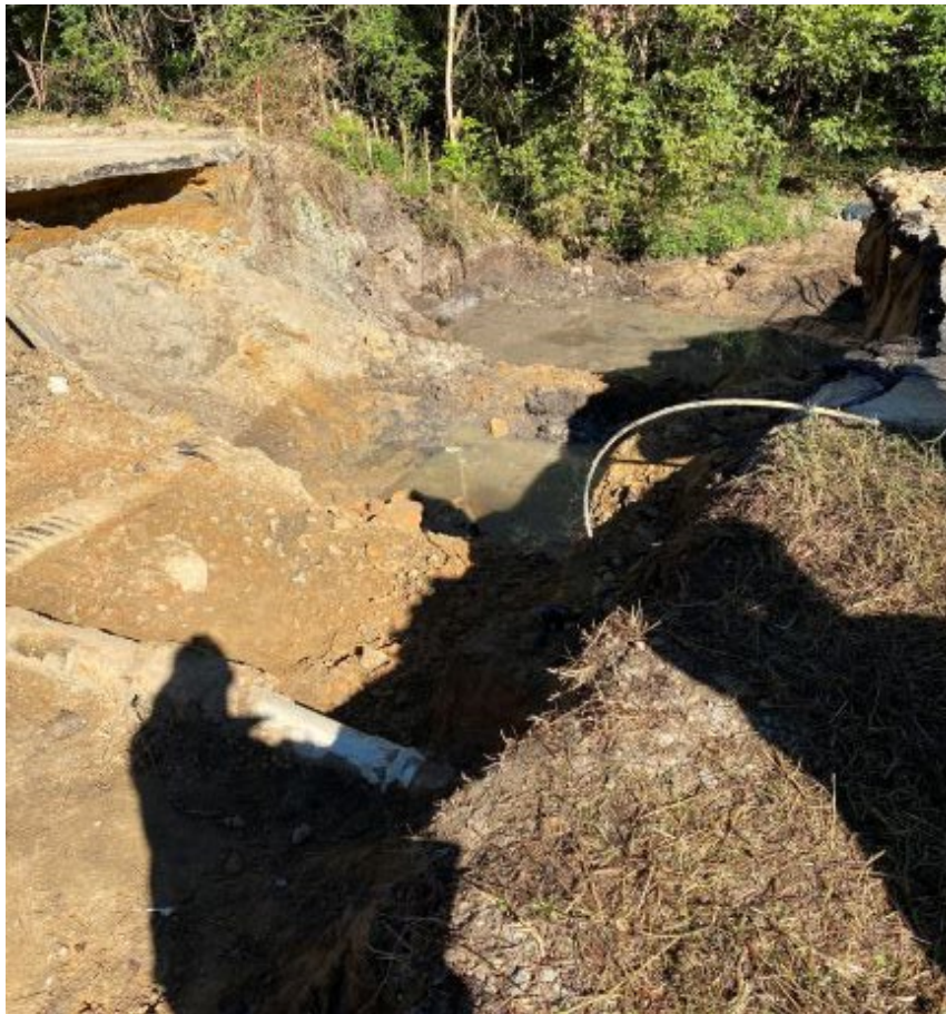
Photo- Existing pipe has been excavated (10/19/2021)
