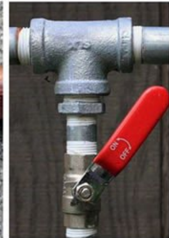
Galvanized Steel & valve
