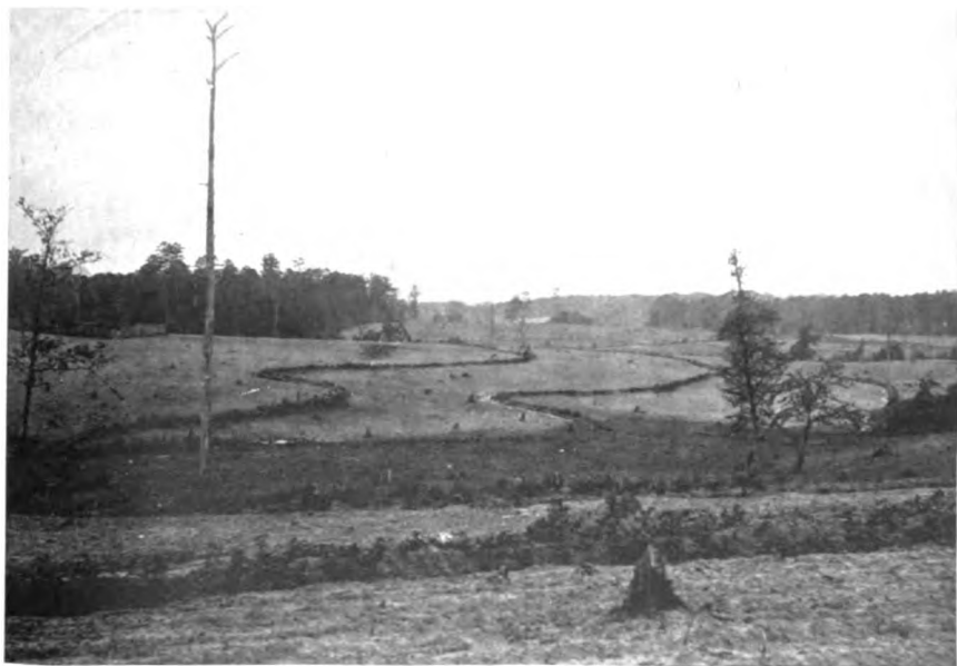
B. INCOMPLETE TERRACES WELL LOCATED BUT TOO FAR APART, THE RISE BETWEEN THEM BEING TOO GREAT. AT LEAST ONE INTERVENING TERRACE SHOULD HAVE BEEN CONSTRUCTED.
