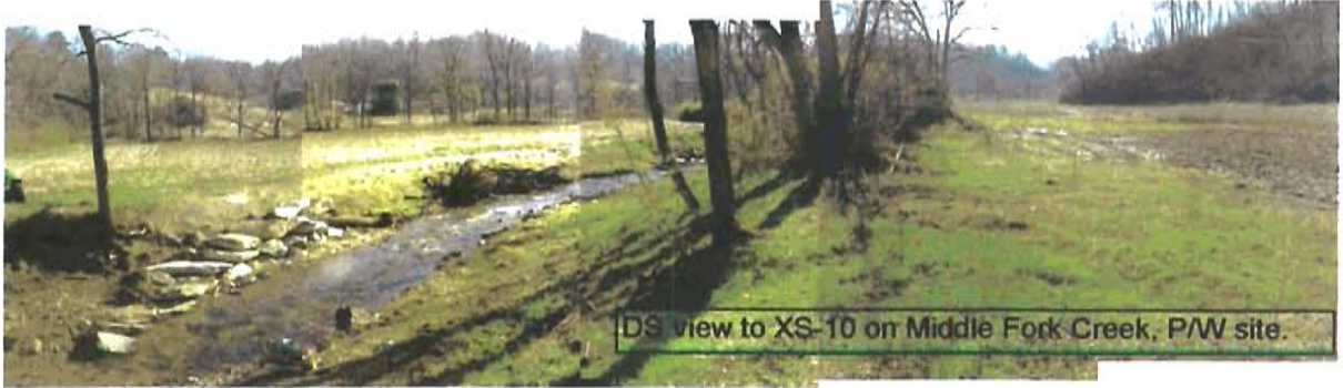
US view to XS-10 on Middle Fork Creek, P/W site.
