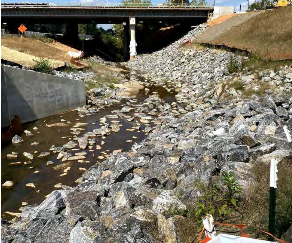
Photo- Culvert extension and Channel Stabilization (9/29/21)
