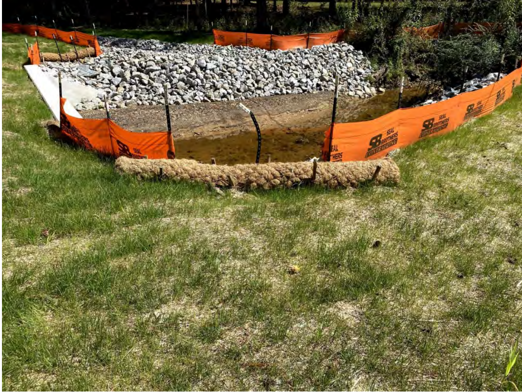
Photo- Riprap armoring and silt fence maintained (9/28/2021)
