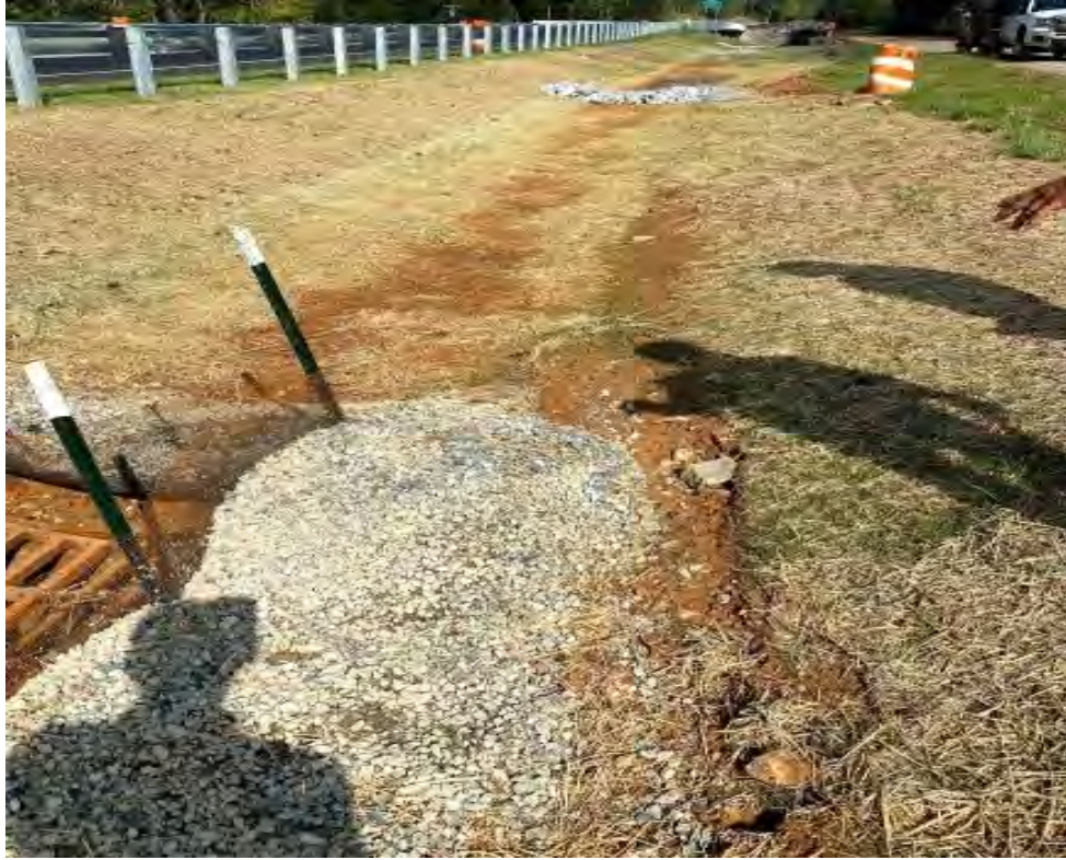
Photo- Ditch line measures installed (10/5/21)
