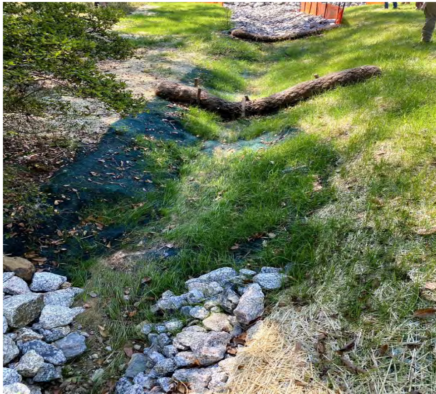
Photo- Wattles and vegetation establishing (9/28/2021)
