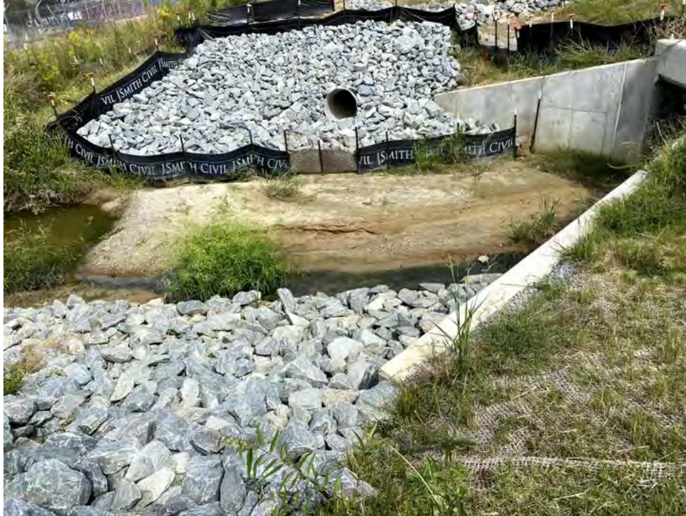
Photo- Culvert completed, surrounding areas stabilized (9/30/21)
