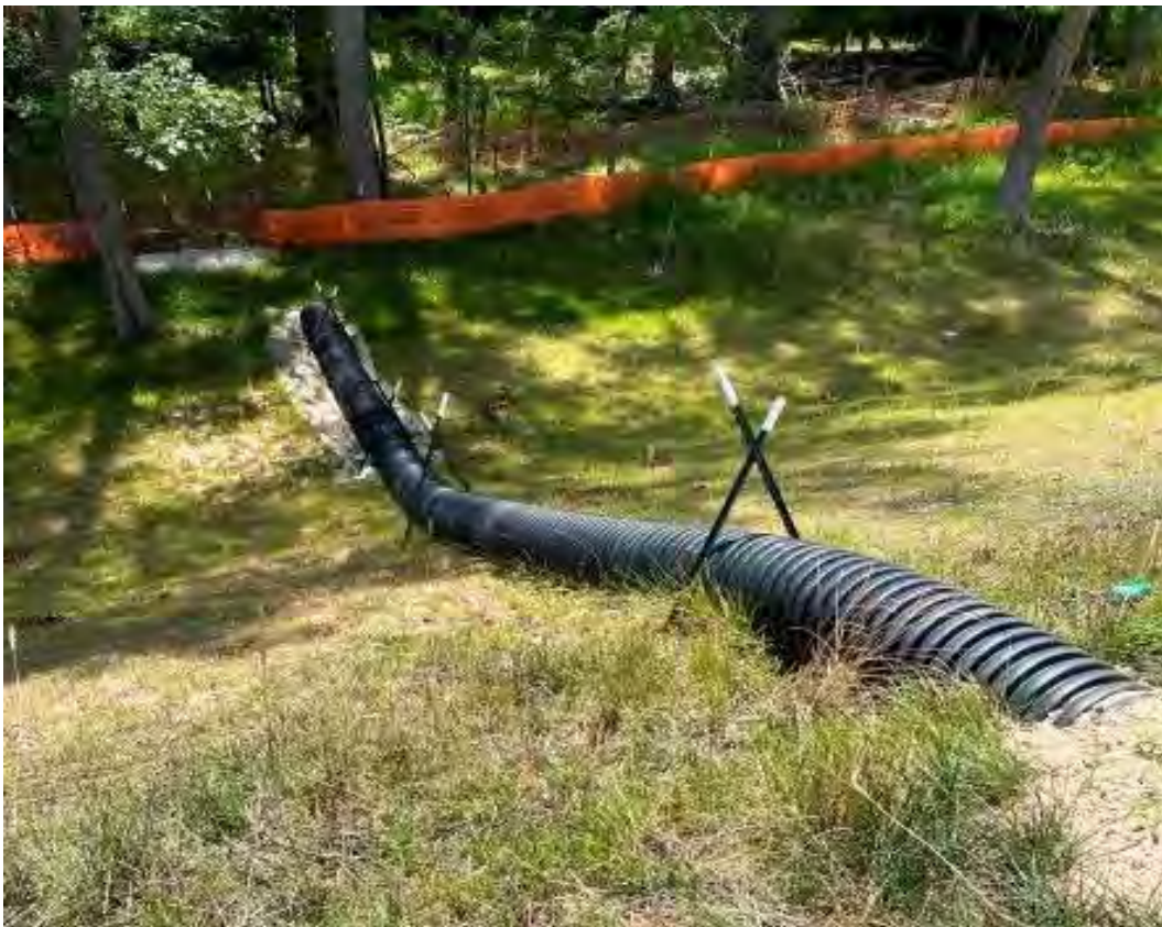
Photo – Well maintained Temporary Slope Drain. (7/14/2021)
