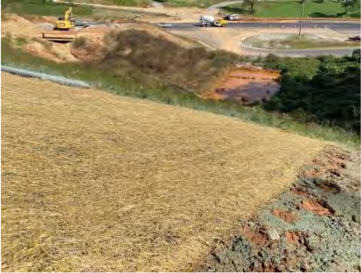
Photo- Waste Area Skimmer Basin and Entrance (10/13/21)
