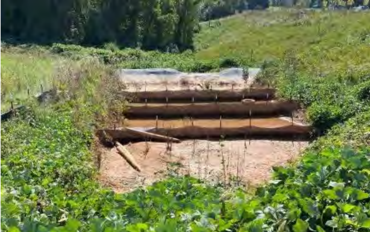
Photo- Wood pole laying across Baffle (10/13/21)
