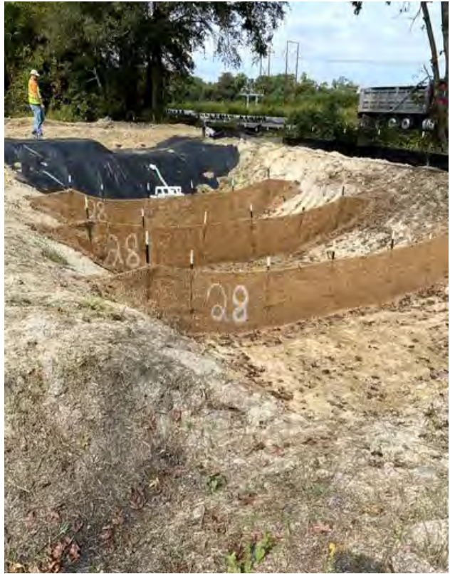
Photo- Skimmer Basins installed in laydown area (9/30/21)
