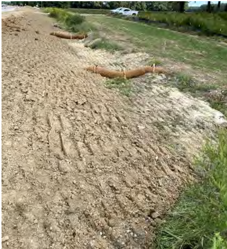
Photo- Recently graded ditch with Wattles (9/30/21)
