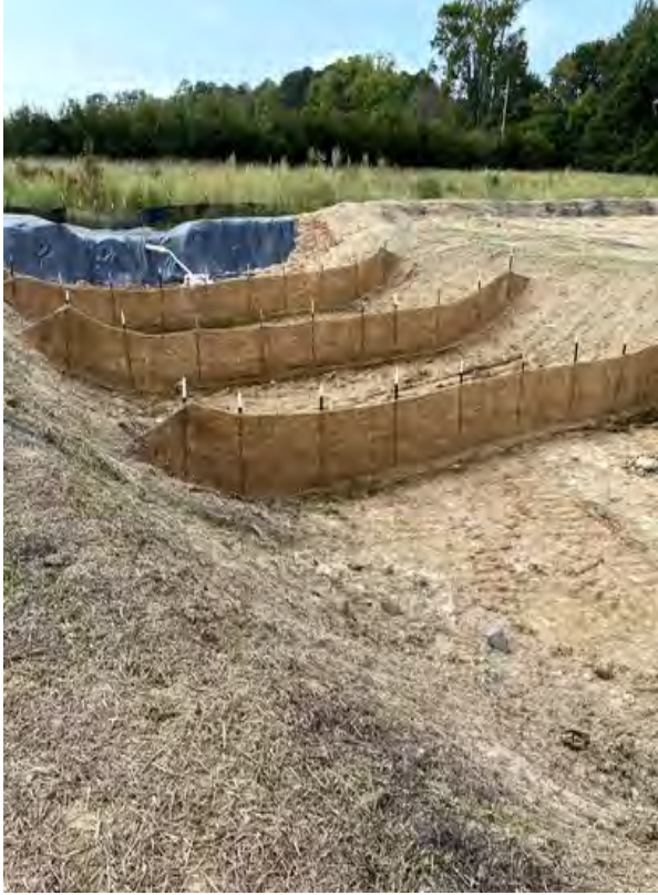
Photo- Skimmer Basins installed in laydown area (9/30/21)
