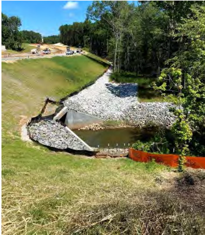
Photo- Culvert installed and area stabilized. (7/14/2021)
