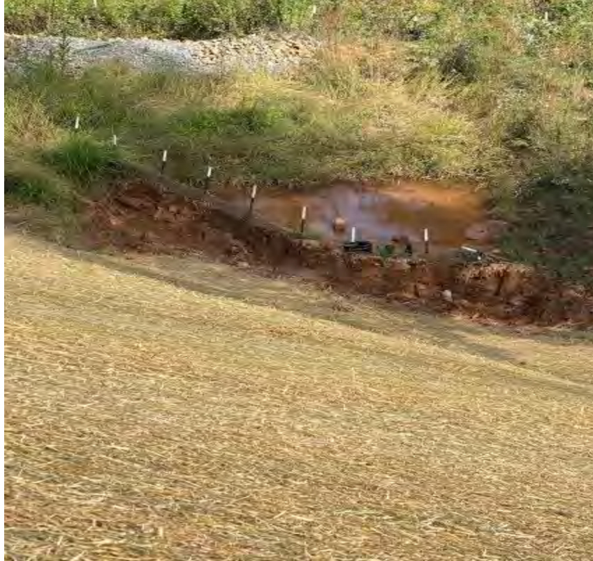
Photo- TRSD-B partially removed for slope grading (10/13/21)
