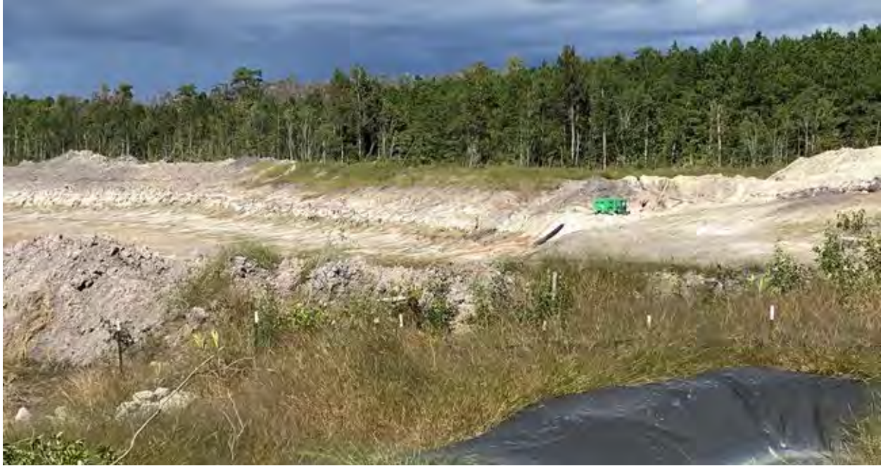
Photo- Active Borrow Pit pumping to Stilling Basin (10/4/21)
