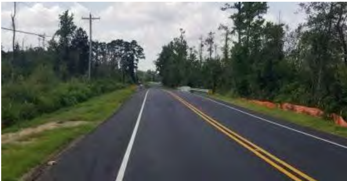
Photo -Bridge construction completed (8/31/21)
