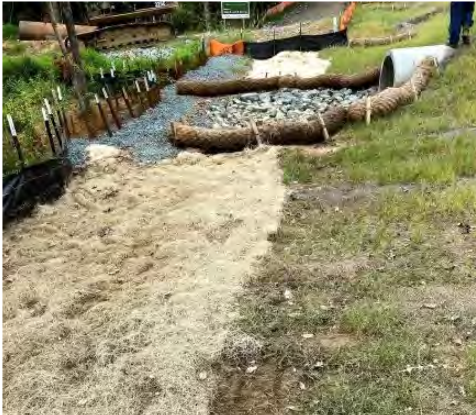
Photo- Storm Drain Outlet (9/17/21)
