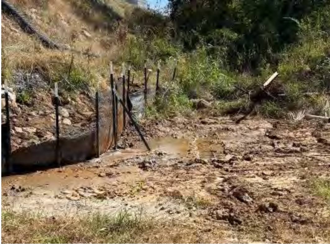
Photo- Sediment deposited beyond SSCF (10/14/21)
