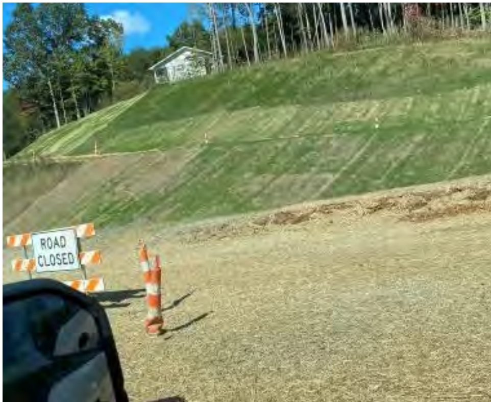
Photo- Completed Slopes stabilized (10/13/21)
