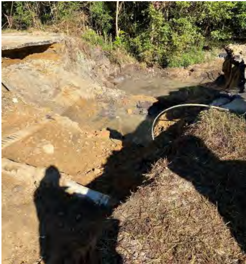
Photo- Existing pipe has been excavated (10/19/2021)
