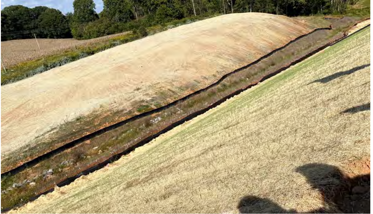
Photo- Channel change and slopes stabilized (9/29/21)
