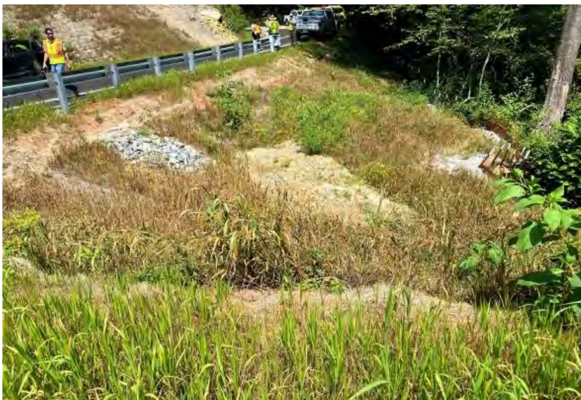
Photo- BR-0124 : Areas being stabilized (8/25/2021) TIP BR-0125 :
