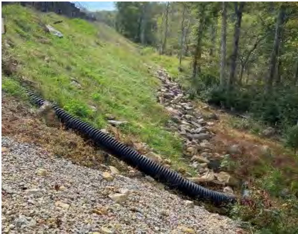
Photo- Slopes Stabilized (10/12/21)
