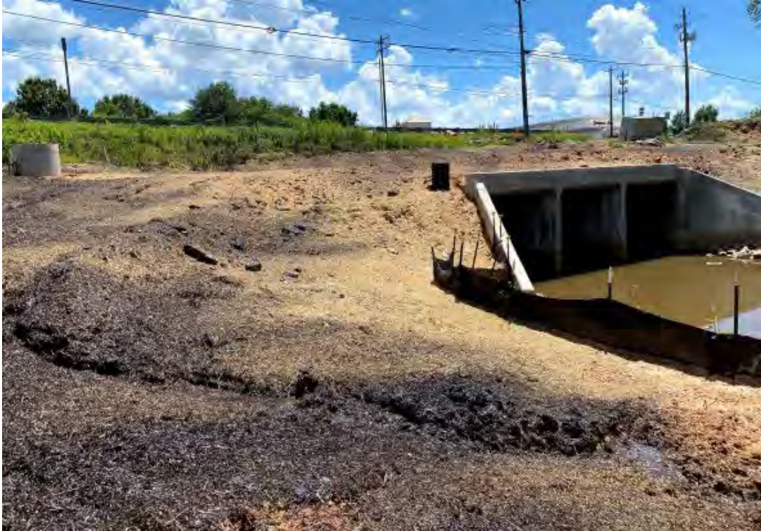
Photo- Culvert installed (7/14/2021)
