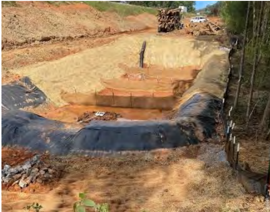
Photo-Recently Installed Basin (10/14/21)
