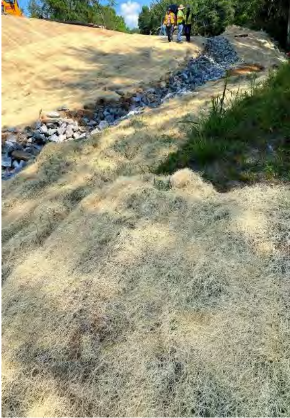
Photo- BR-0125 : Permanent Ditch (left) and Stream Relocation (Right) (8/25/2021)
