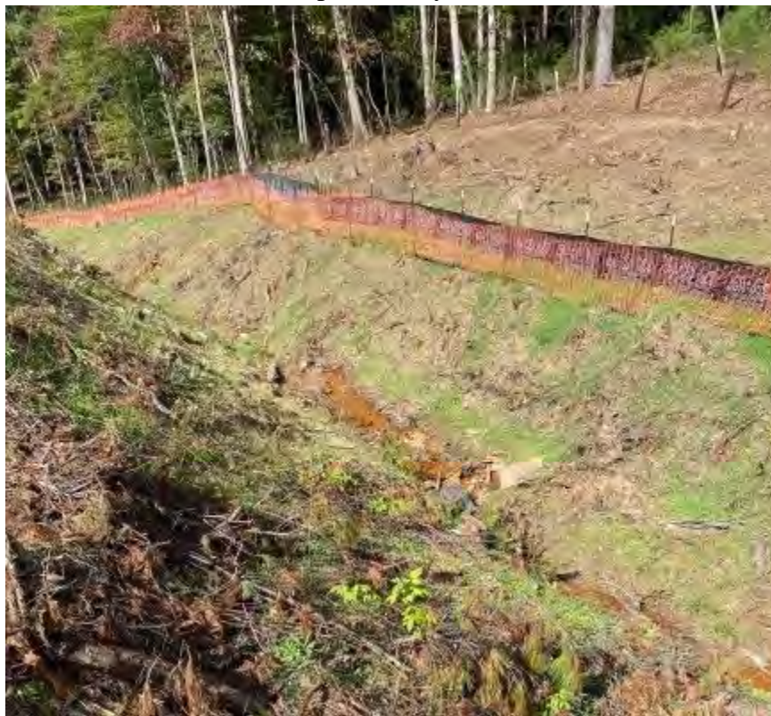
Photo- Cleared ESA (10/14/21)
