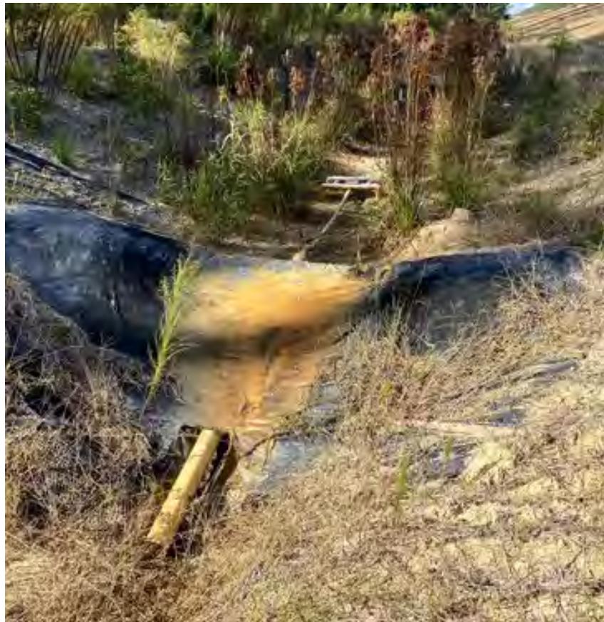
Photo- Earthen Dam with Skimmer (10/4/21)
