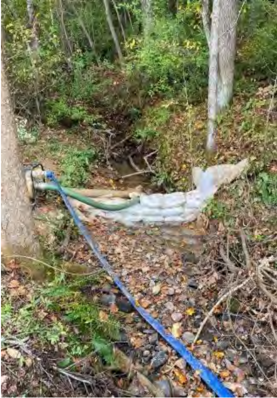
Photo- Impervious dike and pump around for culvert extension (10/14/21)
