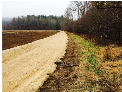
Grassed waterway installation
