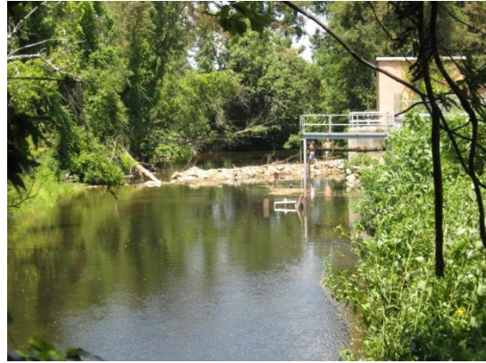
Hendersonville Water Intake Structure
