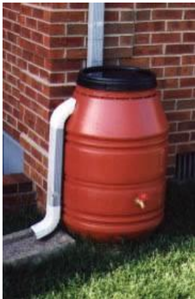
A rain barrel is attached to a downspout and collects rain water.
