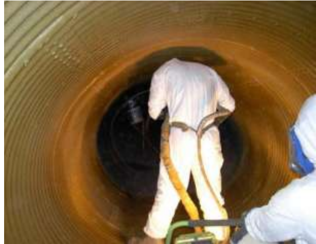
Figure 2-10. Spray-Applied Polyurethane in a Man-Entry Size Pipe
