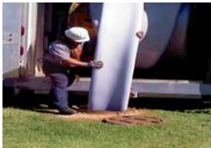
Figure 2-6. PVC FnF Material Heated and Being Pulled into Position
