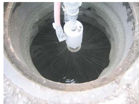
Figure 6-3. Spin-Cast Application of a Fiber-Reinforced Cementitious Structural Liner (Courtesy AP/M Permacast)
