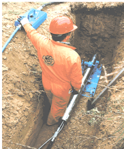
Figure 4-21. Impact-Moling Process (Courtesy TT Technologies)
