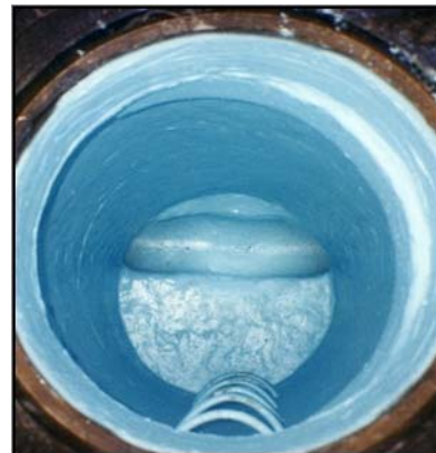
Figure 6-4. Rehabilitated Manhole Using a Spray-Applied Epoxy Liner (Courtesy RLS Solutions)
