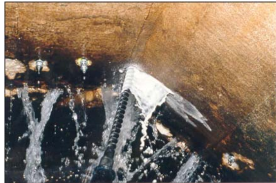
Figure 6-1. Grouting of Active Leaks (Courtesy Prime Resins)
