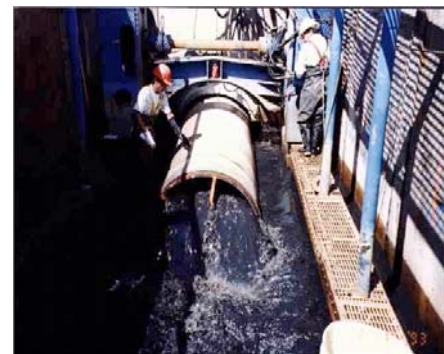
Figure 4-18. Live Insertion Sliplining (Courtesy Hobas Pipe USA)
