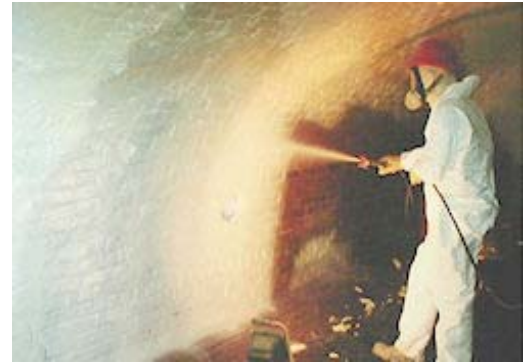
Figure 4-15. Spray-Applied Epoxy Lining in a Brick Sewer Tunnel (Courtesy Warren Environmental)
