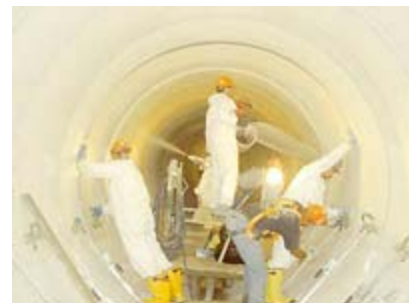
Figure 4-13. Linabond Panel Lining Installation (Courtesy Linabond)
