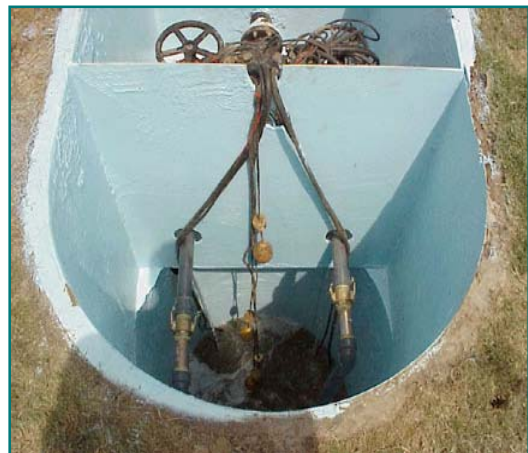
Figure 7-1. Spray Epoxy Rehabilitation of a Lift Station (Courtesy RLS Solutions)
