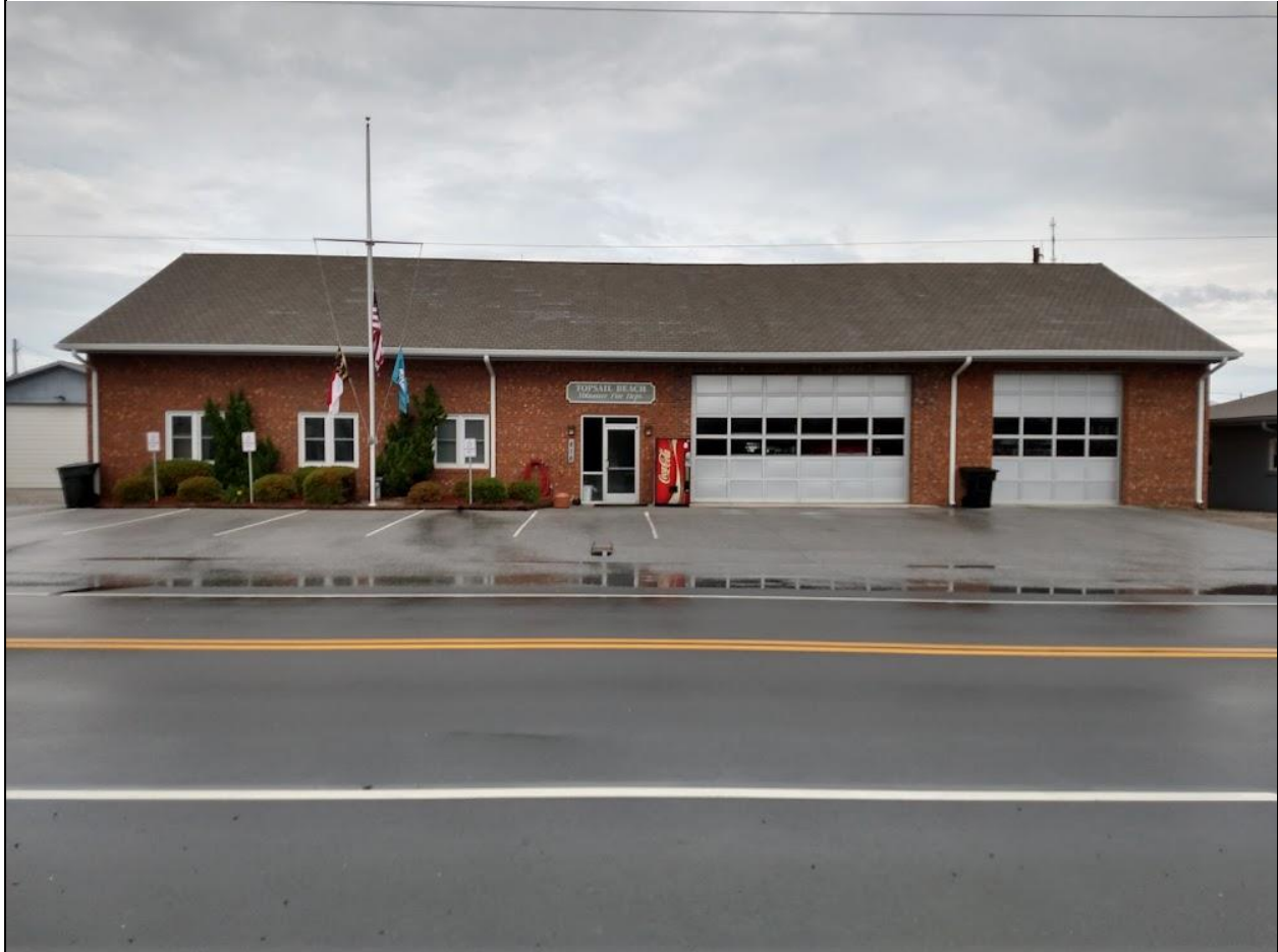
FIGURE B.1 – TOPSAIL BEACH FIRE STATION, FFE 4.71 NAVD88 (SOURCE: https://www.helpmecovid.com/us/6958525_topsail-beach-fire-department )
