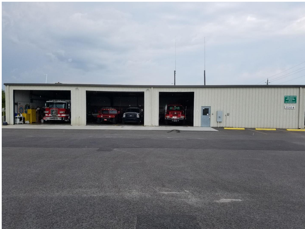
FIGURE B.5 – NORTH TOPSAIL BEACH – SOUTH END FIRE STATION, FFE 8.35 NAVD88 (SOURCE: https://www.onslowcountync.gov/1080/Fire-Rescue-Agencies )
