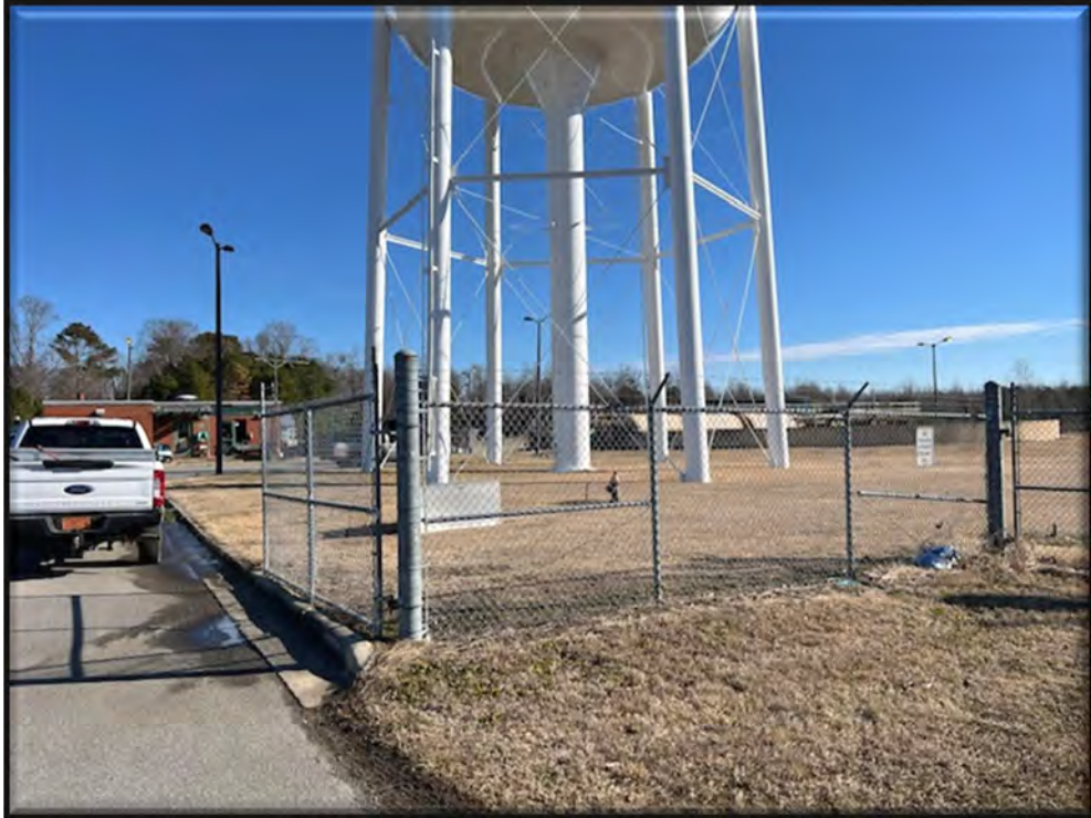
Photo 1: View of WWTP, facing northeast.
