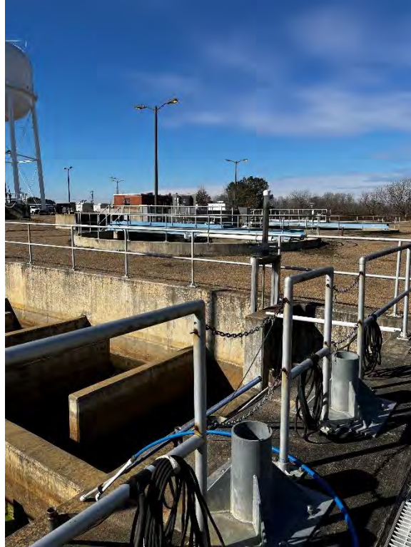
Permanently Open Slide Gate
