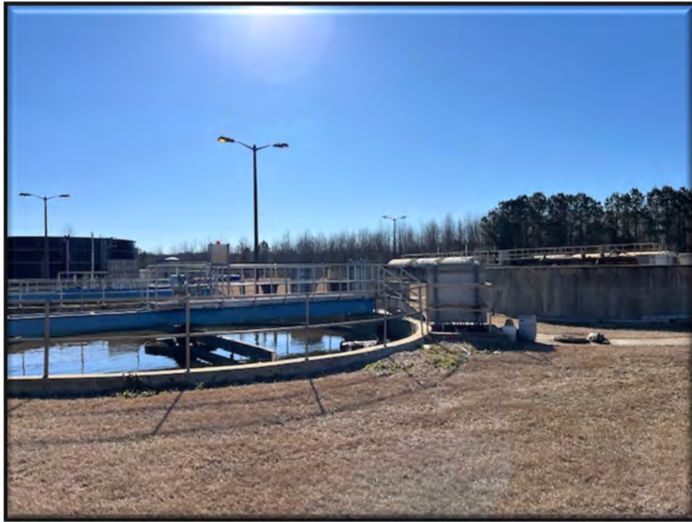
Photo 5: View of WWTP, facing east.
