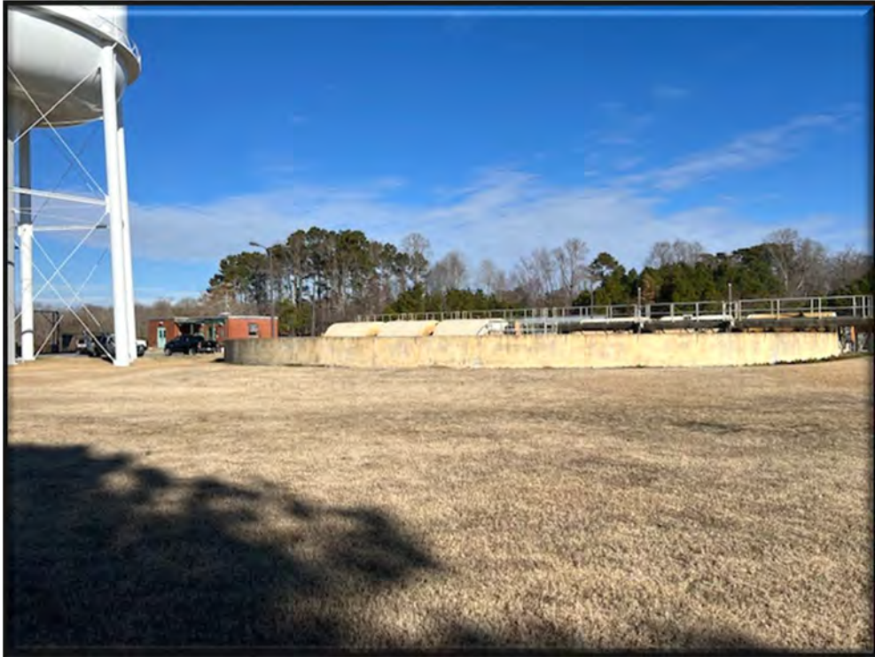
Photo 3: View of WWTP, facing north.
