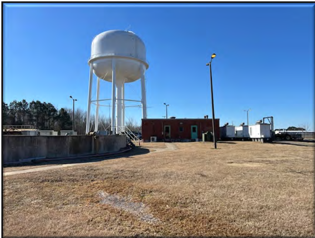
Photo 5: View of WWTP, facing south.
