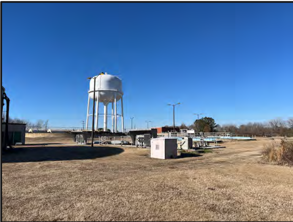
Photo 4: View of WWTP, facing south.
