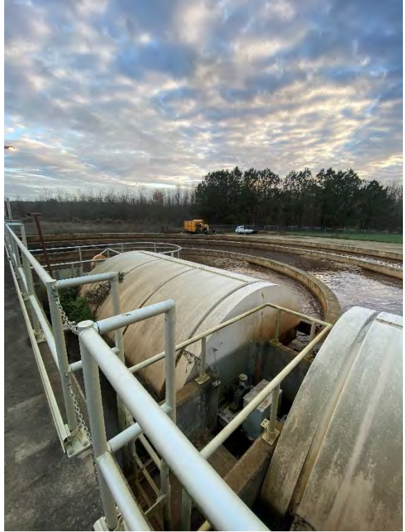
Oxidation Ditch Aerators
