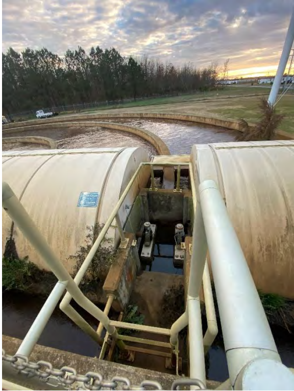
Oxidation Ditch Aerators
