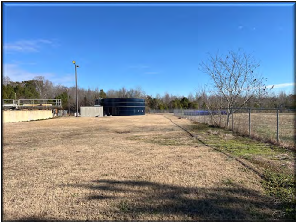
Photo 2: View of WWTP, facing east.
