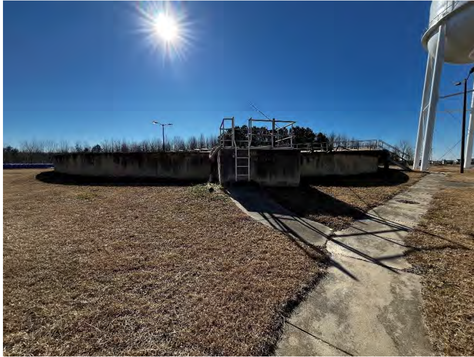
Sludge Holding Tank
