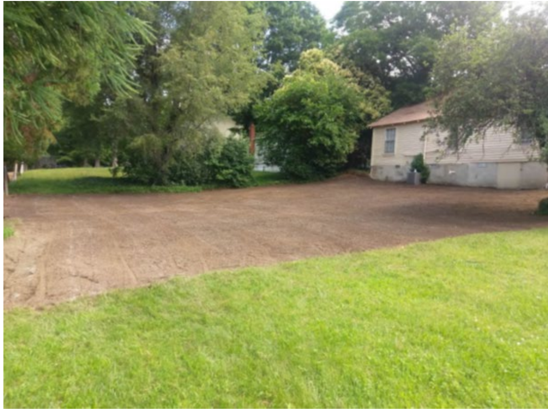
1-2 feet of certified clean topsoil added
