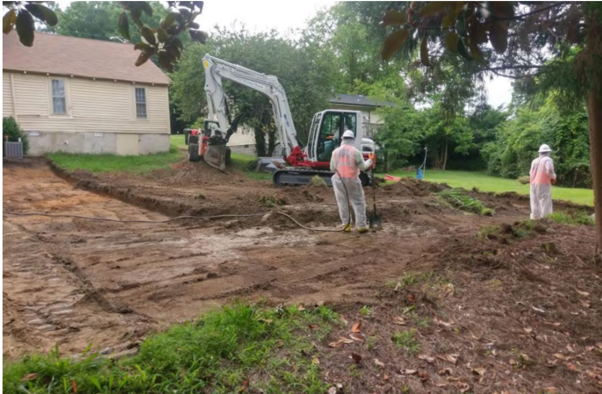
Removal of 1-2 feet of asbestos containing soil
