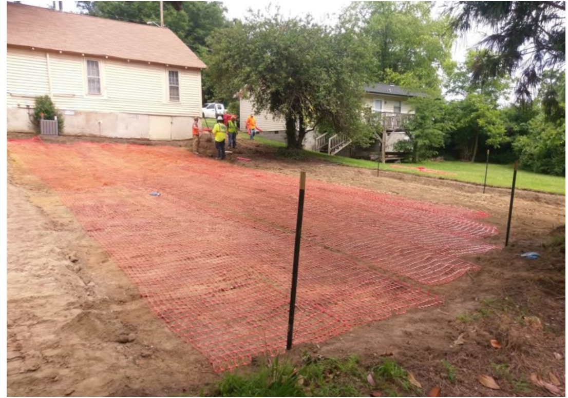
Visual barrier with fence material
