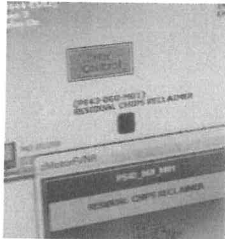
Figure 4-3. Mix Control Program Indicator in Control Room
