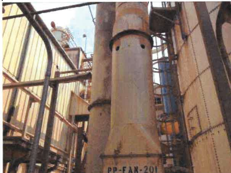
Figure 4-6. Photograph of the Dry Hammermill 2 Sampling Location
