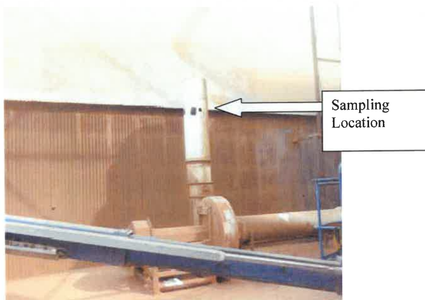
Figure 4-8. Green Hammermill Stack
