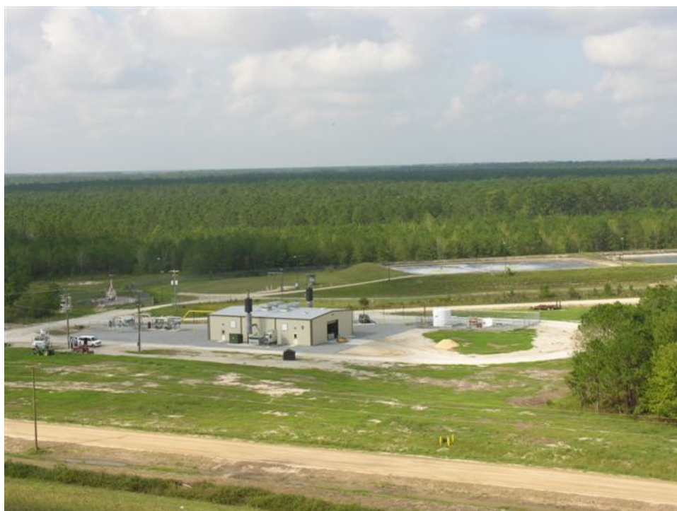
The generator as viewed from the top of the closed CRSWMA landfill cell. The leachate pre-treatment ponds and the flare station are in the background.
