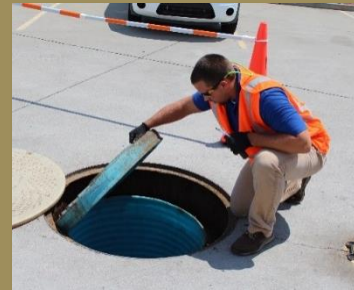
Inspecting a containment sump
